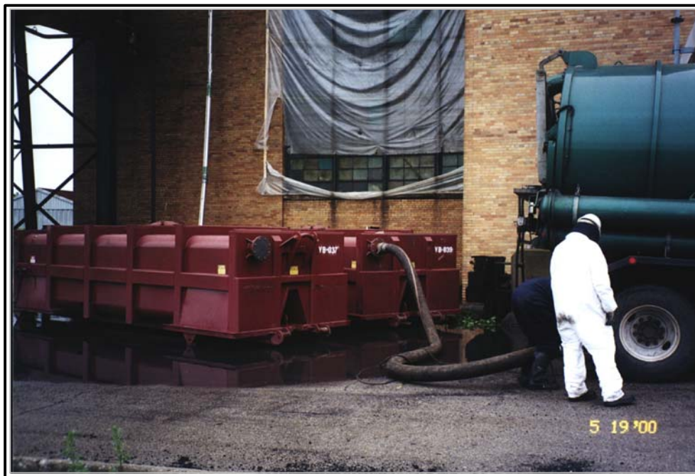
PHOTO #8 INLAND WATER REMOVING FLY ASH FROM THE POWERHOUSE.
