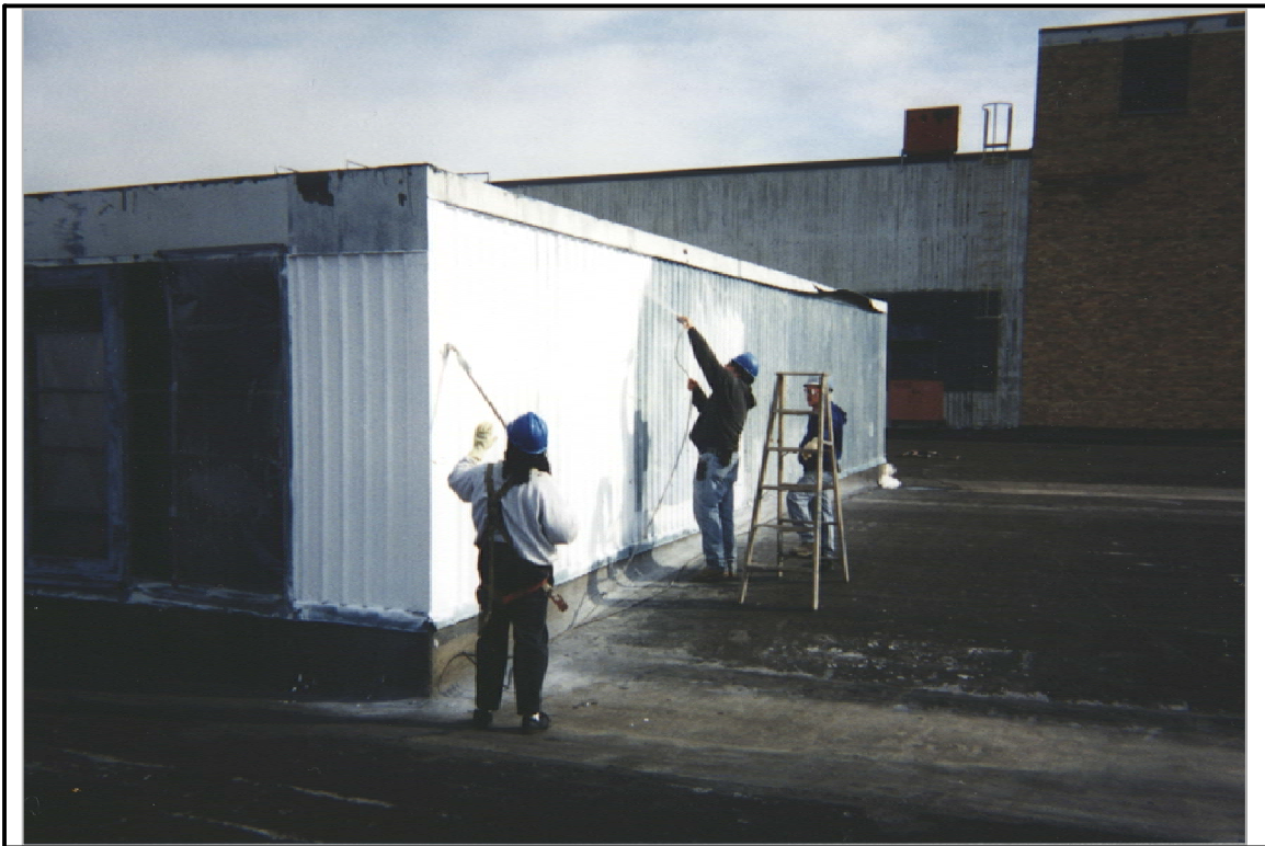
PHOTO #1 GALBESTOS ENCAPSULATION
