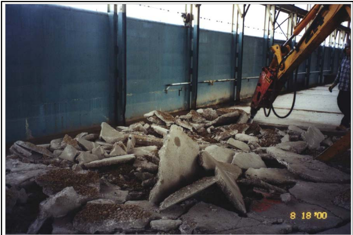
PHOTO #10 OPENING CONCRETE BINS IN BUILDING 63.
