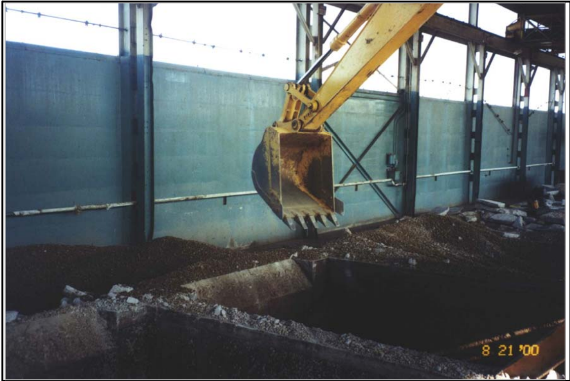
PHOTO #11 REMOVING MATERIAL FROM BINS IN BUILDING 63.
