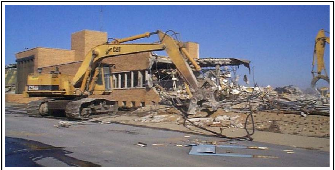
PHOTO 6: ADMINISTRATION BUILDING DEMOLITION
