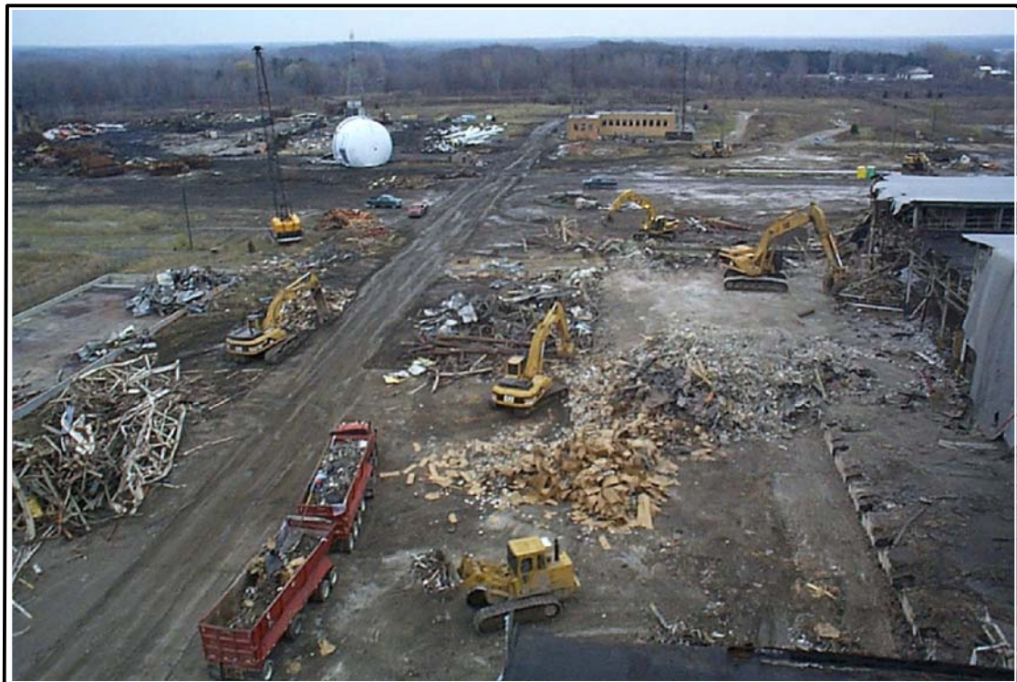
PHOTO 4: SORTING DEMOLITION DEBRIS
