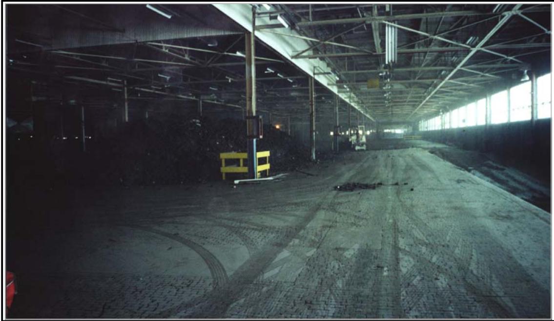
PHOTO #7 STAGED WOOD BLOCK FLOORING.
