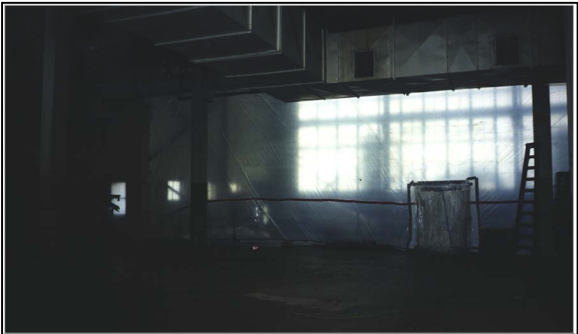
PHOTO #4 ENCAPSULATION THE POWERHOUSE PRIOR TO ASBESTOS REMOVAL.
