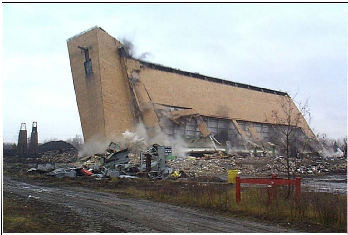
PHOTO 2: SOUTH WALL POWERHOUSE DEMOLITION
