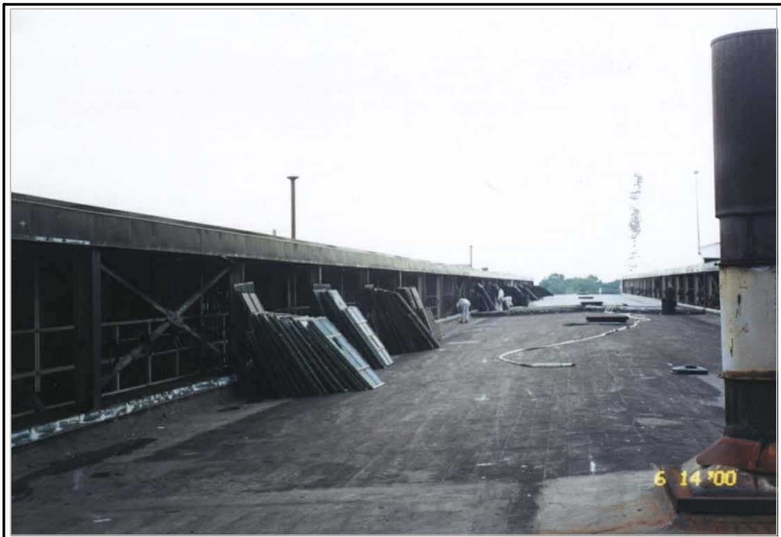
PHOTO #12 WINDOW PANE REMOVAL FROM BUILDING 44.
