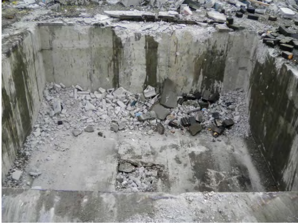
Photo 2: Former freight elevator pit (AOI 30.2)
