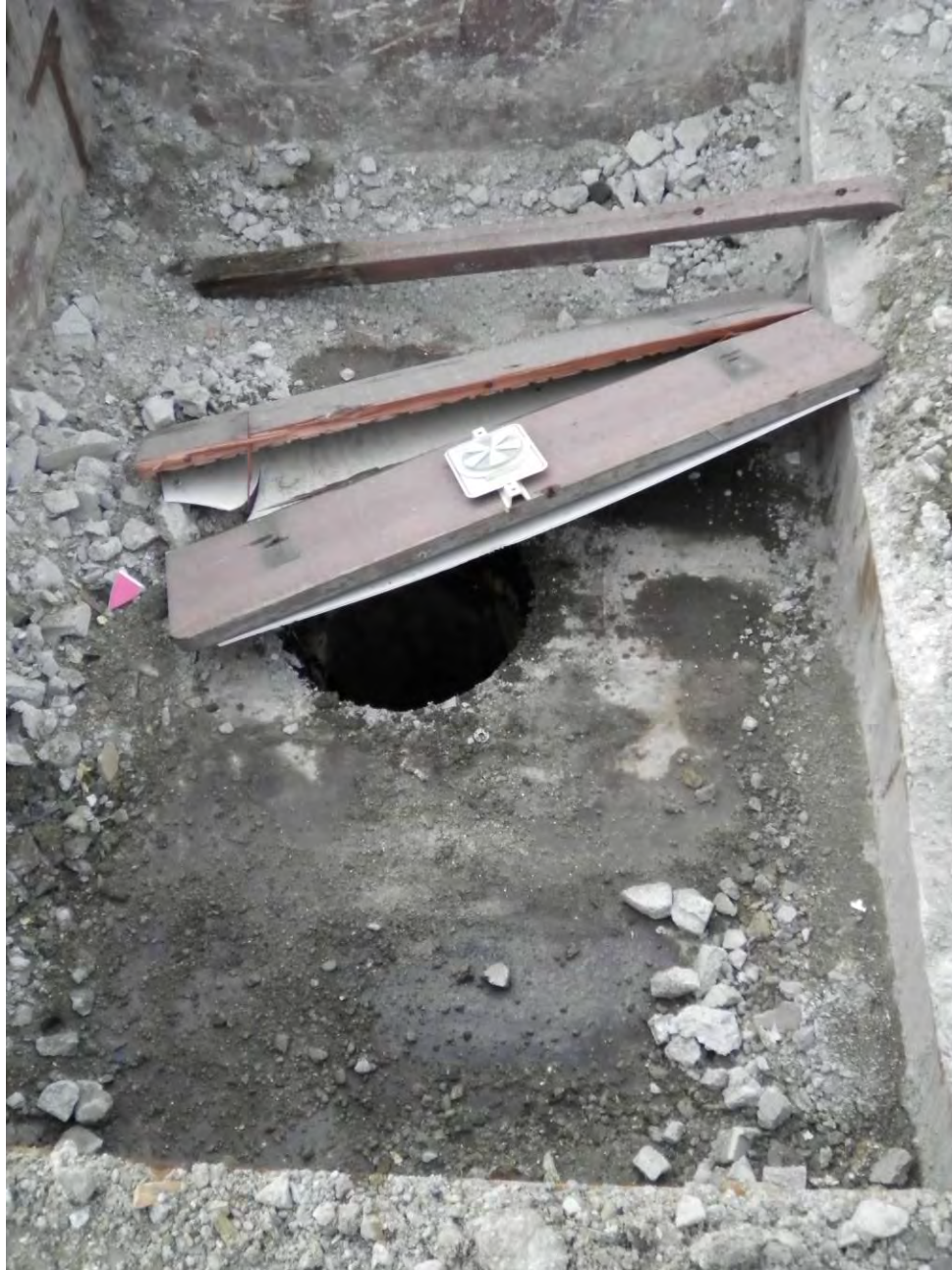
Photo 1: Former passenger elevator pit (AOI 30.1)
