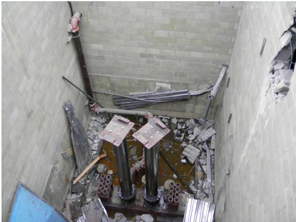
Photo 3: Former freight elevator pit (AOI 30.3)
