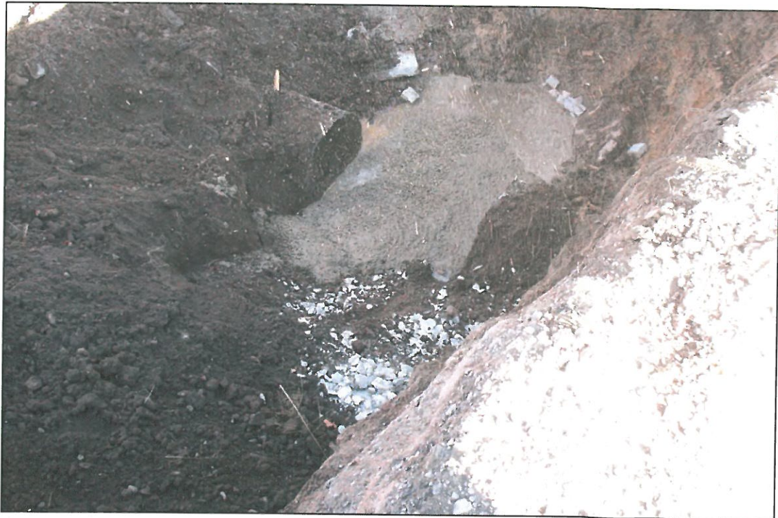
PHOTOGRAPH LOG MANHOLE/CHAMBER FA 19.5 (OCTOBER 24, 2011) FORMER SAGINAW MALLEABLE IRON PLANT Saginaw, Michigan
