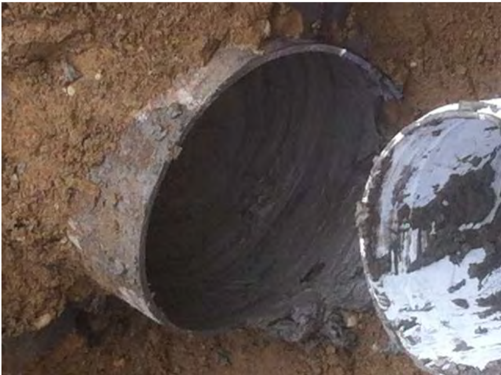
Photo 2: View cut and separated pipe and brick and cement in pipe of bulkhead location #1.
