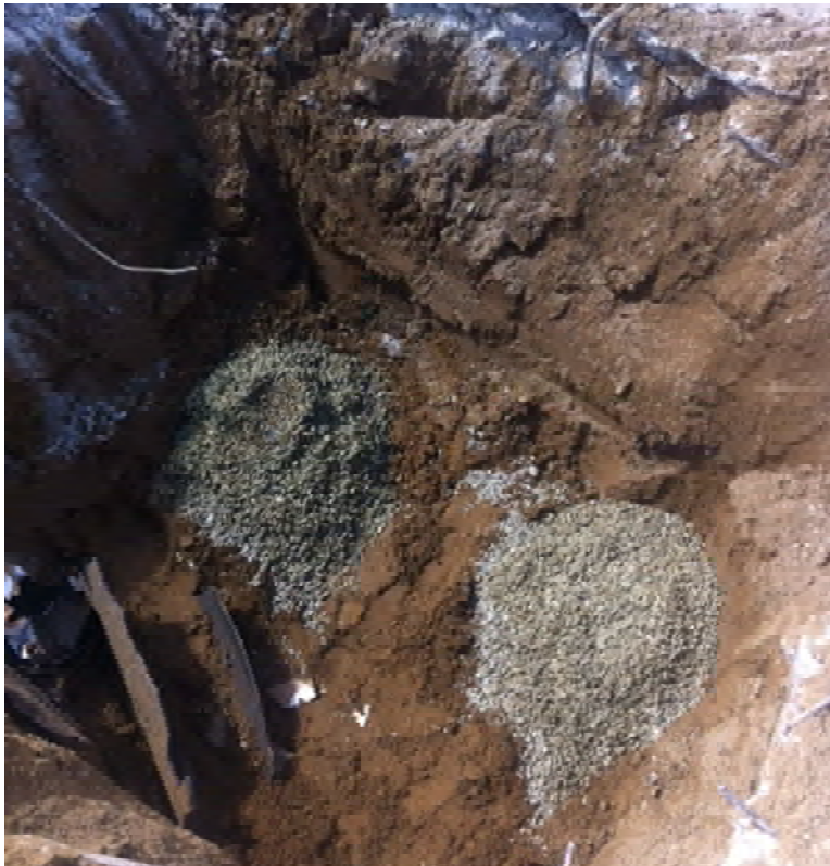
Photo 6: View of bentonite collar around lines at bulkhead location #3.
