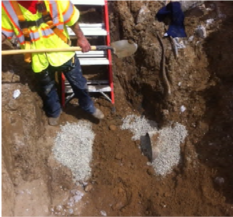
Photo 3: View of bentonite collar at bulkhead location #1.
