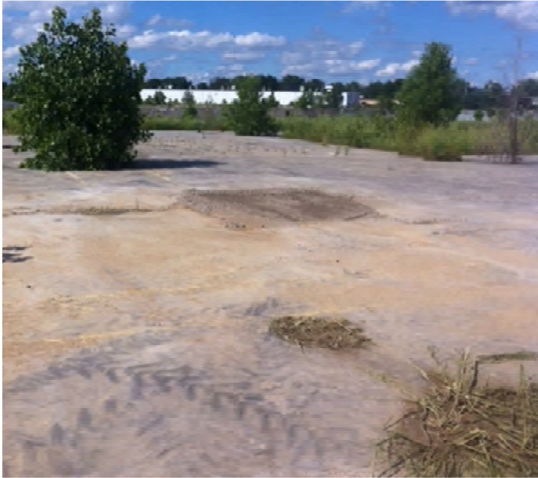
Photo 7: View of backfill at bulkhead locations.
