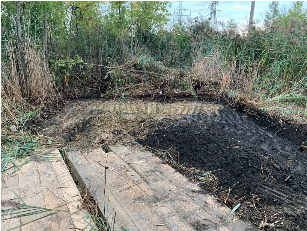
Photo 3 – Eastern Portion of Excavation Area – September 15, 2020
