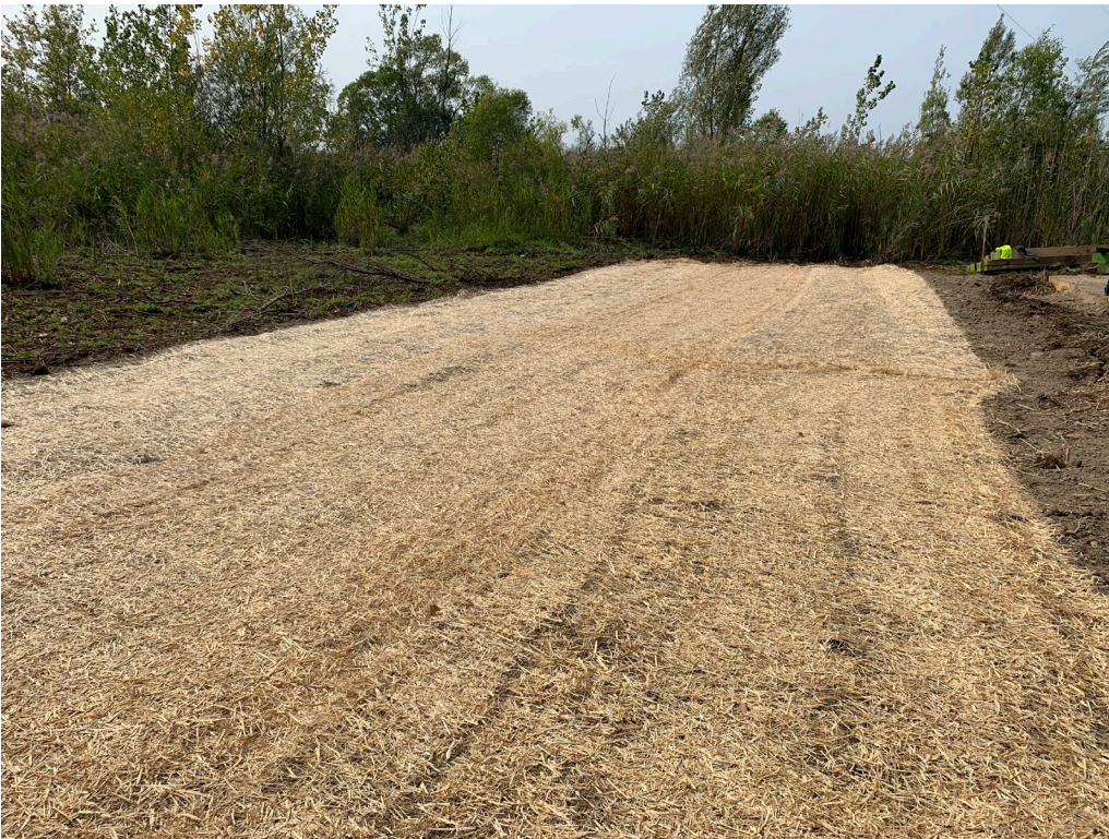
Photo 9 – Straw Mat for Restoration of Disturbed Soil, Facing West – September 17, 2020
