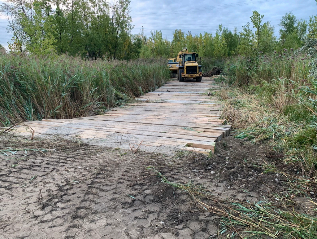
Photo 1 – Track Mats to Access Excavation Area Facing South – September 15, 2020
