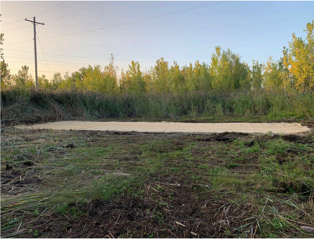
Photo 10 – Completed Site Restoration, Facing South – September 17, 2020
