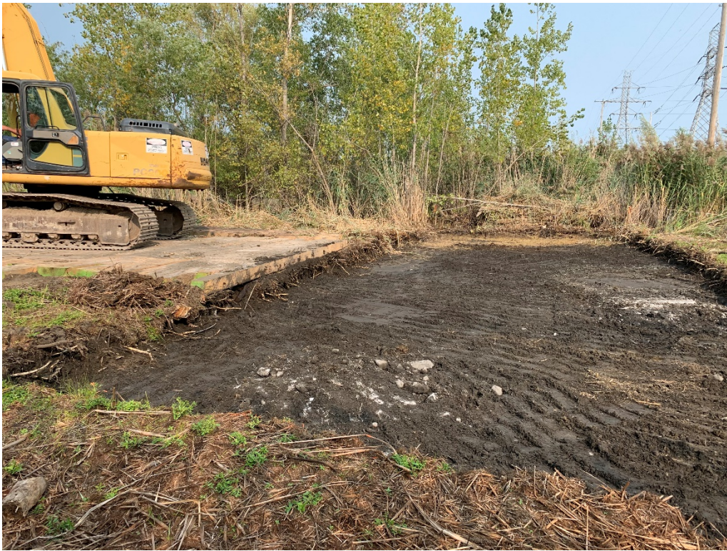
Photo 5 – Completed Excavation Area Facing East – September 16, 2020
