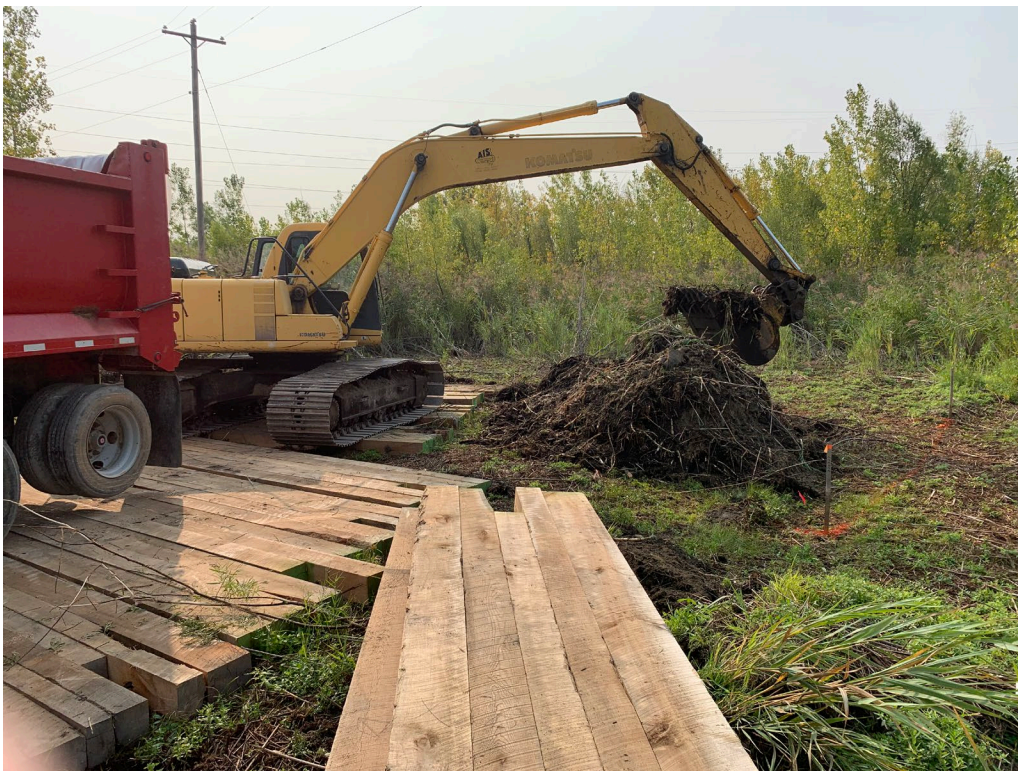
Photo 4 – Loading of Stockpiled Material from Excavation Area – September 15, 2020
