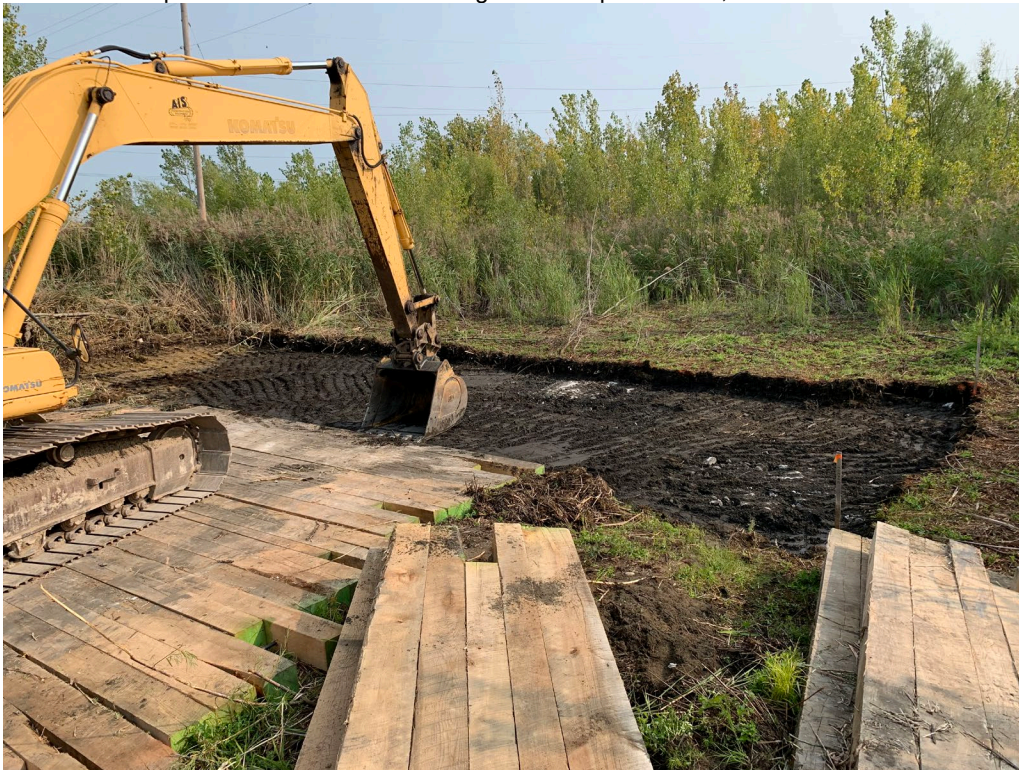
Photo 7 – Completed Excavation Area Facing Southeast – September 16, 2020
