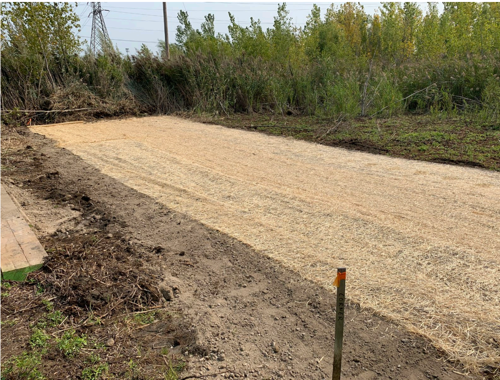
Photo 8 – Straw Mat for Restoration of Disturbed Soil, Facing East – September 17, 2020
