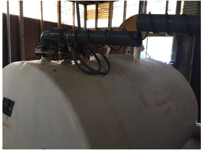
Photo #8: Influent piping cut and removed
