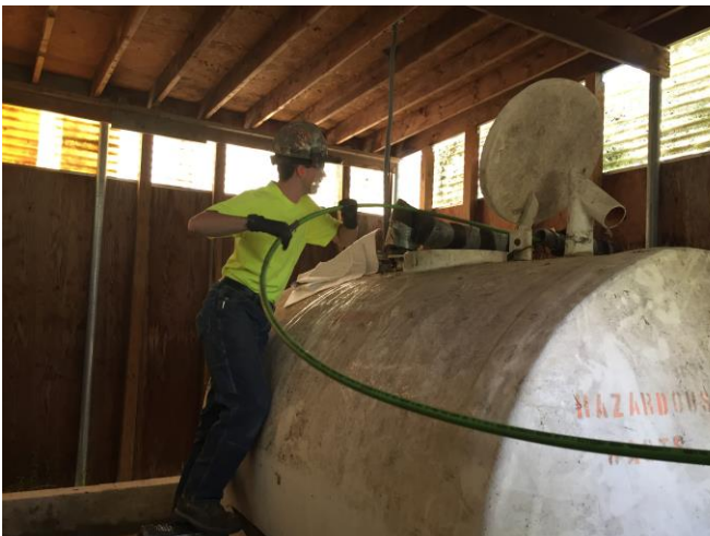
Photo #5: EMS Power washing interior of AST
