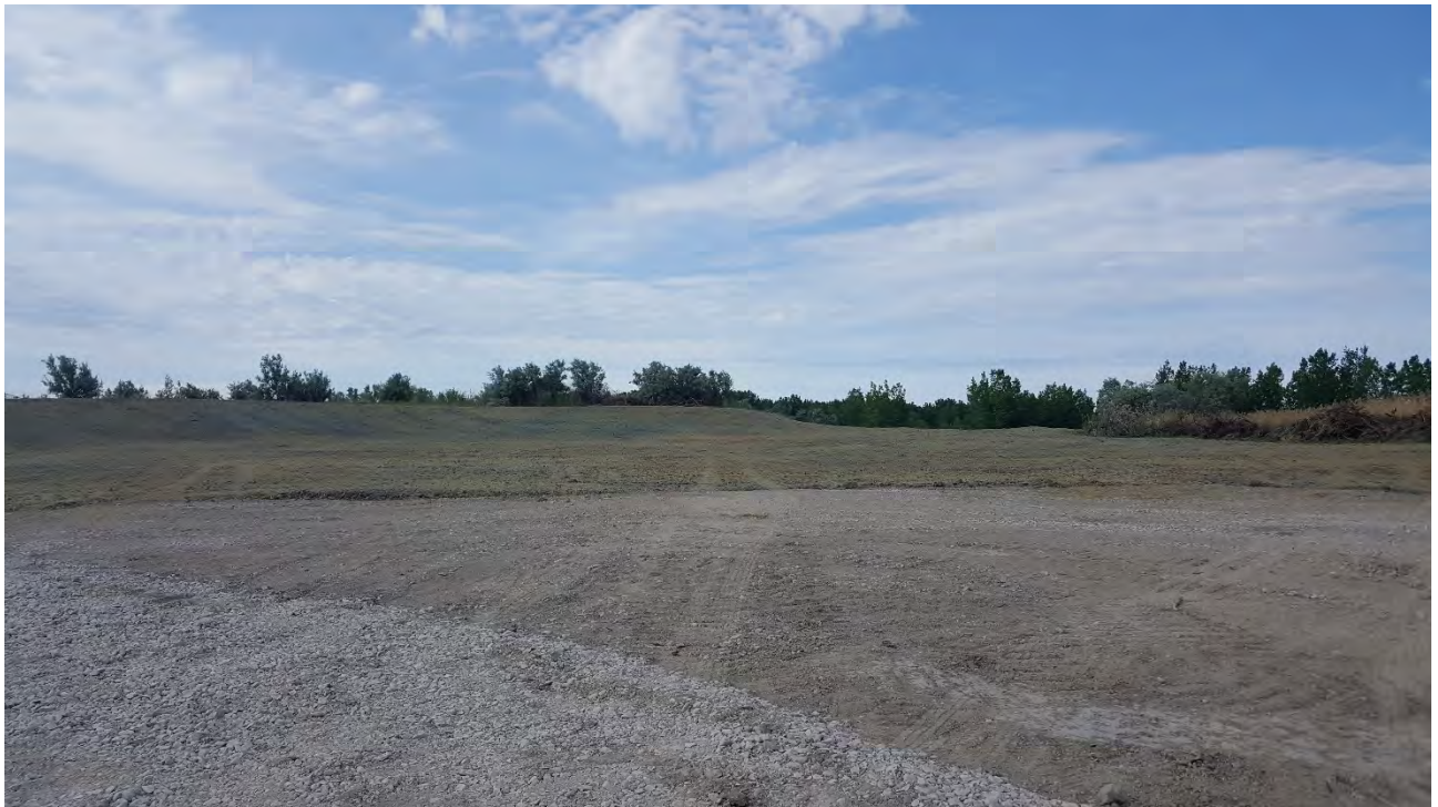
Photo 4 – June 16, 2016 – Nodular Clay Pile Restoration
