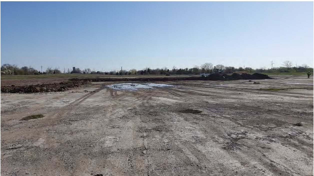
Photo 2 – April 24, 2017 – On-Going Clay Cover Placement
