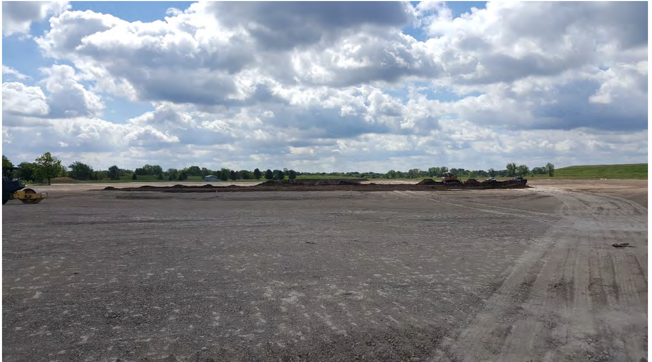
Photo 8 – May 31, 2017 – Topsoil Placement Over Clay Cover
