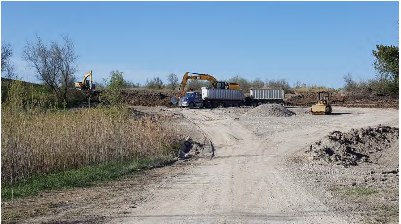
Photo 2 – May 12, 2017 – Clay Removal for Placement at Malleable
