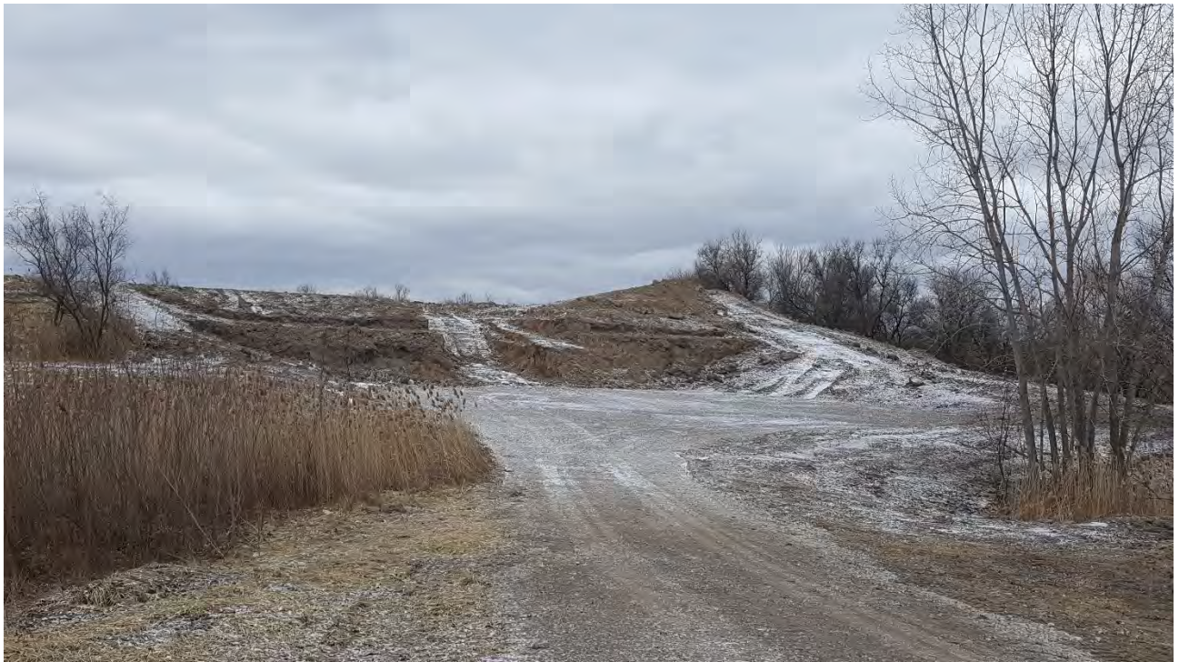
Photo 1 – February 15, 2017 – Setup of Clay Pile (incl. access road)
