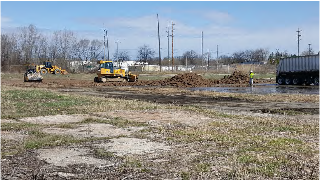
Photo 1 – April 17, 2017 – Initiating Placement of Clay Cover
