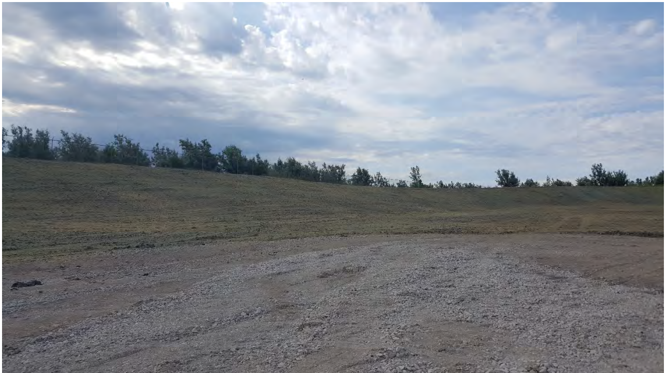
Photo 5 – June 16, 2016 – Nodular Clay Pile Restoration
