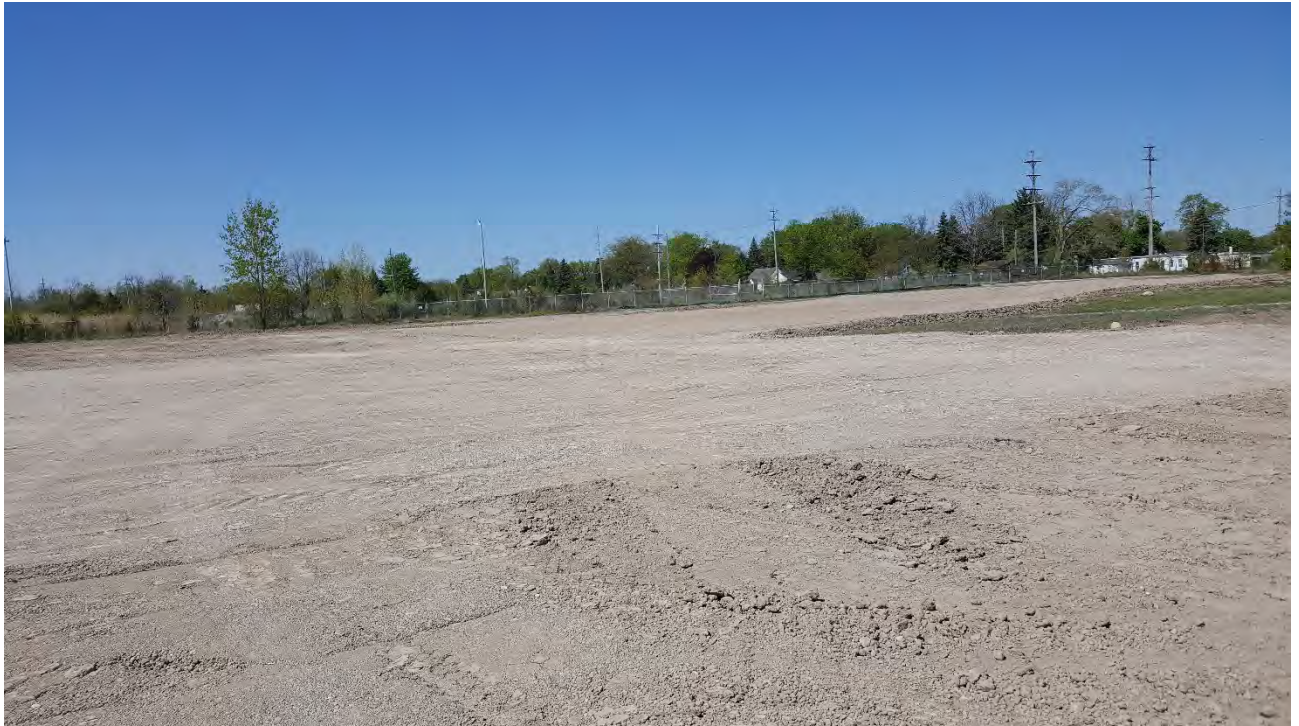
Photo 7 – May 12, 2017 – Clay Cover Placement over I27.7 Manhole Area
