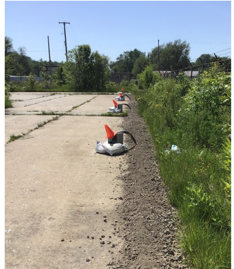
Biosparge Transect With Hoses Covered in Gravel
