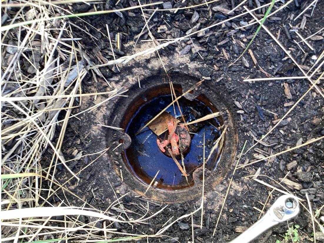
Photo 3: Inside of well with tubing and cap lock.
