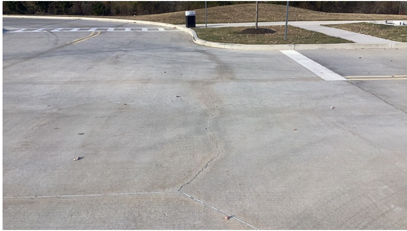
Photo 3 - View Looking West - View of Inspection from other entrance. This is where big trucks come in and out from loading.
