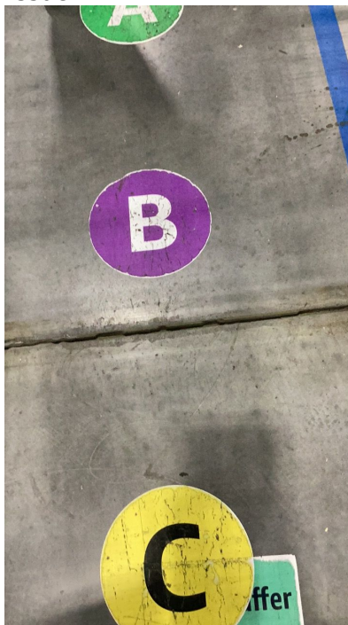
Photo 37 - View Looking South - Expansion joint with a crack that started from F-14 to B-14. Believe landlord is aware of this issue.
