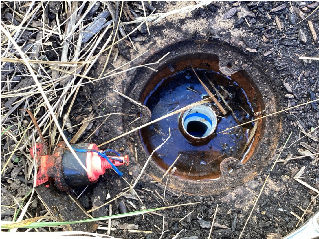
Photo 3: Inside of well with tubing and cap lock.
