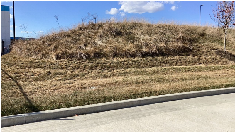
Photo 45 - View Looking West - Eroded area of grass near big hill area near trailer park.
