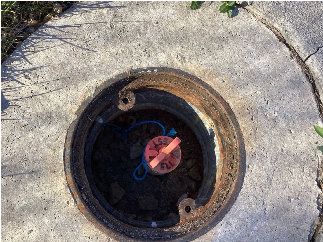
Photo 3: Well, diameter and tubing with Caplock.
