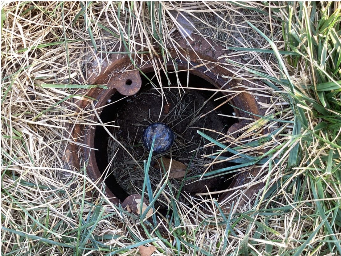
Photo 3: Inside of well with tubing.
