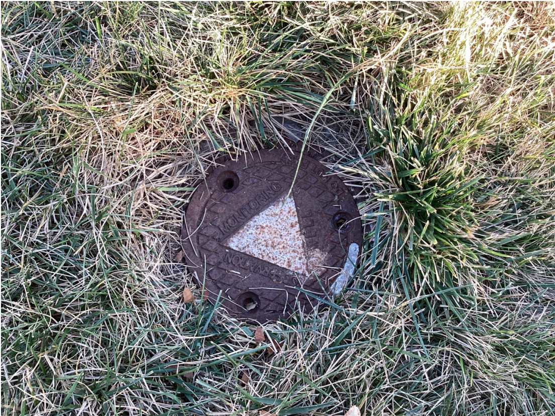
Photo 1: Outside of well.
