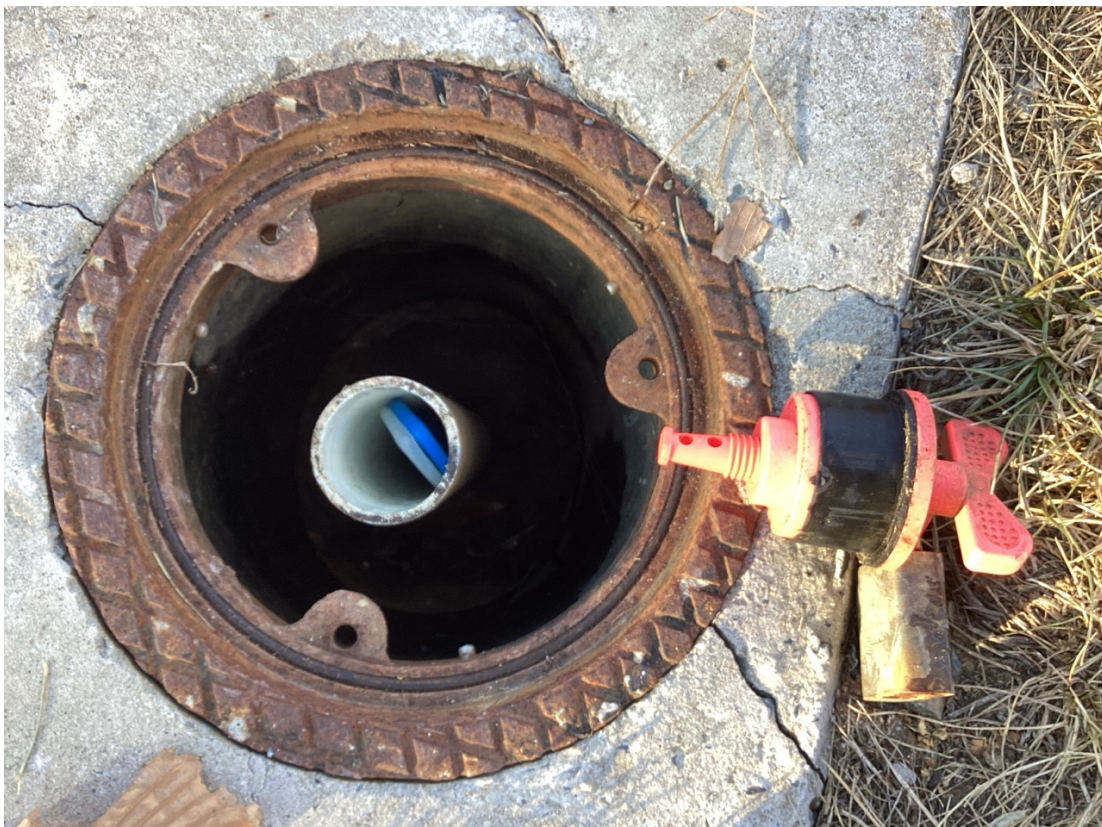
Photo 3: Ground water, tubing and cap lock and top of casing.
