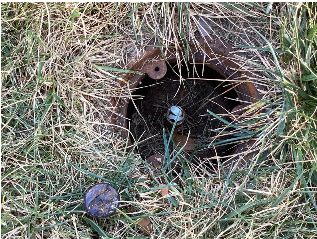
Photo 3: Inside of well with tubing.
