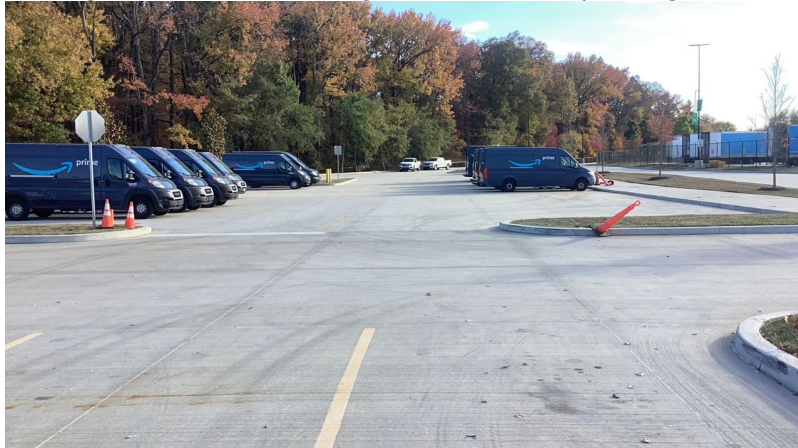
Photo 10 - View Looking South - You looking south of other parking lots and cap area.
