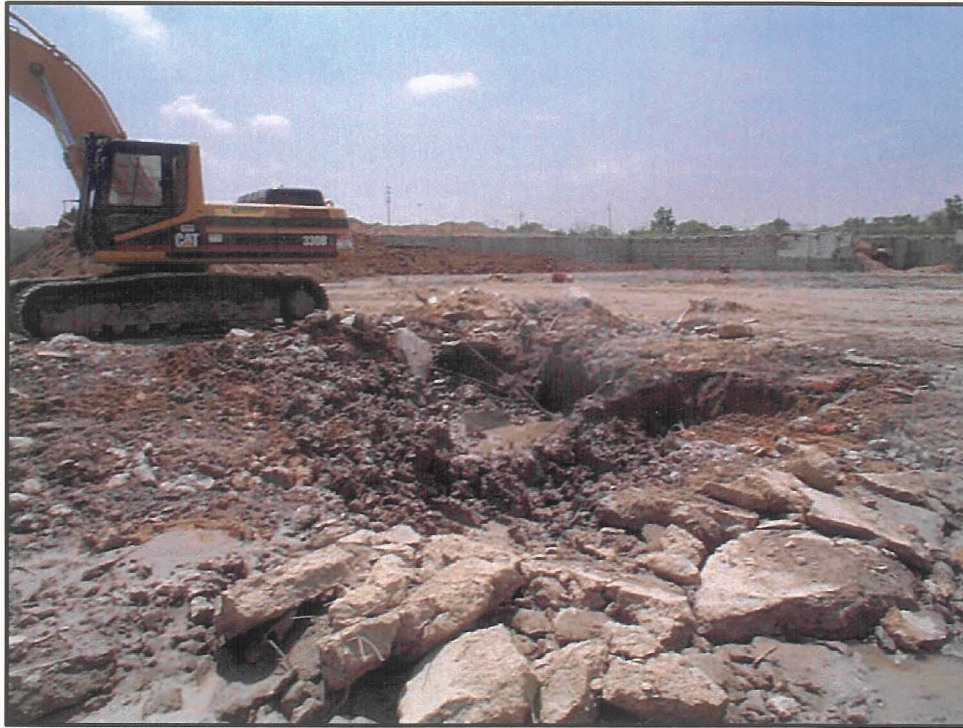
PHOTO 1 - JUNE 13, 2001 EXCAVATION OF HOT SPOT AT BH-9-26-00 LOOKING SOUTHEAST
