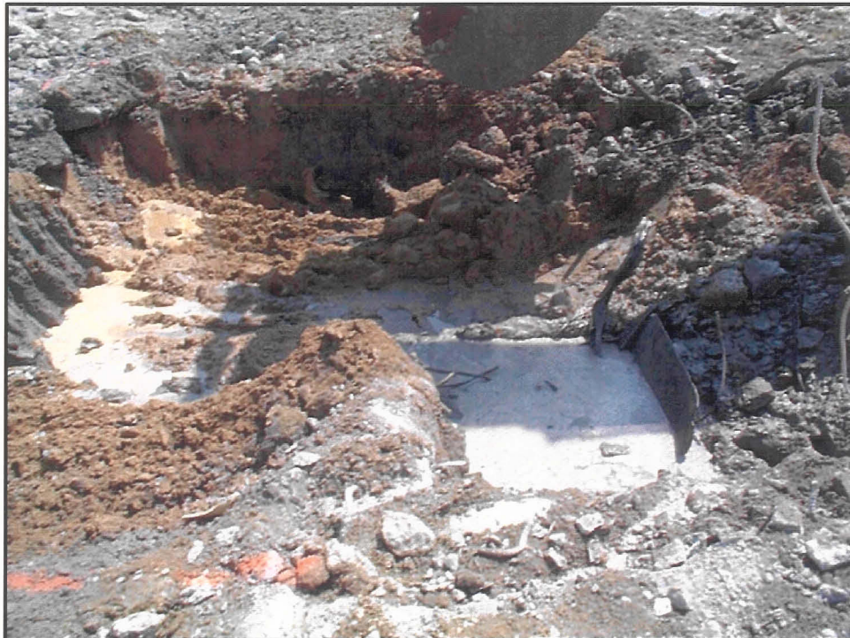
PHOTO 3 - JUNE 13, 2001 EXCAVATION OF HOTSPOT AT BH-9-26-00
