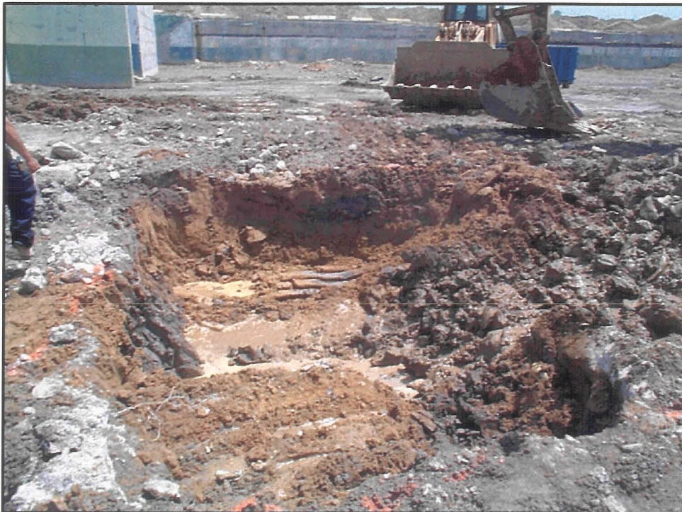
PHOTO 2 - JUNE 13, 2001 EXCAVATION OF HOT SPOT AT BH-9-26-00 LOOKING EAST
