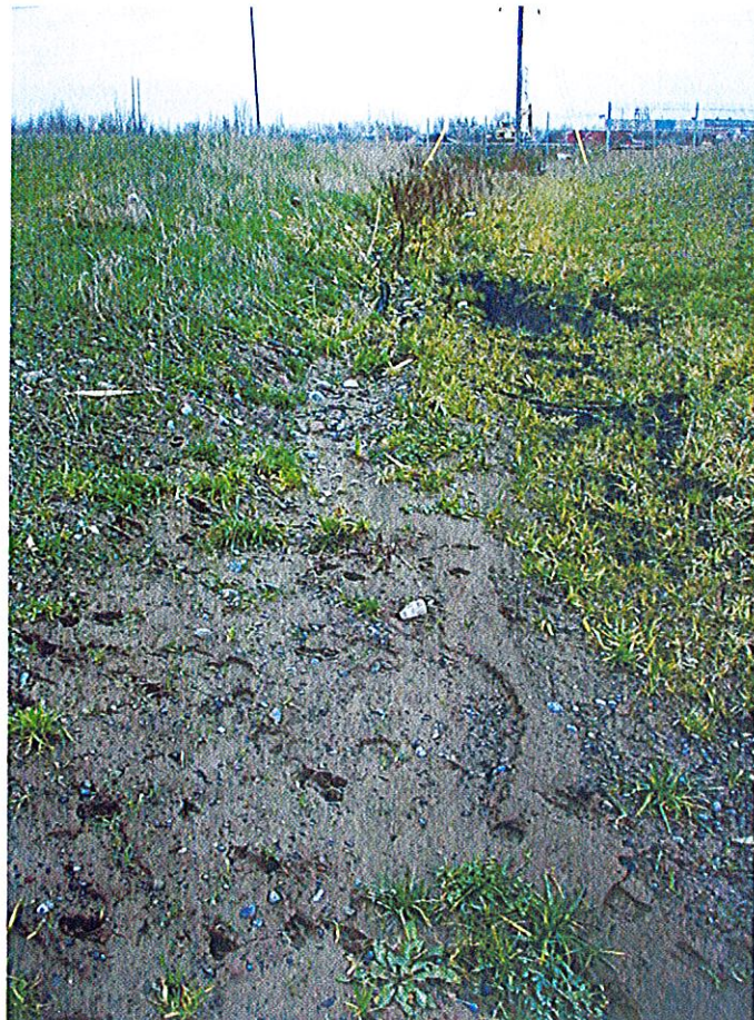
Photo 14 - View or erosion in CB-1 overflow spillway.
