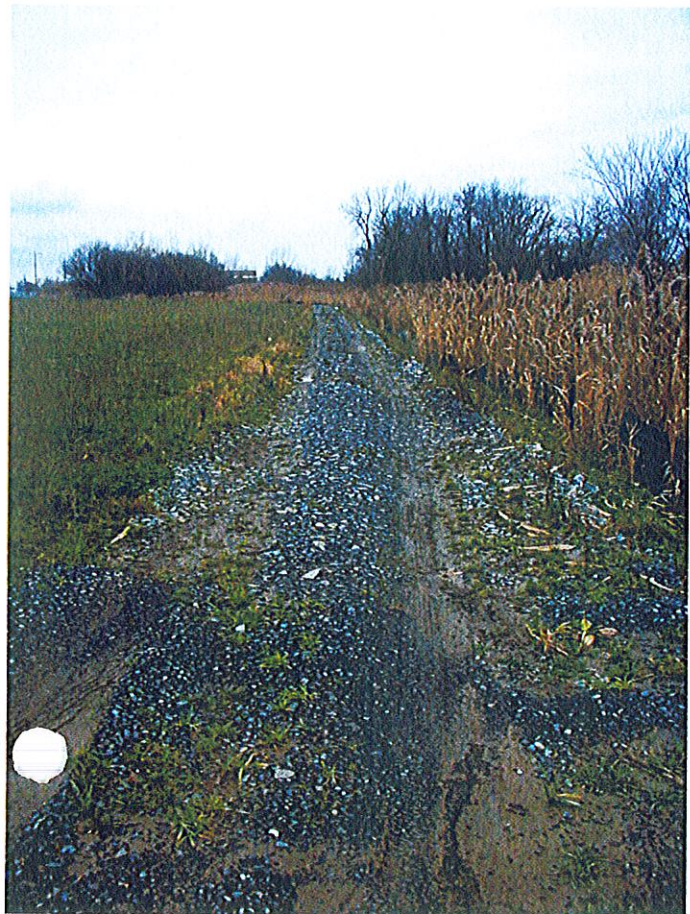
12/14/01 Photo 19 - View of ruts in access road heading west from CB-1.
