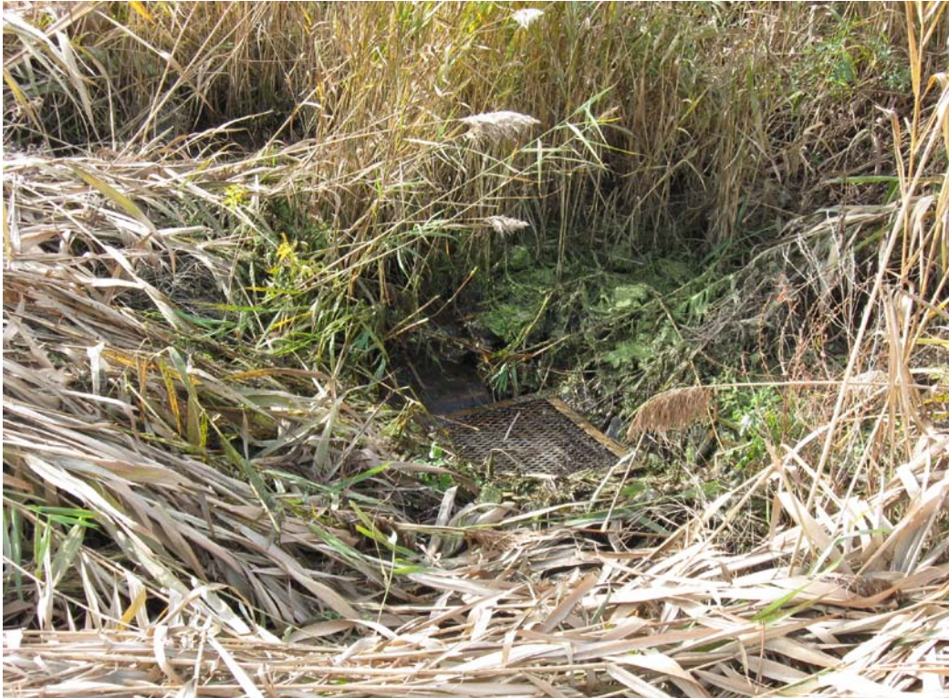
Photograph 16: View of CB-03 after cleaning.
