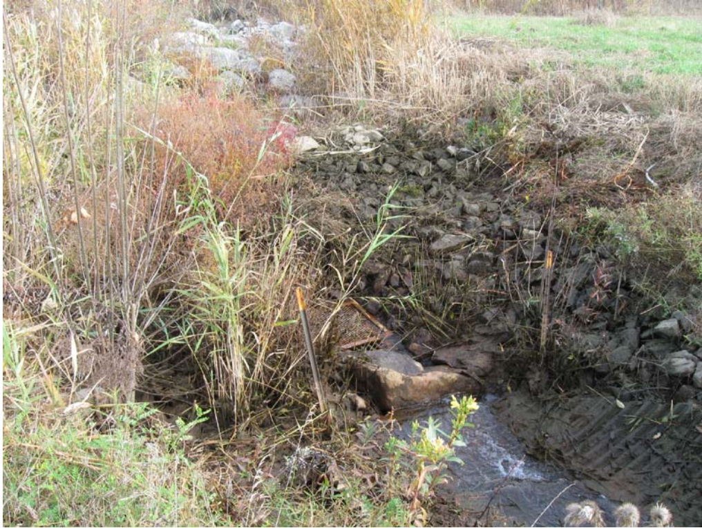
Photograph 17: View of CB-04 after cleaning.
