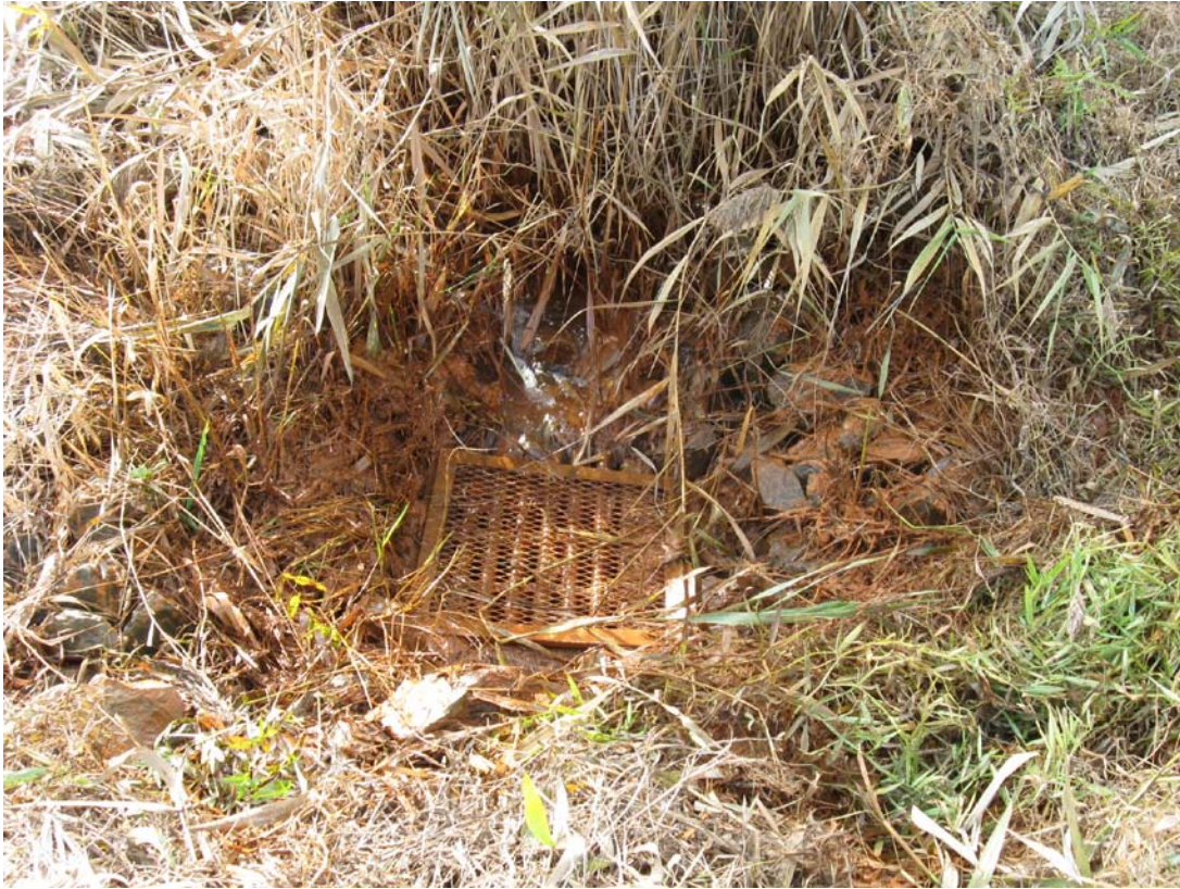
Photograph 15: View of CB-02 after cleaning.
