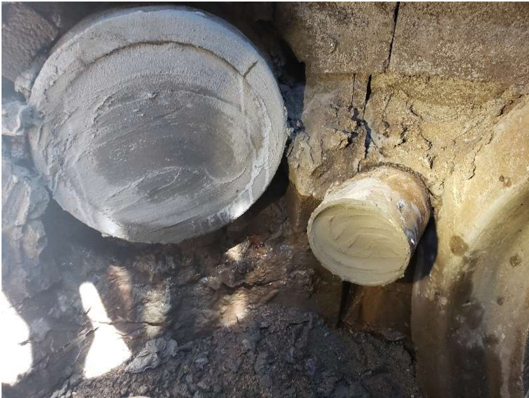
Two sealed plugs in laterals.
