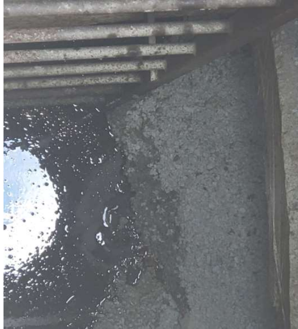
Bentonite placed in manhole prior to filling with concrete.
