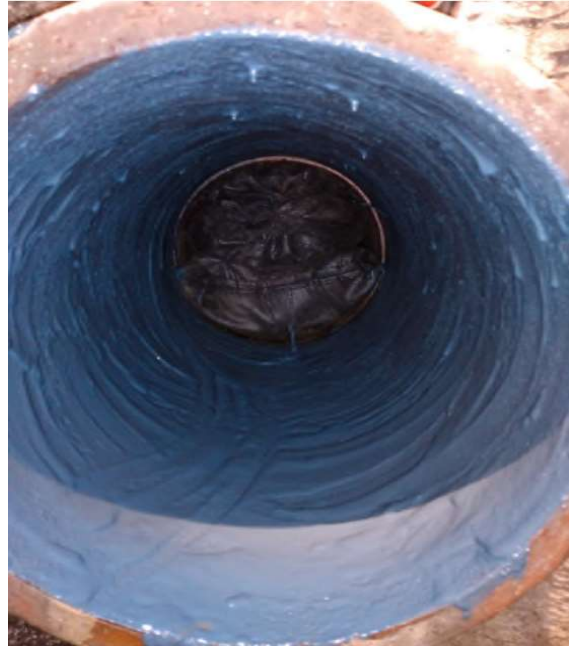
Sandbags installed inside pipe to block flow while bonding agent cures.
