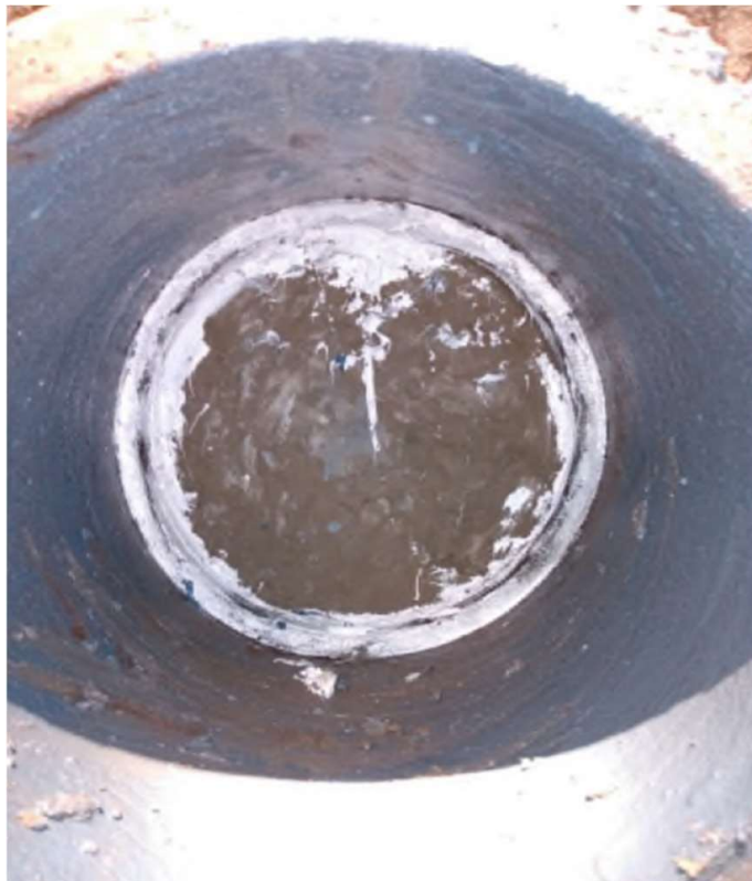
Water stop and adhesive added to back side of plug.
