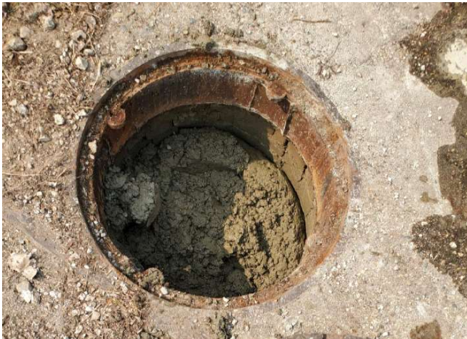
Manhole partially filled with concrete. Small pours completed to eliminate voids.
