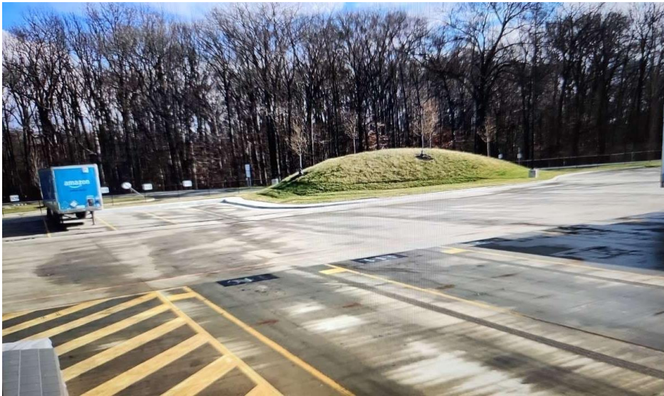
Photo 14 View Looking East - Cap trailer parking
