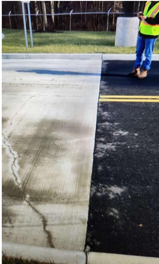
Photo 6 View Looking East - SE edge of cap
