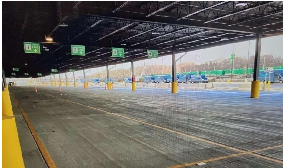
Photo 5 Outside looking N/NW of warehouse
