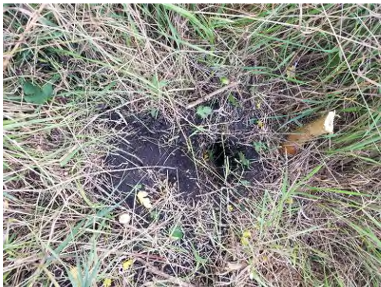
Photo 1. Small animal burrow on the north side of the north Type III Landfill.
