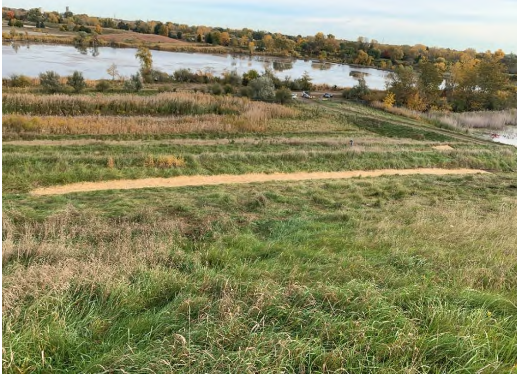
Photo 3: Erosion blanket installed over area on northeast side of GPL.
