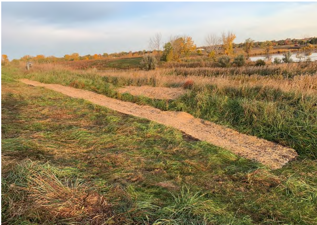
Photo 2: Erosion blanket installed over area on northeast side of GPL.
