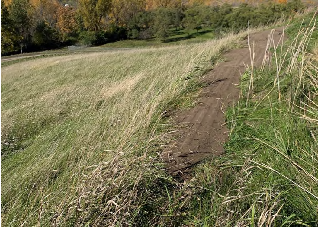
Photo 17: Area on northwest side of GPL after filling in with topsoil.
