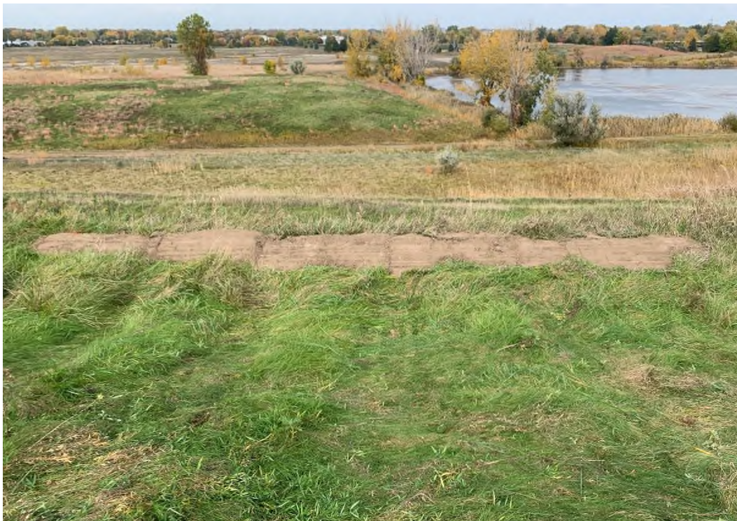
Photo 4: Area on north side of GPL after filling with topsoil.
