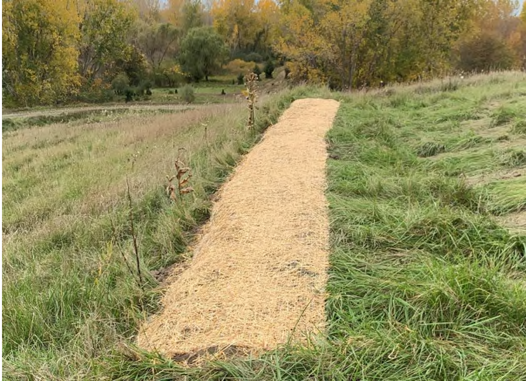
Photo 13: Erosion blanket installed over area on southwest side of GPL.
