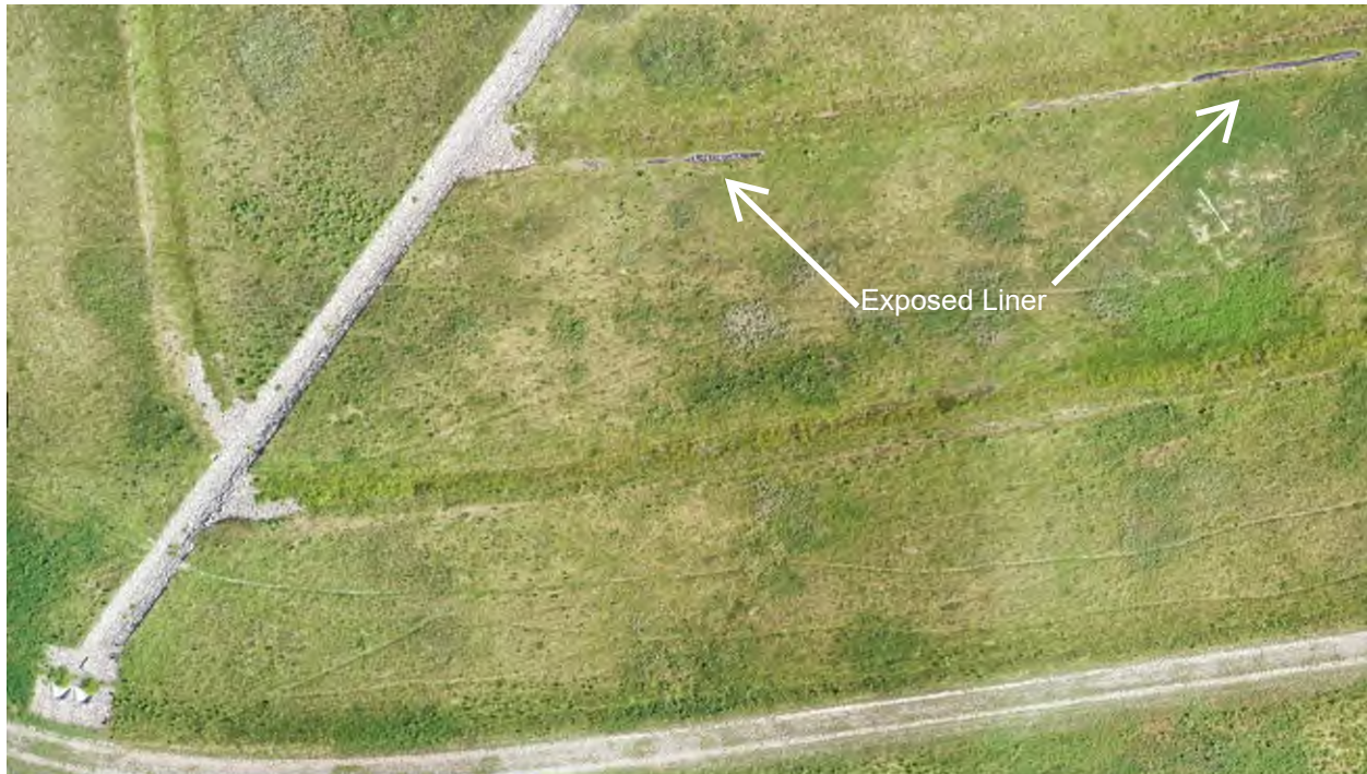
Photo 1: Green Point Landfill, southwest corner of landfill showing mid-slope drainage swale with exposed surface cover liner.
