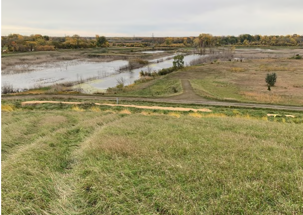
Photo 9: Erosion blanket installed over area on southeast side of GPL.
