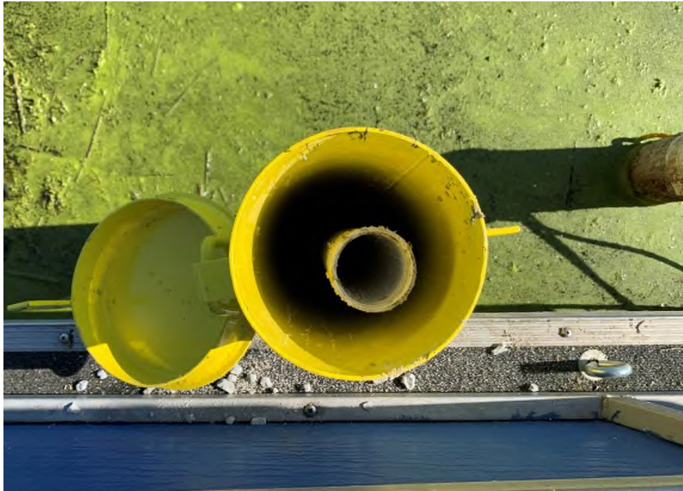
Photo 1: Well casing extended using a PVC coupling and riser section and protective well cover extension added that is designed to fit tightly over existing protective cover and add more length.
