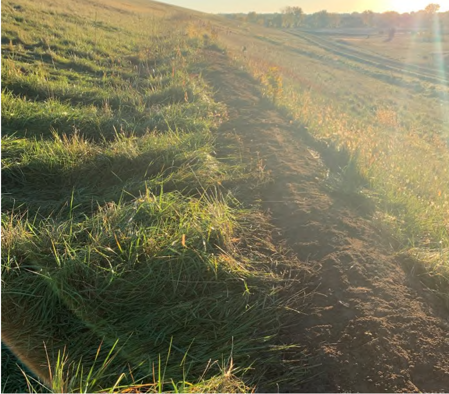
Photo 11: Area on southwest side of GPL after filling in with topsoil.
