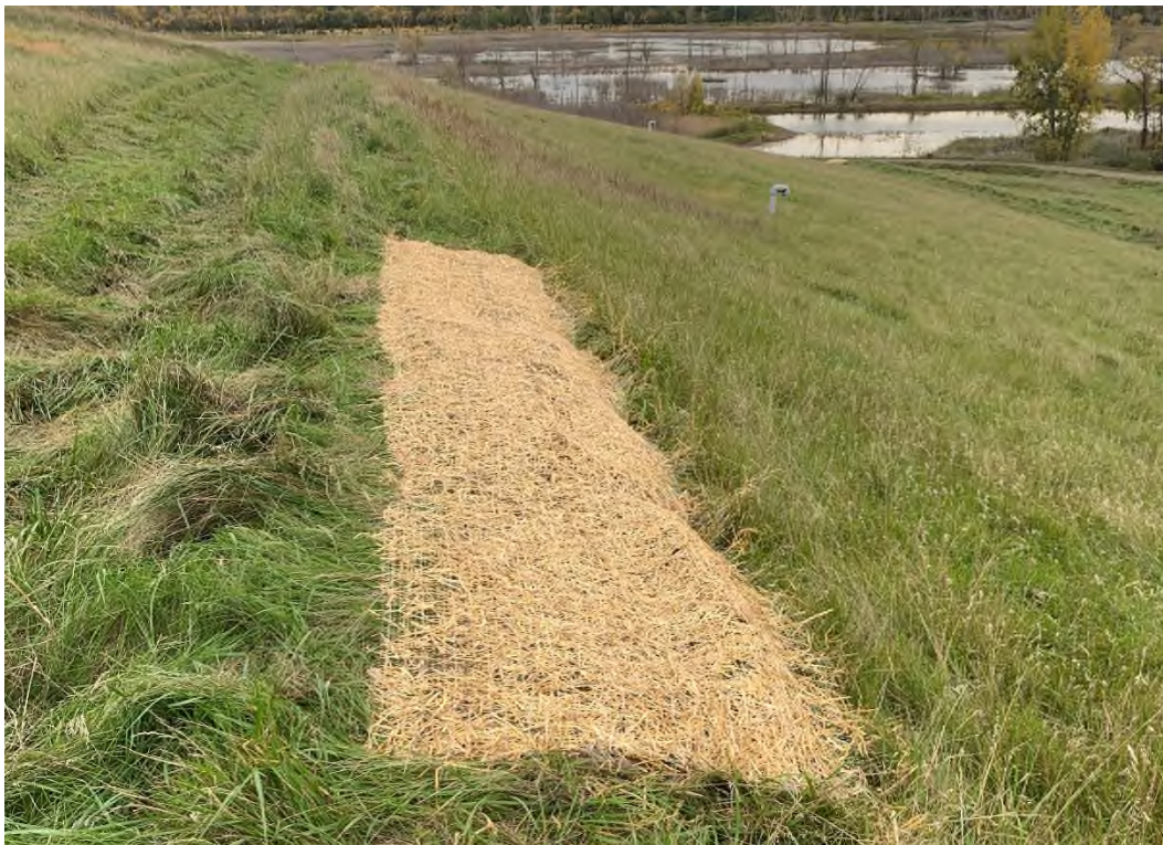
Photo 18: Erosion blanket installed over area on northwest side of GPL.
