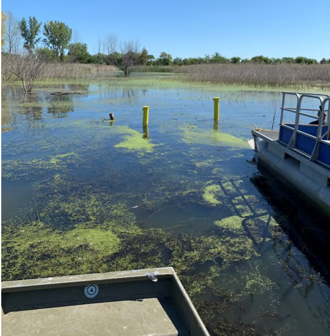
Photo 3: MW-117WT and NW-117S1 series showing completed riser and protective cover extensions raised above waterline and additional seal along well casing.
