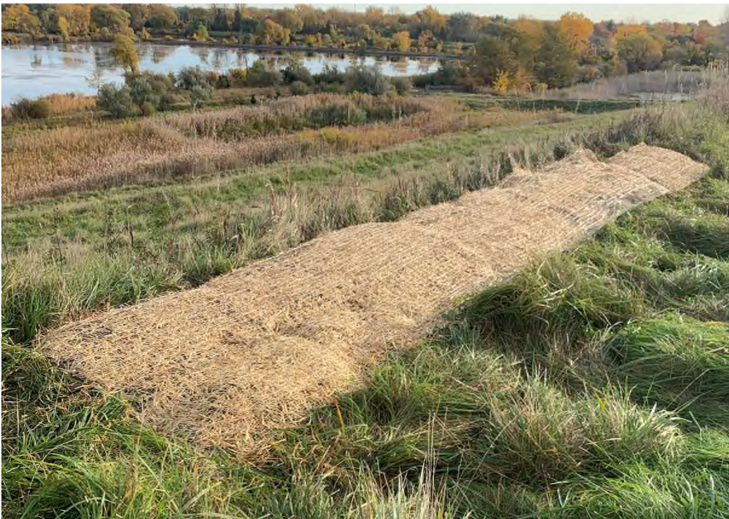
Photo 6: Erosion blanket installed over area on north side of GPL.
