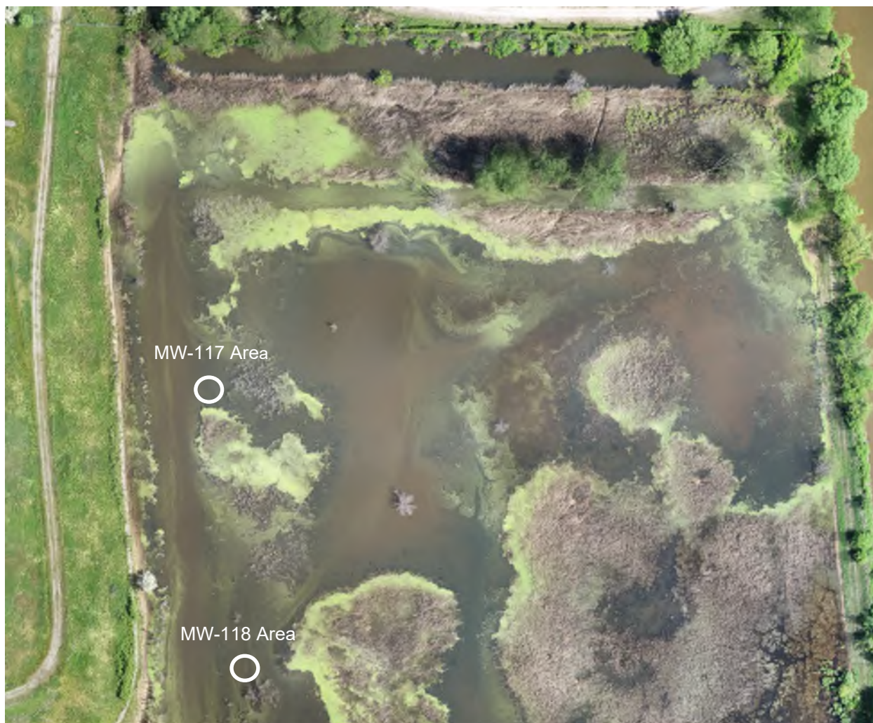
Photo 3: Eastern Property Extension of GPL along east edge of Green Point Landfill showing high water areas including MW-117's and MW-118's, and X-2A fully or mostly underwater.
