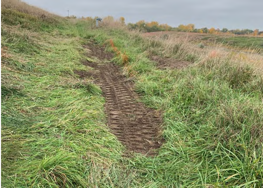
Photo 1: Area on northeast side of GPL after filling with topsoil.
