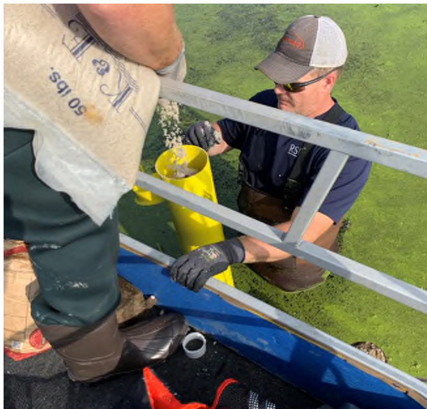
Photo 2: Adding bentonite-concrete slurry to seal then sand to set in place.
