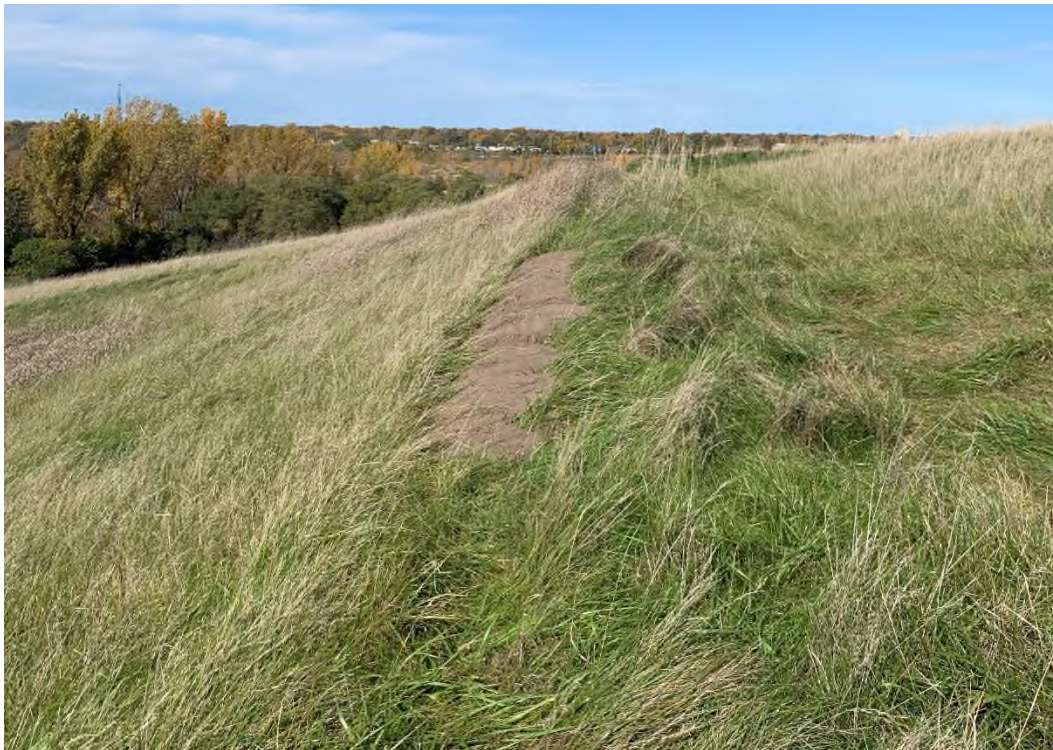
Photo 16: Area on northwest side of GPL after filling in with topsoil.
