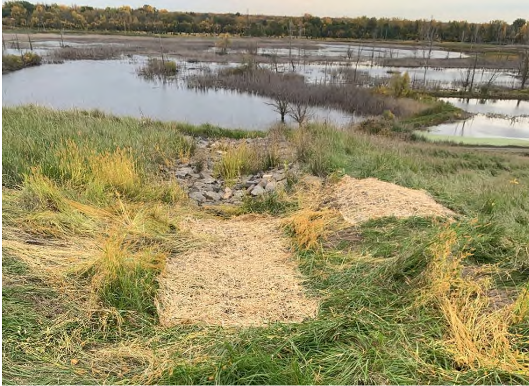
Photo 15: Erosion blanket installed over area on southwest side of GPL.
