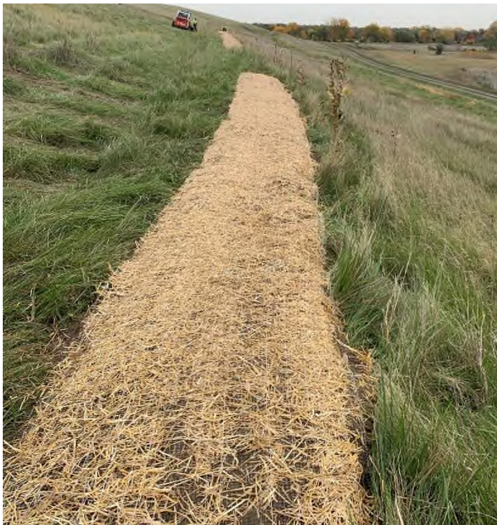
Photo 14: Erosion blanket installed over area on southwest side of GPL.
