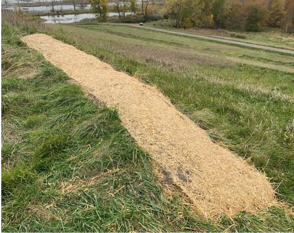
Photo 19: Erosion blanket installed over area on northwest side of GPL.
