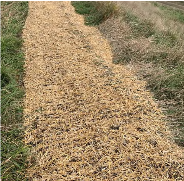
Photo 8: Erosion blanket installed over area on southeast side of GPL.
