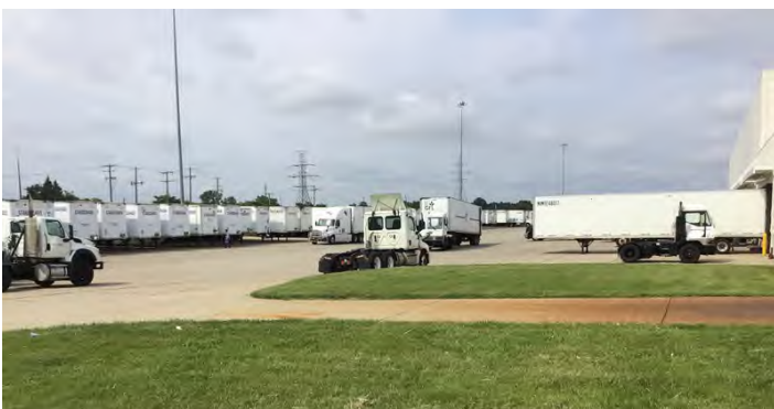
Photo of Concrete surfaced trailer storage and loading dock area at USPS southeast PCB Cap area facing west-southwest
