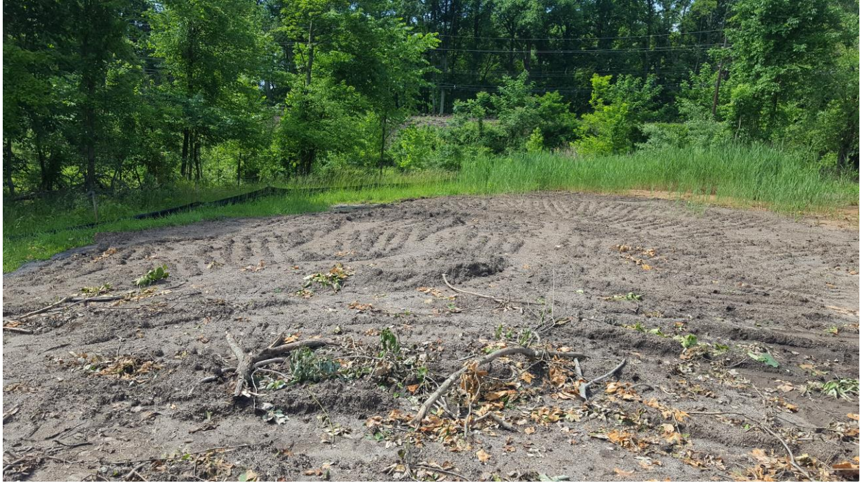
Photo C- View south of area B-21 showing the restoration area containing proper topsoil and prepared for seeding.
