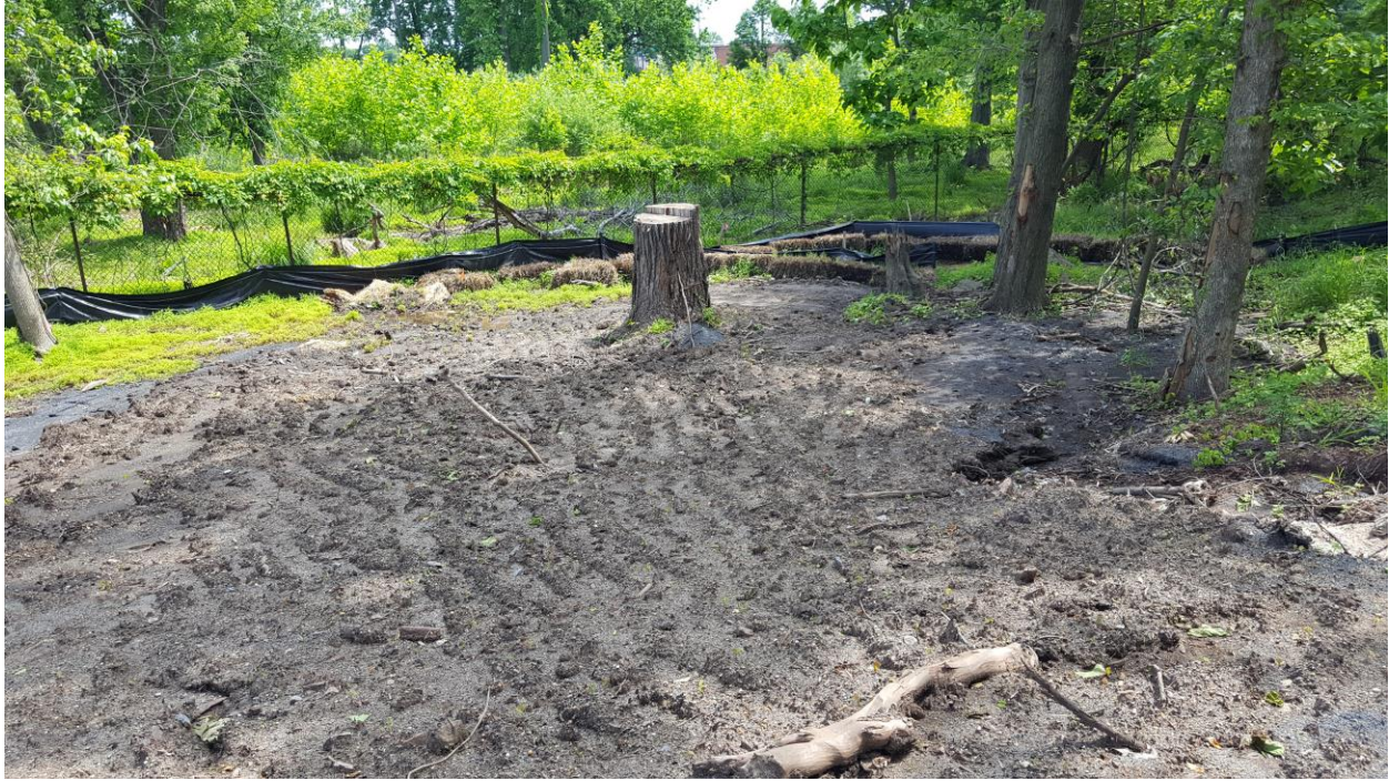
Photo A- View north of the restoration area in the vicinity of B17, B18 & B19 showing restored topsoil and preparation for native seeding. Note the removal of the felled tree for safety reasons. (May 2018)
