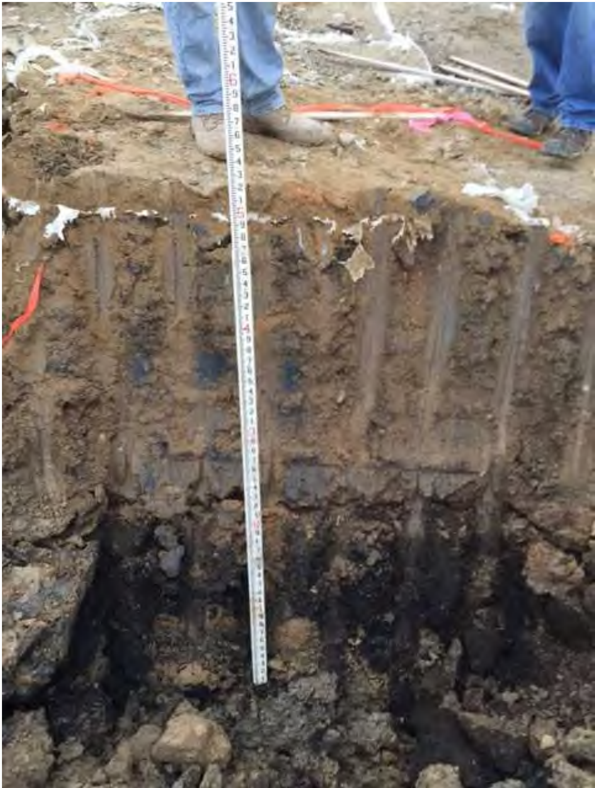
Excavation C facing east sidewall at 1.5 foot over excavation
