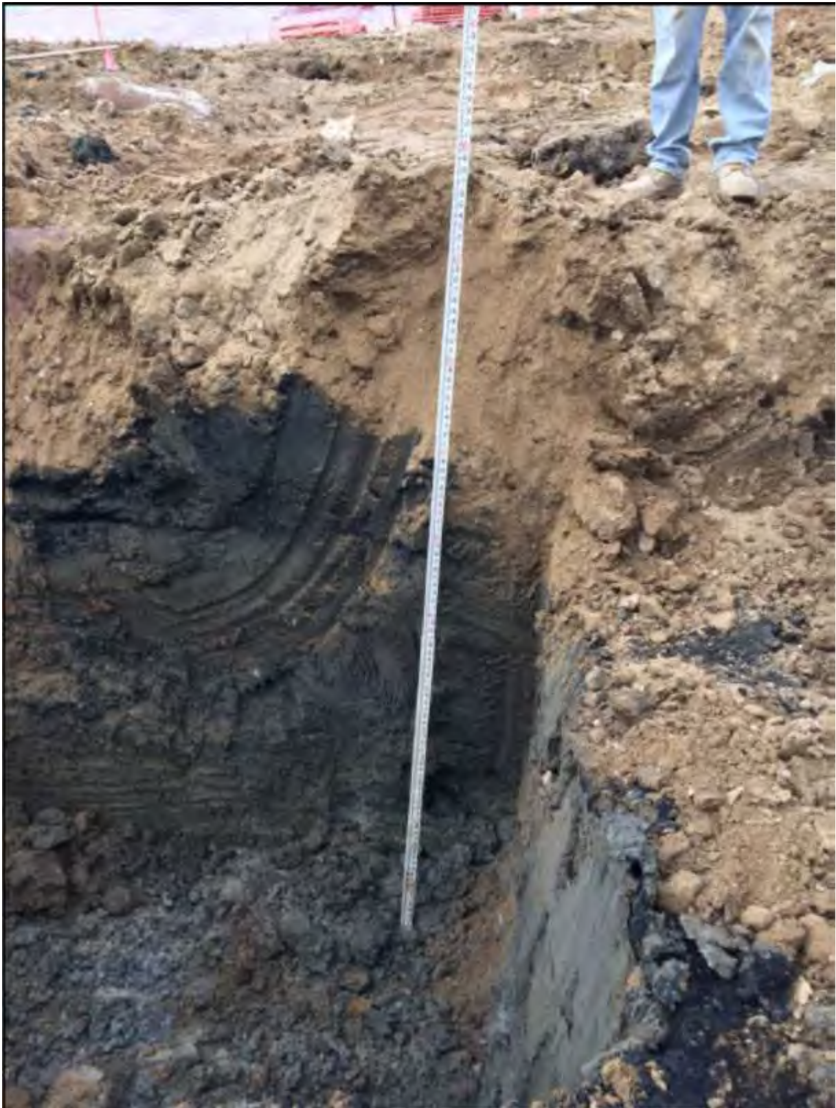
Excavation D facing Northeast corner
