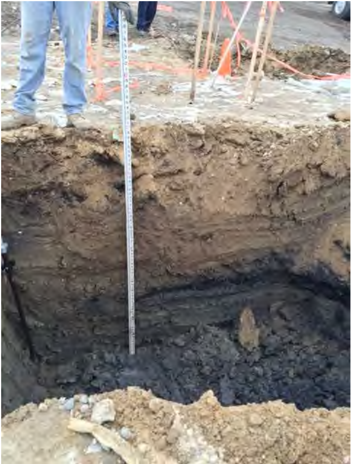
Excavation A facing North sidewall
