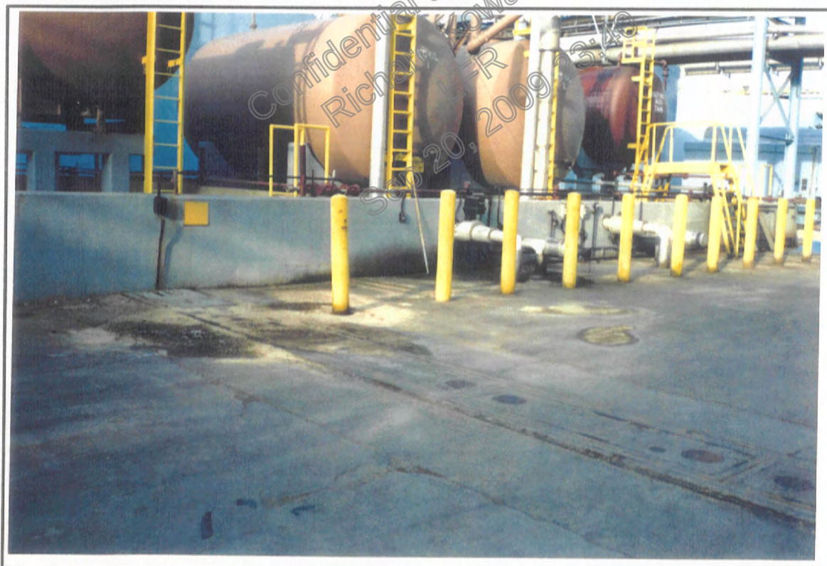
PHOTOGRAPH 6: STAINING NEAR AST FARM
