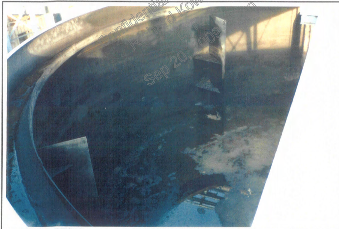
PHOTOGRAPH 2: CONTENTS OF OILY WASTE TANK NO.3
