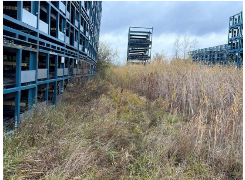
PP11, Facing North
