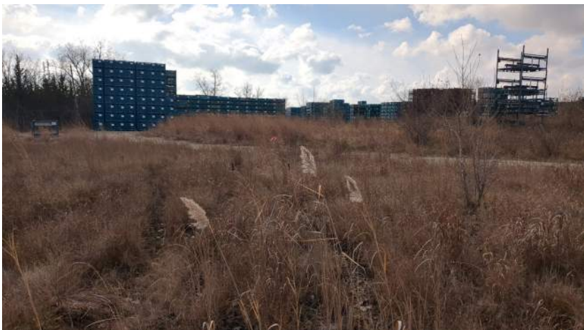
WSP.I, Facing South
