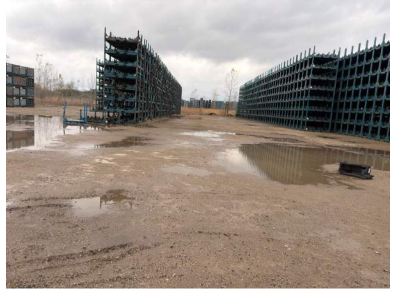
PP13, Facing North
