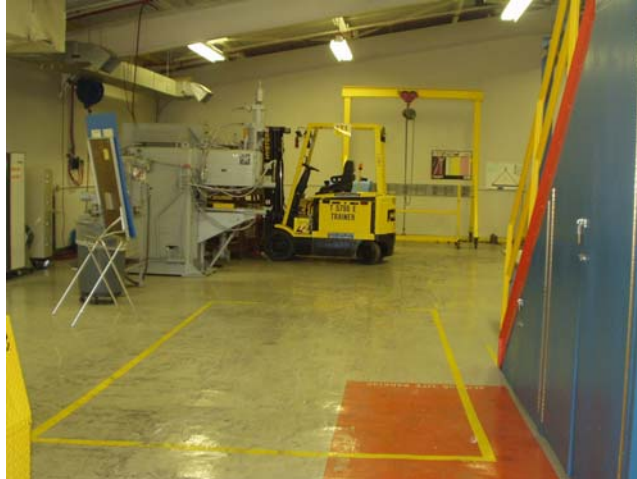
Photograph 15. View of garage area in 1 st floor where abandoned underground hydraulic lifts and floor drain were observed.
