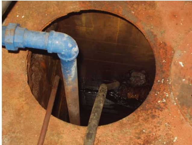
Photograph 13. View of the sump located in the boiler room of the basement.
