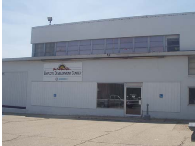
Photograph 4. View of the northeastern wall of the Site building, facing northwest.
