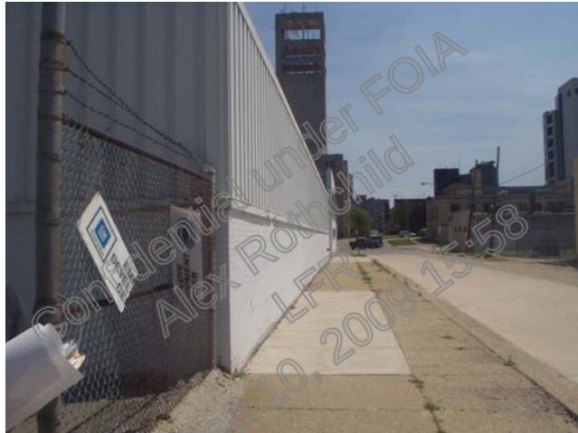
Photograph 5. View of the western wall of the Site building, facing southeast.
