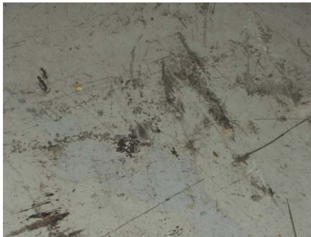
Photograph 17. View of abandoned underground hydraulic lift in the garage area.
