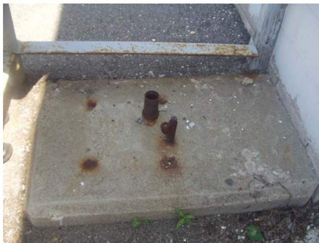
Photograph 9. View of former gasoline dispenser location outside the northeast corner of the Site building.
