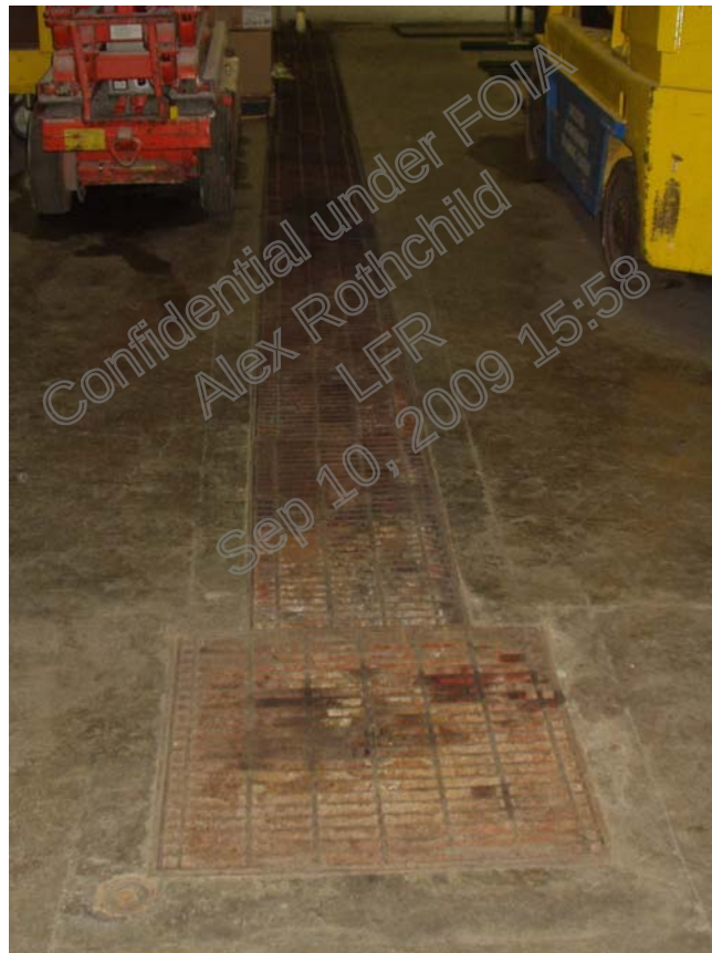
Photograph 14. View of the trench drain and adjacent sump located in the basement.
