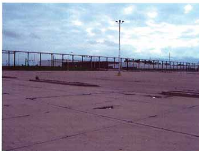
Photograph 12. View of Site from eastern boundary, facing southwest.
