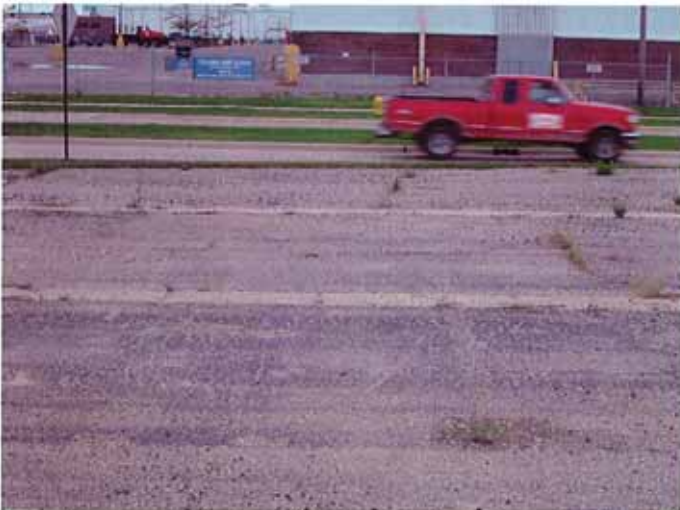
Photograph 9. View of concrete footers, facing south, Columbia Avenue in background.
