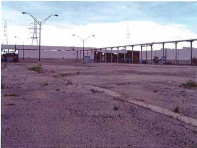
Photograph 8. View of Site and concrete footers, facing northwest.
