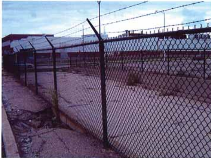
Photograph 7. View of former entrance to Plants 25 and 33, facing southwest.
