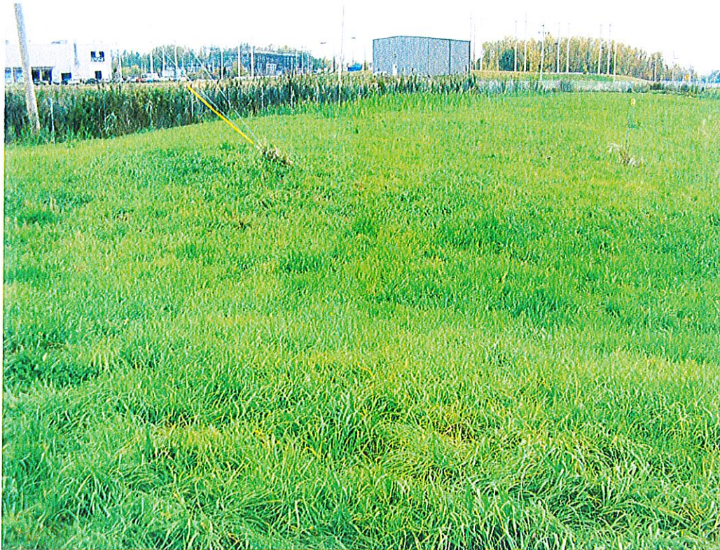
Photograph 1: Looking at east from CB-1 overflow spillway.
