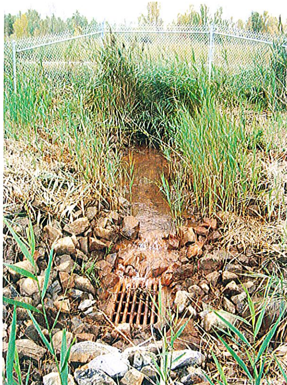
Photograph 13: View of repaired erosion areas within CB-2 overflow spillway.
