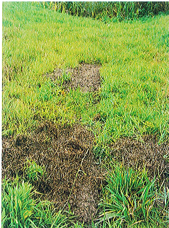
Photograph 10: View of repaired erosion areas within CB-3 overflow spillway.
