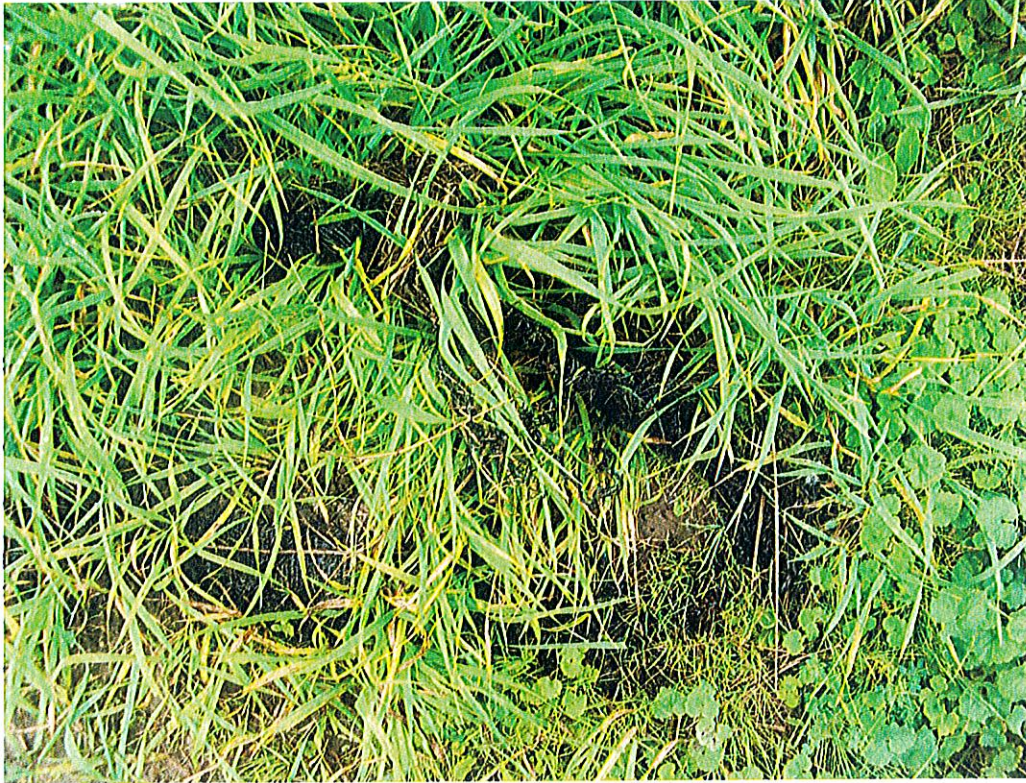
Photograph 11: View of exposed erosion control fabric within CB-3 overflow spillway.
