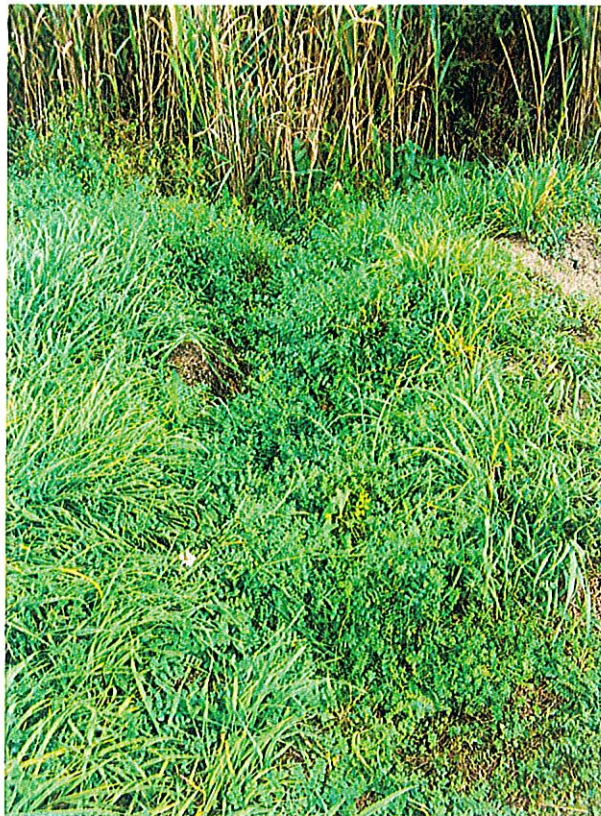
Photograph 7: View of erosion channel near CB-3 along fenceline.
