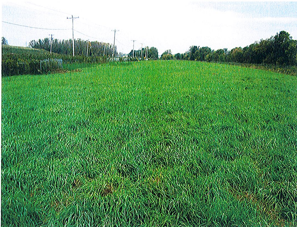
Photograph 15: View looking west from CB-2 overflow spillway.
