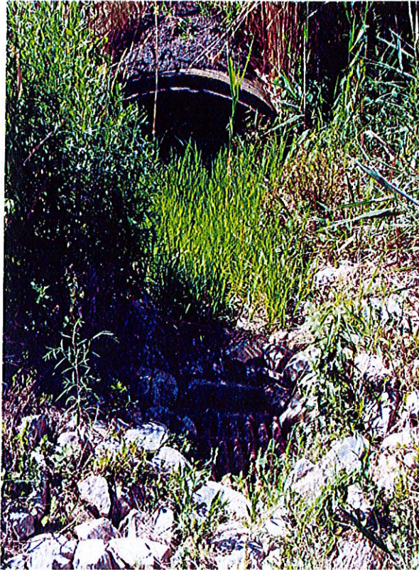
Photograph 1: View of CB-5/Outfall 004 spillway.
