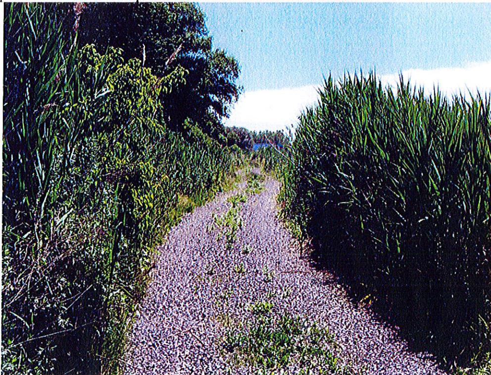
Photograph 8: View looking east from CB-3 outlet at repaired access road.
