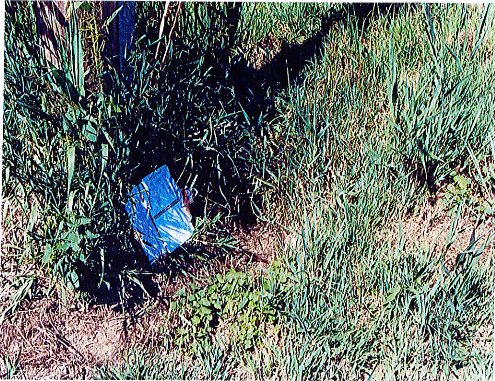
Photograph 5: Burrowing animal hole along fenceline southeast of OBG-21D.
