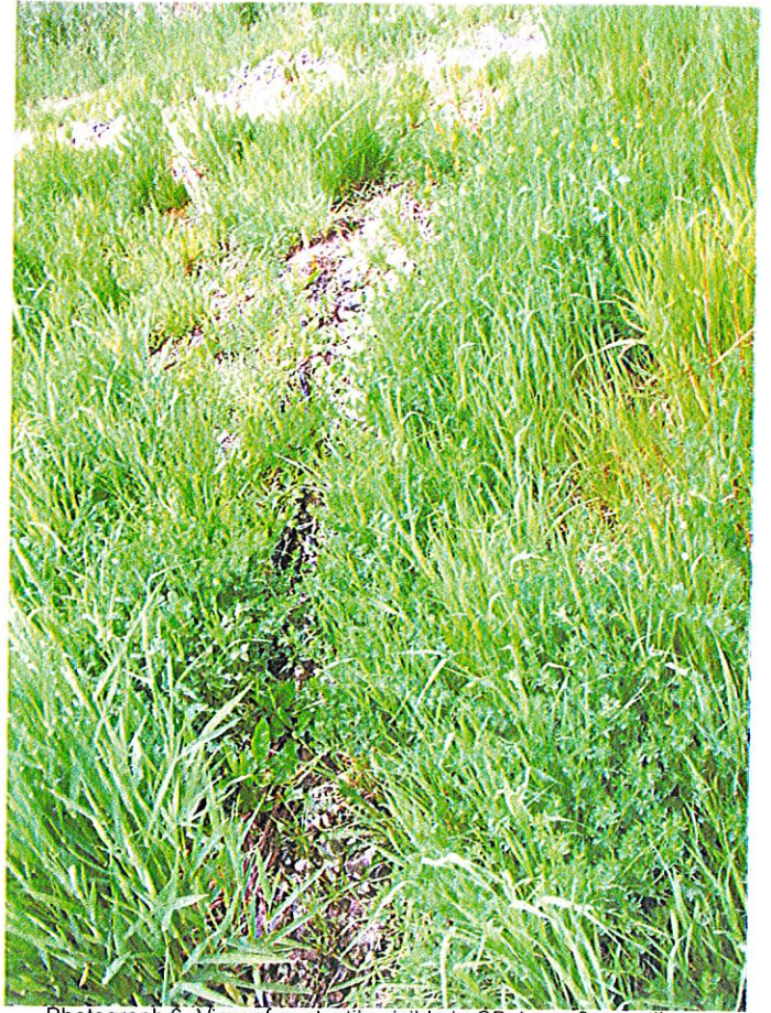
Photograph 6 -View of geotextile visible in CB-1 overflow spillway
