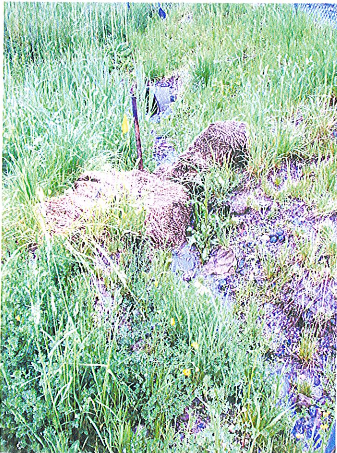
Photograph 19 - View of erosion channel near CB-3.
