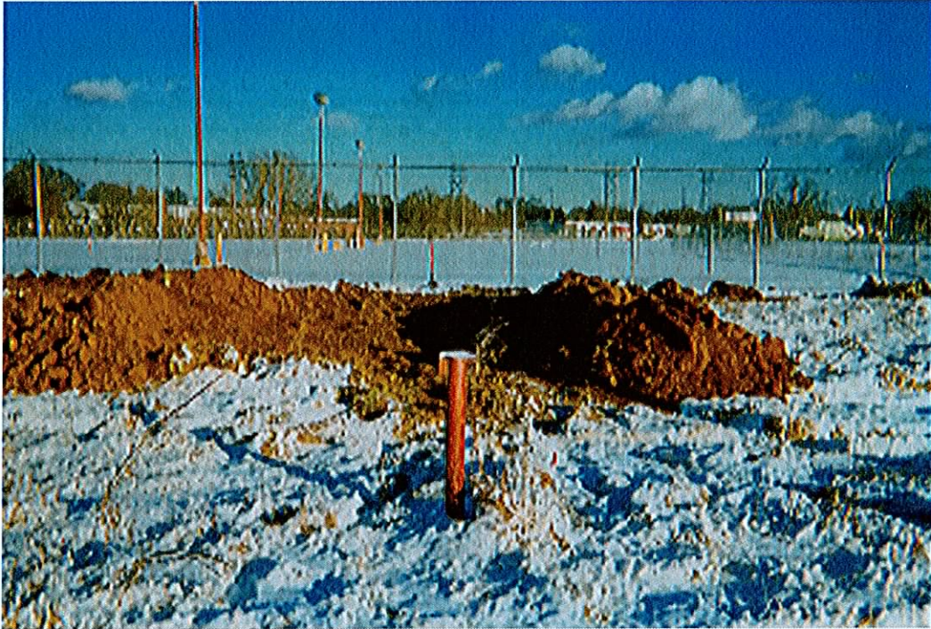
Excavation to look for historical monitoring well MW-11. Photo taken on January 16, 2007 looking east with monitoring well MW-19 in the foreground.
