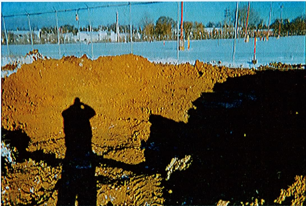
Excavation to look for historical monitoring well MW-11. Photo taken on January 16, 2007 looking northeast.
