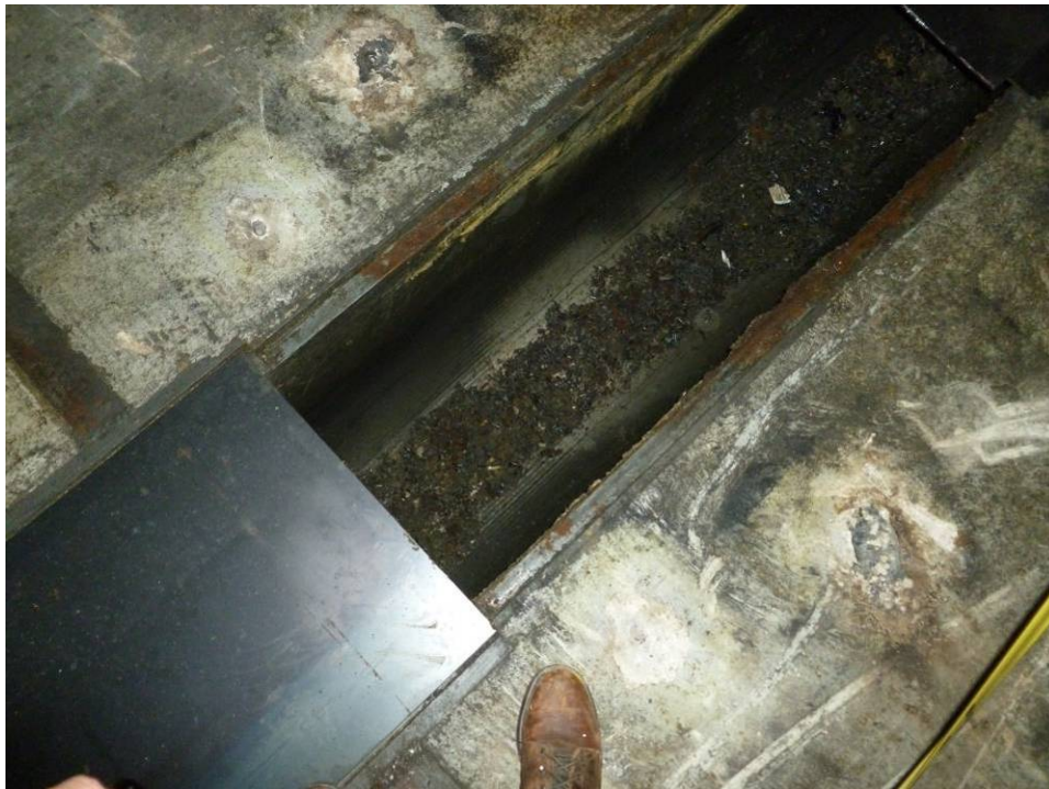
Photograph 86. (AOI-10) Flume conveyance between Equipment Pit (AOI-10) and Oil Sump (AOI-09). Flume extends approximately 22 feet from southeast area of AOI-10 to AOI-09.
