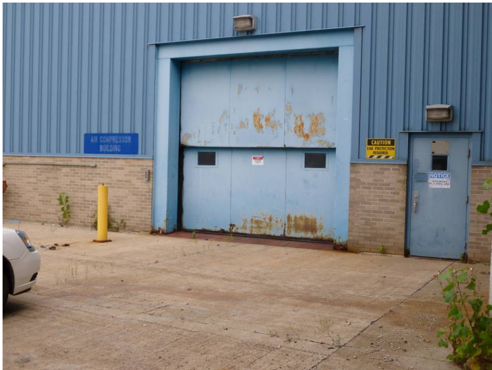
Photograph 110. (AOI-35) Entrance to Air Compressor Building. Photo taken facing east.
