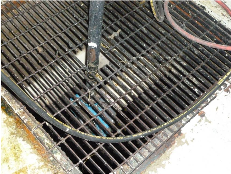
Photograph 119. (AOI-36) Oil Storage Building. Close-up of sump pit located within secondary containment area.
