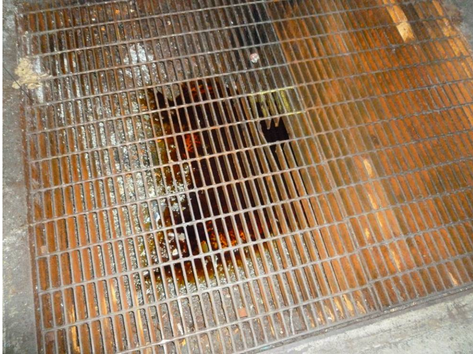
Photograph 89. (AOI-09) Oil pit, possibly associated with Oil Sump (AOI-09). Note pit contains oily material.
