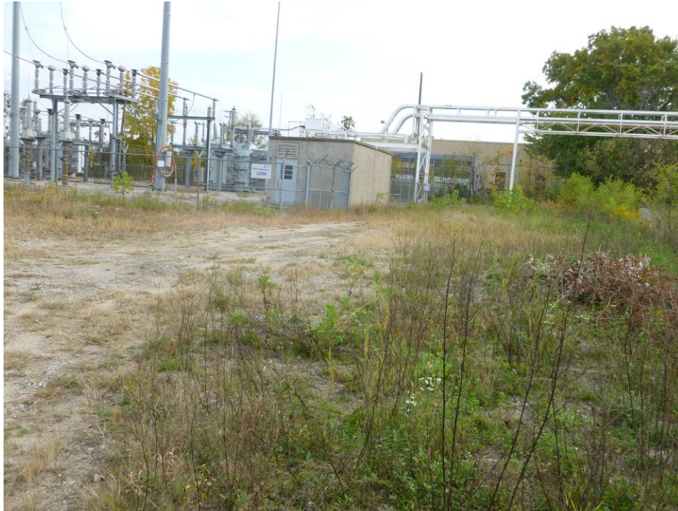
Photograph 129. (AOI-38) Detroit Edison Substation. Located east of the WWTP.
