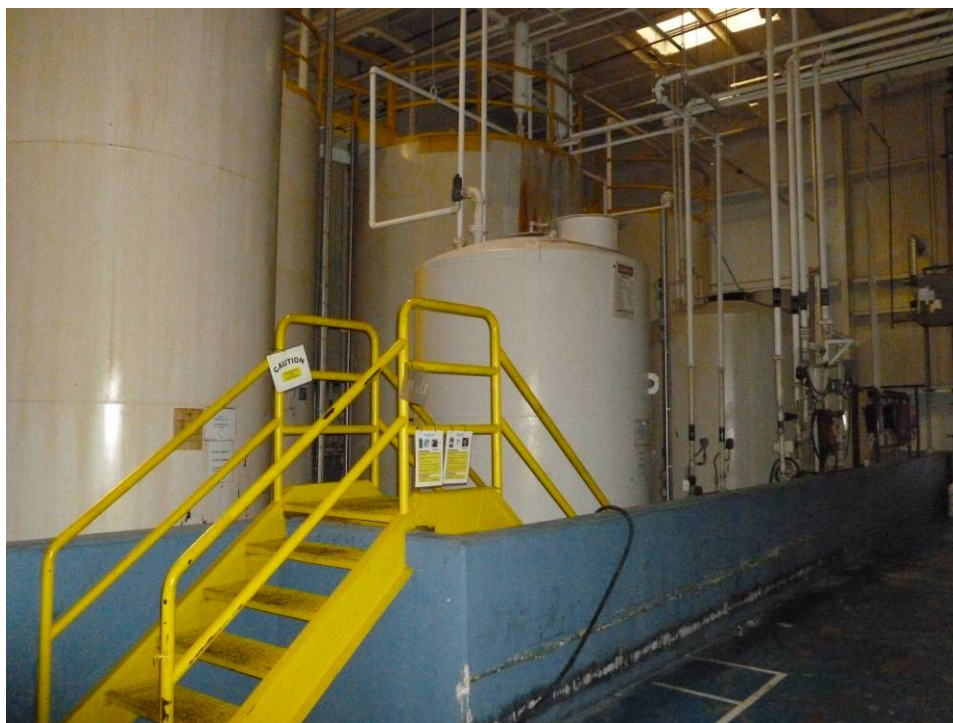
Photograph 115. (AOI-36) Oil Storage Building. Photo taken facing south. Bulk product storage of engine oil, hydraulic oil and caustic product.
