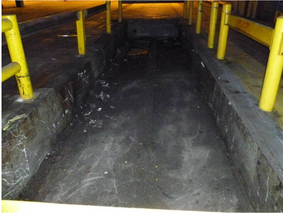
Photograph 31. (AOI-39) Equipment Pit near Columns A15/A14. Photo taken facing south.
