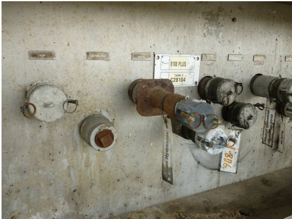
Photograph 24. (AOI-33) Fillports located within wash pad, exterior north side of WWTP.
