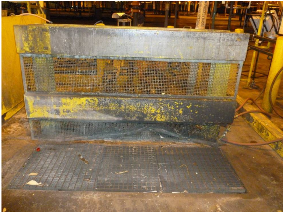
Photograph 72. (AOI-13) Wash / Dump Station.
