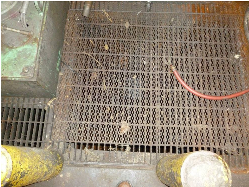
Photograph 106. (AOI-07) Dump Station near Column E14. Close-up of pit. Note oily material in pit. Depth unknown.
