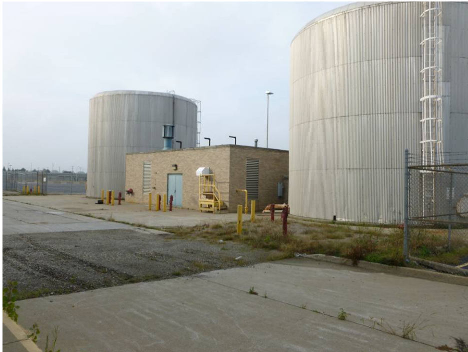
Photograph 37. (AOI-31) Fire Pump House and 2 water tanks. Photo taken facing southwest.
