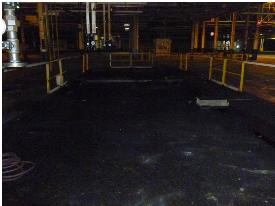
Photograph 69. (AOI-15) Equipment Pit near Columns D2/E2. Photo taken facing south.
