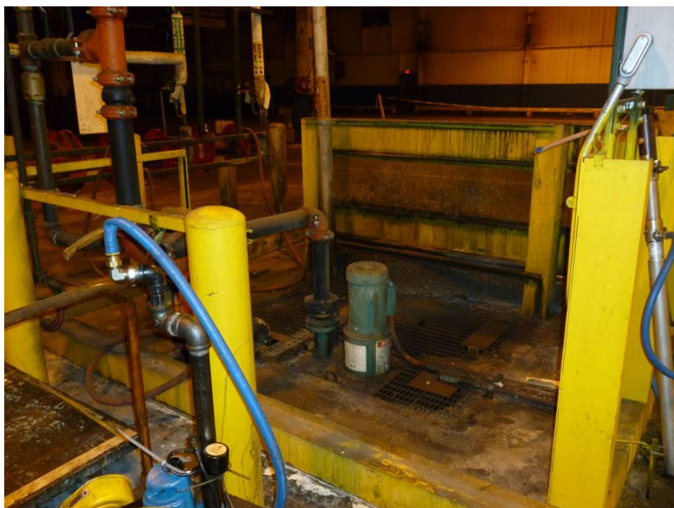
Photograph 74. (AOI-13) Wash / Dump Station. Photo taken facing west wall of Plant. Note view of Column marking "4 A 3" on west wall in background.
