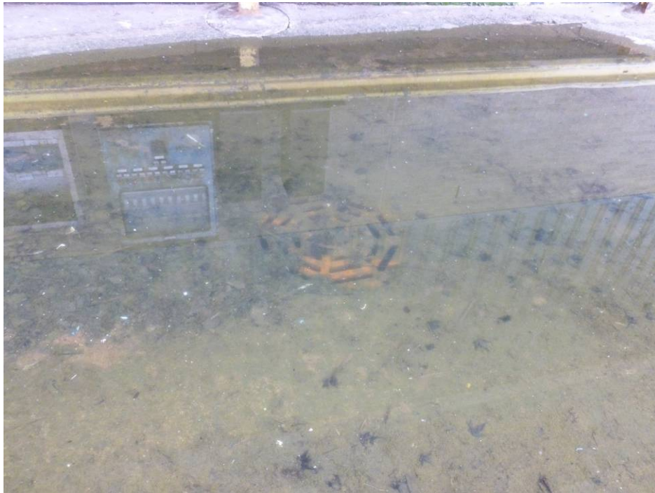
Photograph 25. (AOI-33) Drain located within wash pad, exterior north side of WWTP.
