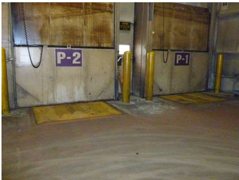
Photograph 44. (AOI-25) Purple dock area. Photo taken inside Plant, facing west.
