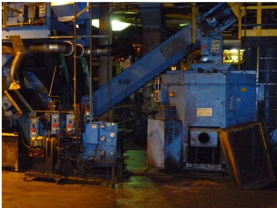
Photograph 3. (AOI-02) South Gallery, west side. Honing and chip processing equipment.
