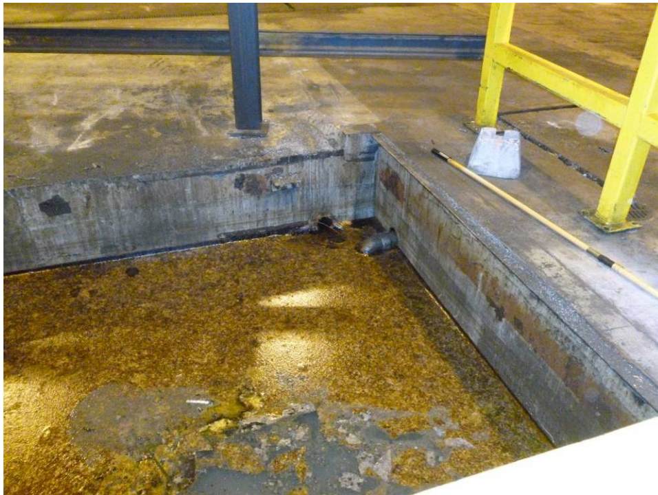
Photograph 30. (AOI-14) Equipment Pit near Columns A3/A2. Note outfalls in southeast corner.
