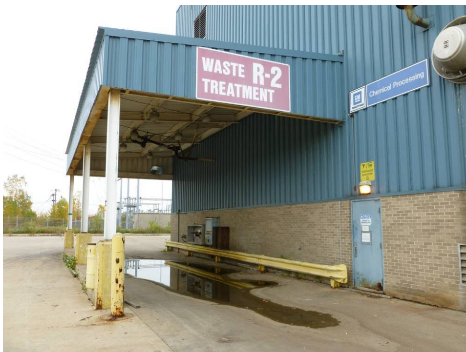
Photograph 22. (AOI-33) WWTP wash pad. Photo taken facing east.
