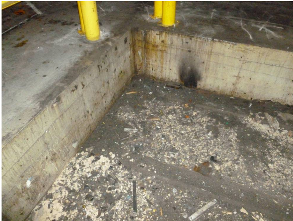
Photograph 36. (AOI-41) Equipment Pit near Columns A7/A6. Northeast area of pit.
