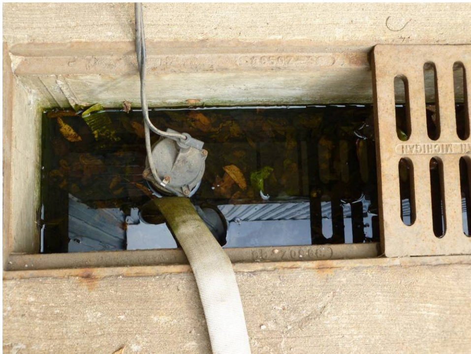
Photograph 96. (AOI-03) Blue Dock exterior. Close-up of blind trench drain. Negligible amount of sheen observed.
