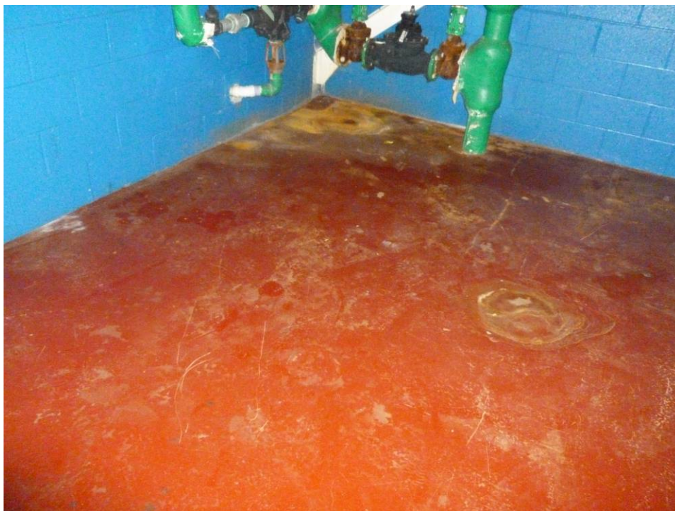
Photograph 124. (AOI-34) Less Than 90-Day Hazardous Waste Storage Area. Water control valves located in southeast corner of HW Storage Area.
