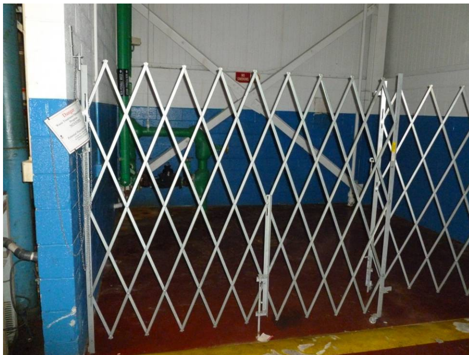
Photograph 21. (AOI-34) Less than 90-day hazardous waste storage area. Note berm at entrance, absence of floor drains.
