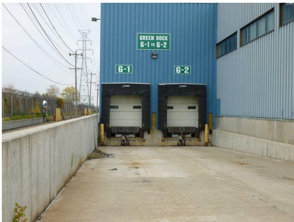
Photograph 48. (AOI-24) Green dock exterior. Photo taken facing east.
