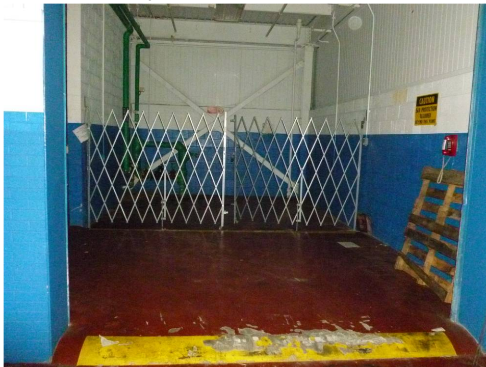
Photograph 122. (AOI-34) Less Than 90-Day Hazardous Waste Storage Area.
