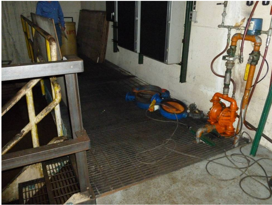
Photograph 11. (AOI-04) Sump located in southeast area of East Gallery.
