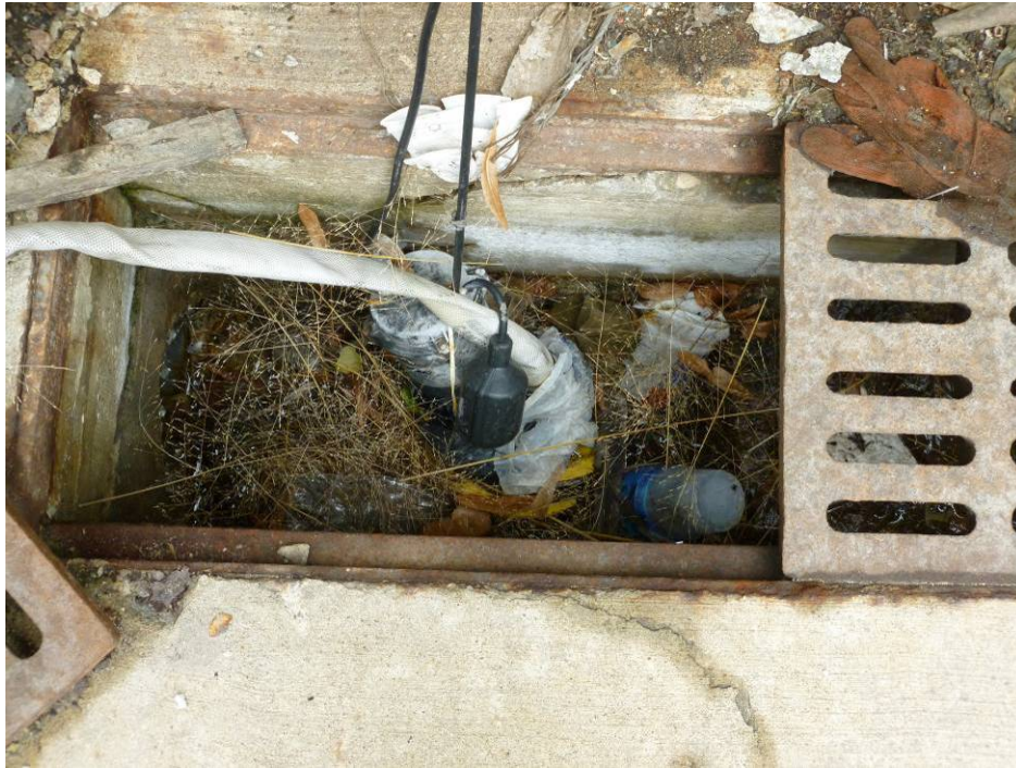
Photograph 49. (AOI-24) Green dock. Blind trench at exterior of dock.
