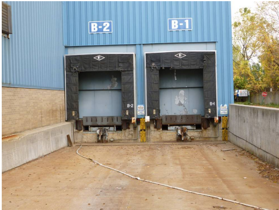
Photograph 95. (AOI-03) Blue Dock exterior. Photo taken facing west. No evidence of staining observed.
