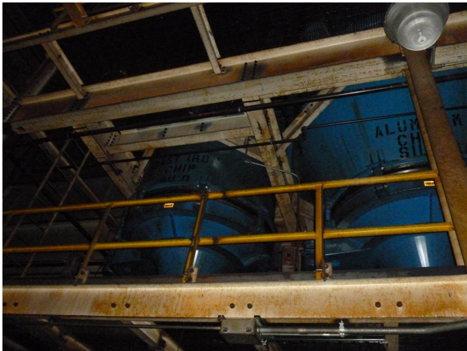
Photograph 104. (AOI-01) Truck Bay. Overhead iron and aluminum chip silos.
