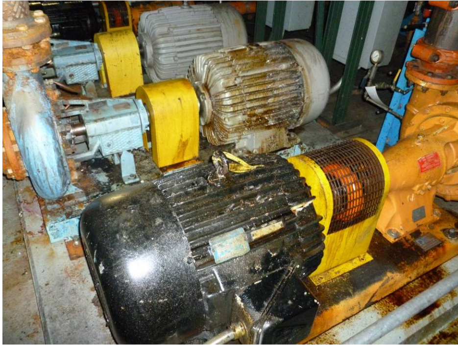
Photograph 9. (AOI-04) East Gallery. Oily residue on rod machining equipment.
