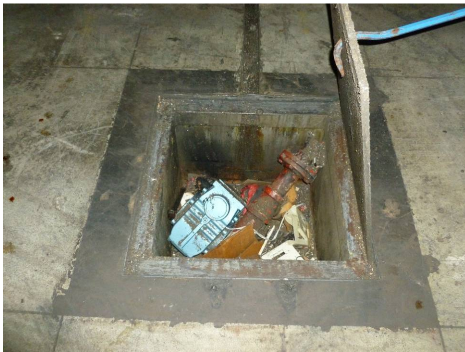
Photograph 33. (AOI-40) Sump near Columns A11/A12, near west wall of Plant. Steel construction. Contains miscellaneous debris, possibly associated with plant decommissioning.
