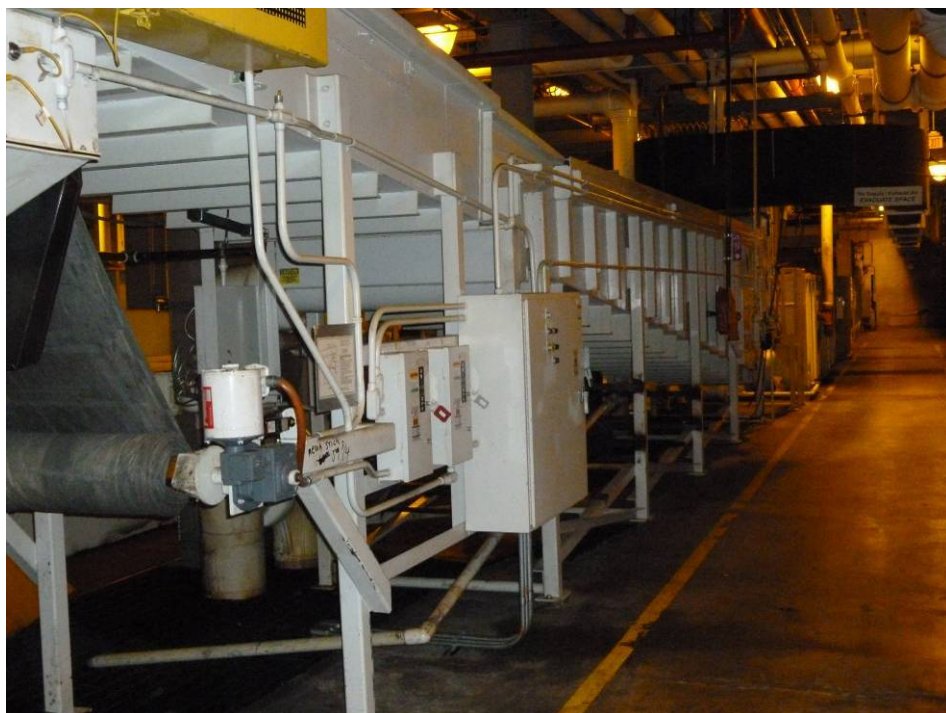
Photograph 4. (AOI-02) South Gallery, east side. Block grinding equipment.
