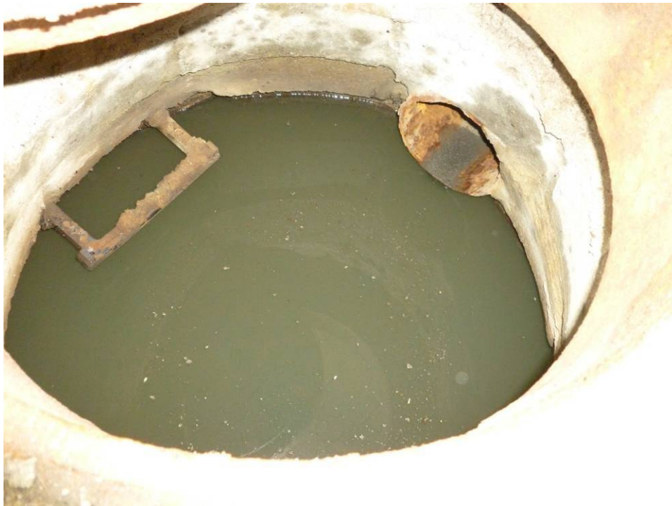
Photograph 26. (AOI-33) Drain located within wash pad. Removed cover to take photo.
