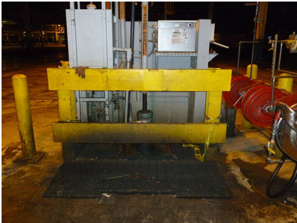
Photograph 92. (AOI-05) Clean / Dump Station near Column L14. Note dark staining / oily residue around station.
