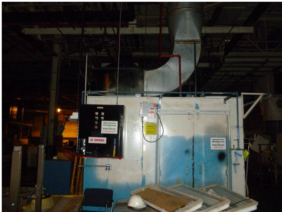
Photograph 28. (AOI-26) Paint booth near Columns D20/D21. Exterior view of paint booth.
