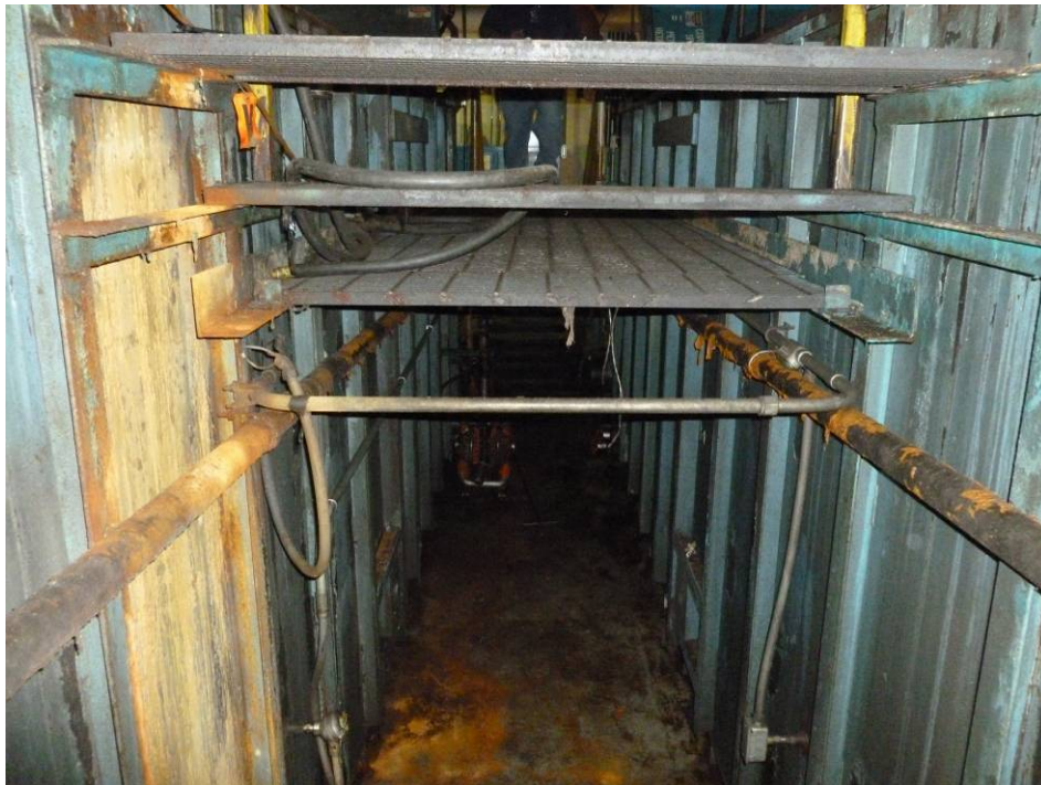
Photograph 10. (AOI-04) East Gallery. Sub-basement.
