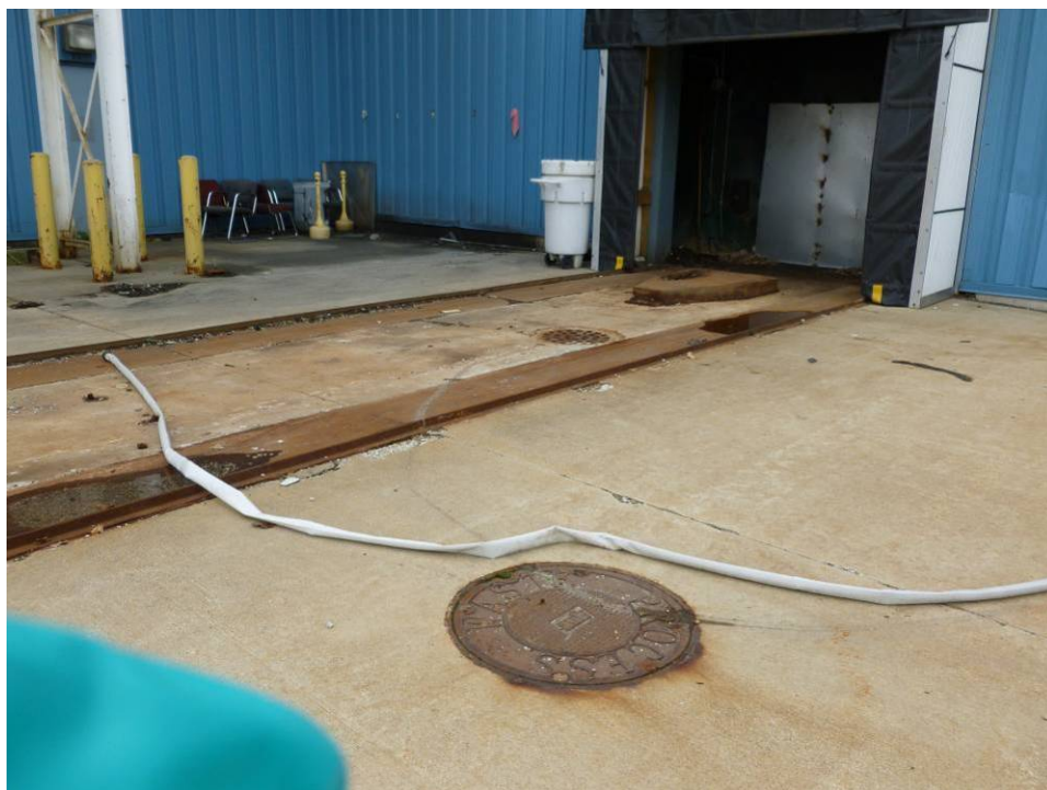
Photograph 63. (AOI-19) Trash compactor area exterior. Note drain located between metal rails and process waste manhole in foreground.
