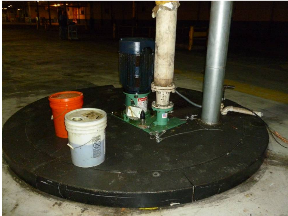
Photograph 87. (AOI-09) Oil Sump near Columns L8/M8. Sump is approximately 5 feet in diameter.
