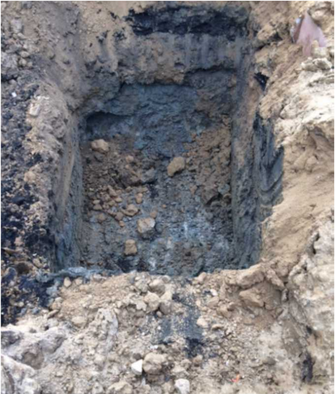
Excavation B facing East sidewall
