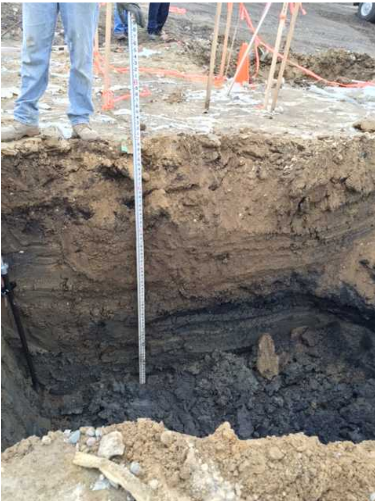
Excavation A facing North sidewall
