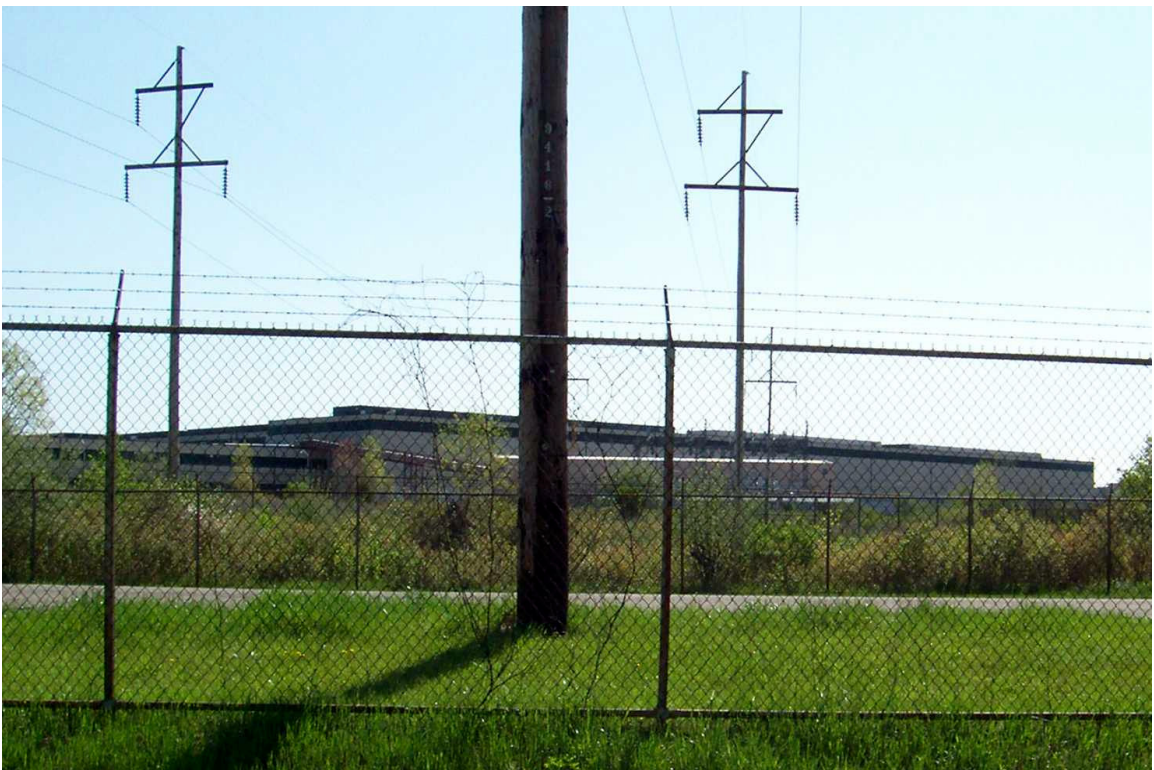
West side of Grand Blanc MFD facility
