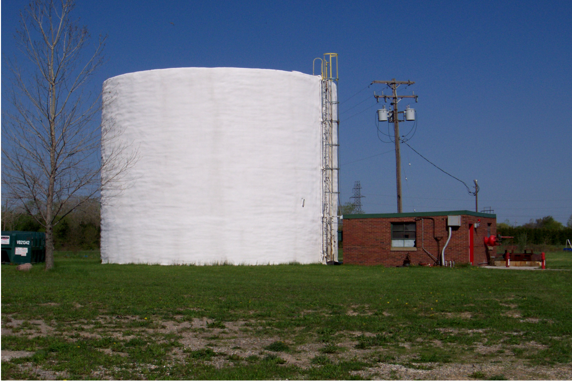
Pump House and water tank in Area 2 looking northwest
