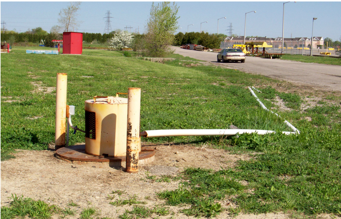
Crock Sump in Area 2 looking northwest
