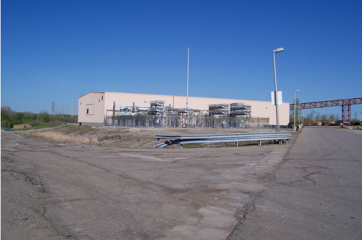
Substation in Area 2 looking northwest
