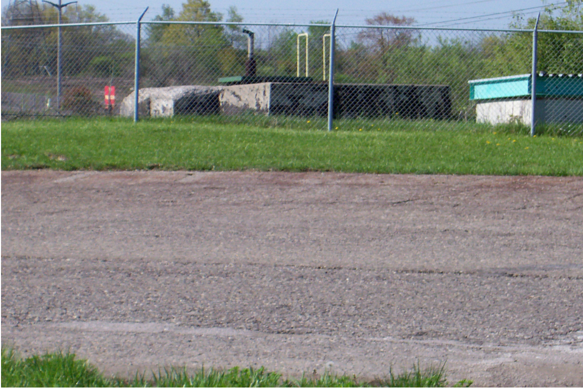
Well #5 and AST vault area (which is former UST area also) in Area 2 looking southwest
