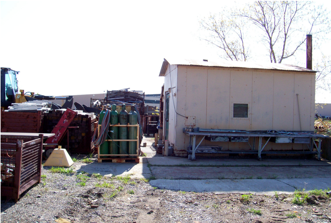
Die storage area shed looking toward the east
