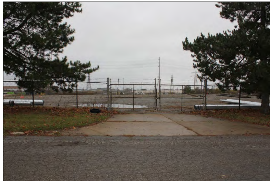
Photo 58: St Clair Street south entrance to project area, looking east.
