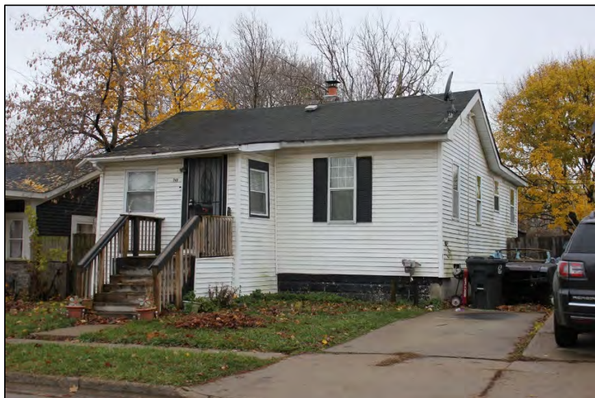
Photo 27: 743 Portland Street, looking southwest. Built 1920.
