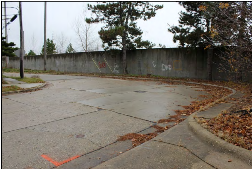
Photo 31: Ribbed concrete wall between south side of central project area and Owen Street, looking northwest.
