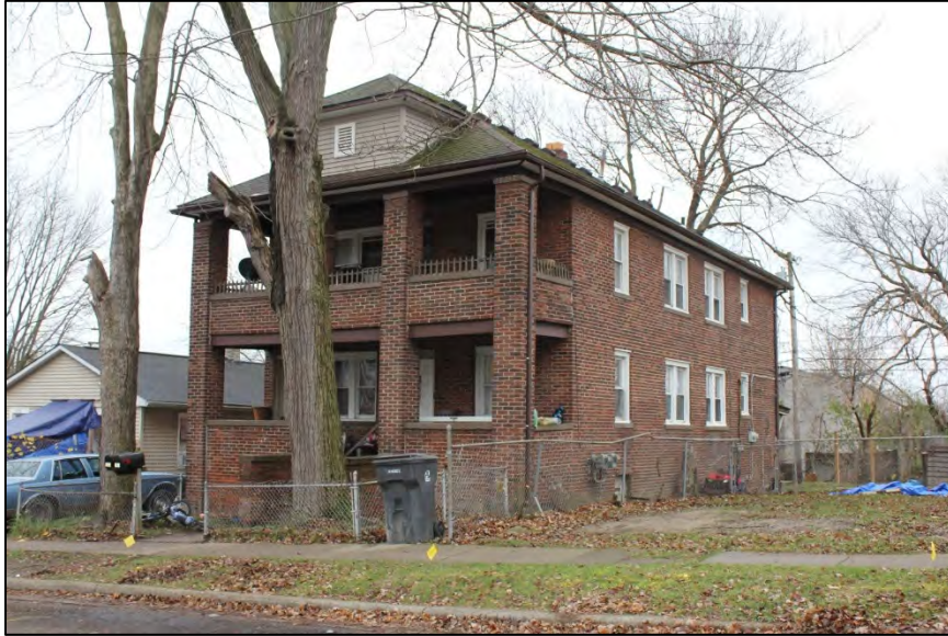
Photo 53: 763-765-767 St Clair Street, looking southwest. Built 1920.
