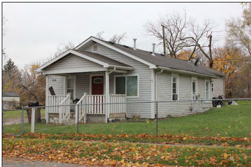
Photo 39: 755 Wing Street, looking southwest. Built 1920.
