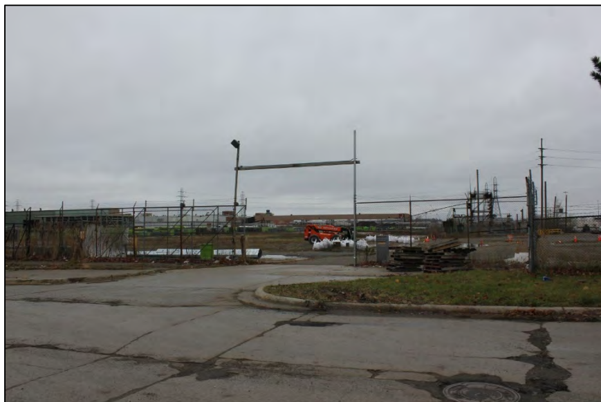
Photo 59: St Clair Street north entrance to project area, looking east.
