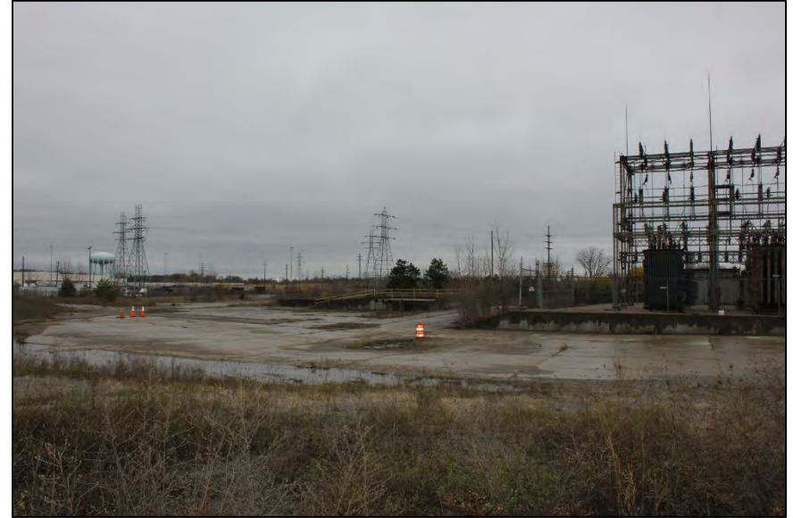
Photo 14: Looking southeast from west-central project area.
