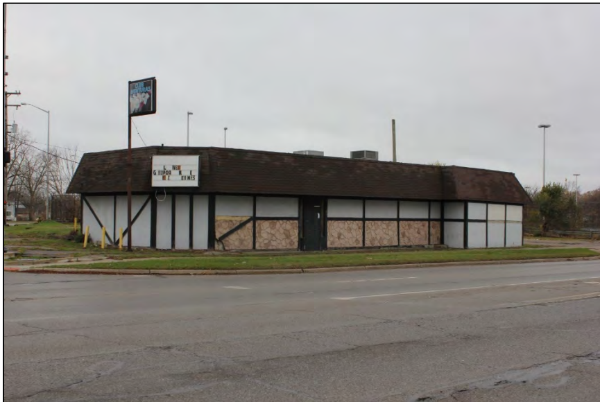
Photo 63: 867 Baldwin Avenue, looking northwest. Built c.1965.
