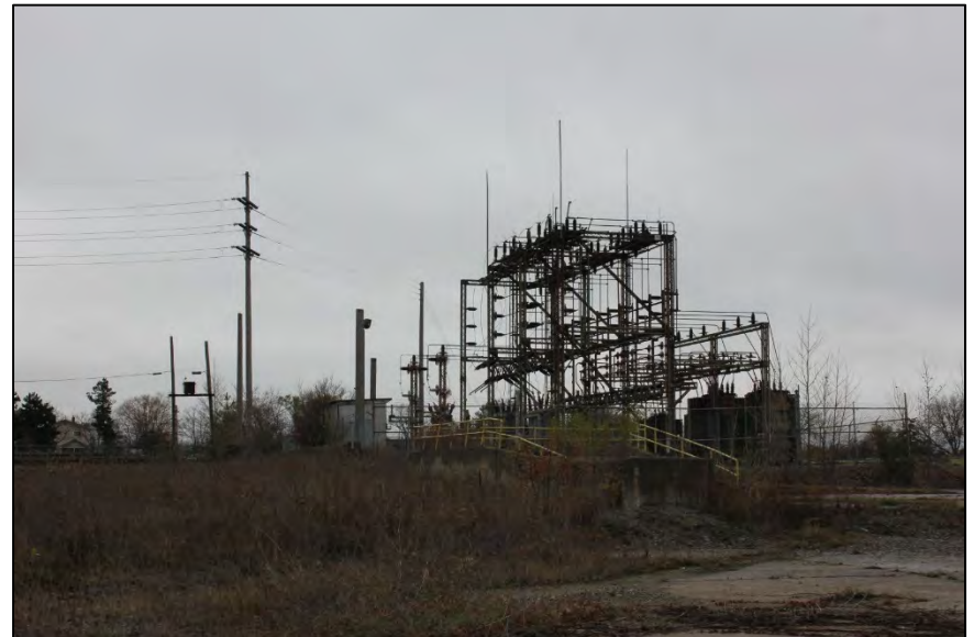
Photo 8: Looking west from east-central project area.
