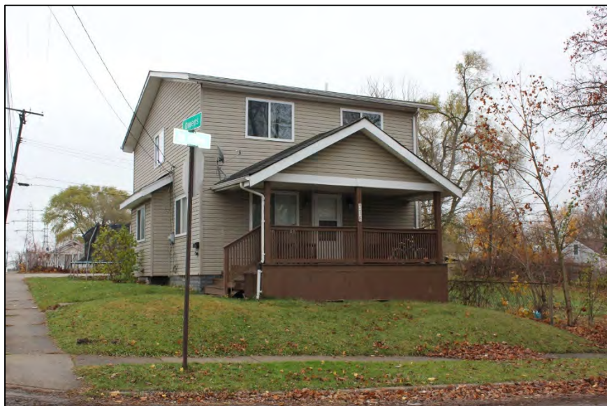
Photo 51: 776 St Clair Street, looking southeast. Built 1920.
