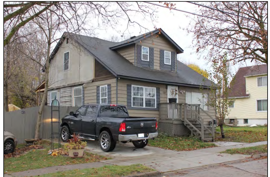
Photo 24: 727 Portland Street, looking northwest. Built 1920.
