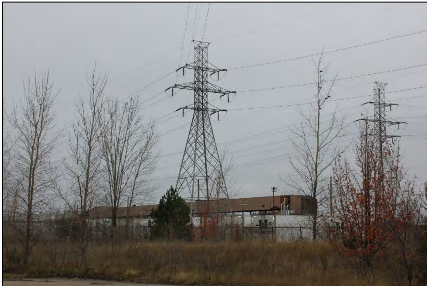
Photo 7: Looking northeast from east-central project area.
