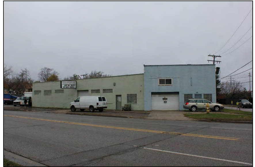
Photo 22: 105 E Montcalm Street, looking north.
