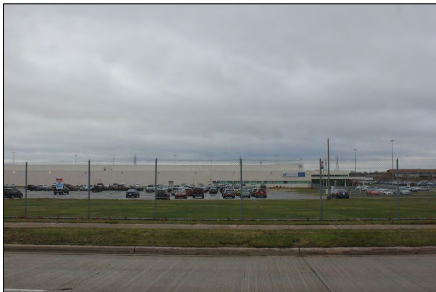
Photo 65: 711 N Glenwood Avenue, looking west. Built c.2008.
