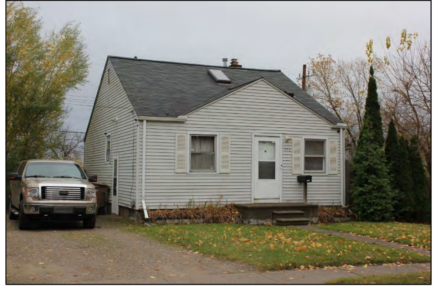
Photo 34: 772 Wing Street, looking southeast. Built 1951.
