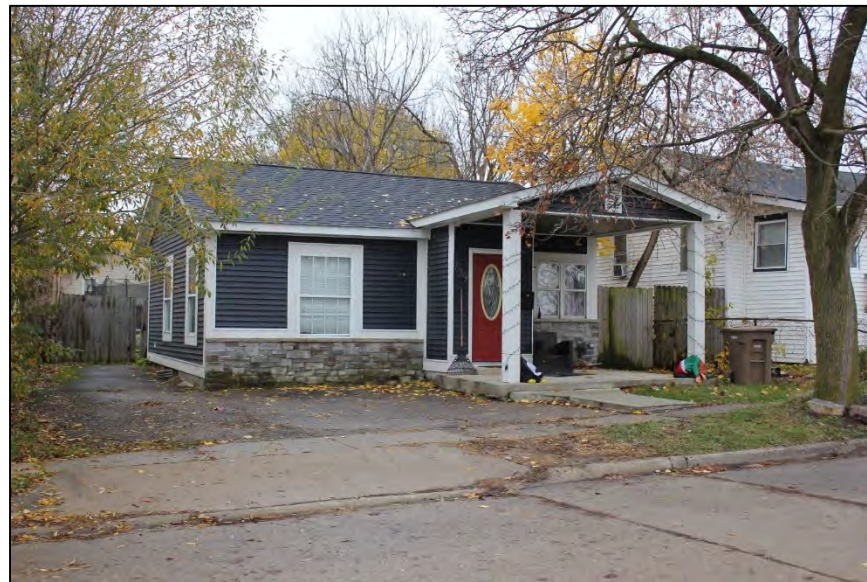
Photo 26: 739 Portland Street, looking northwest. Built 1920.
