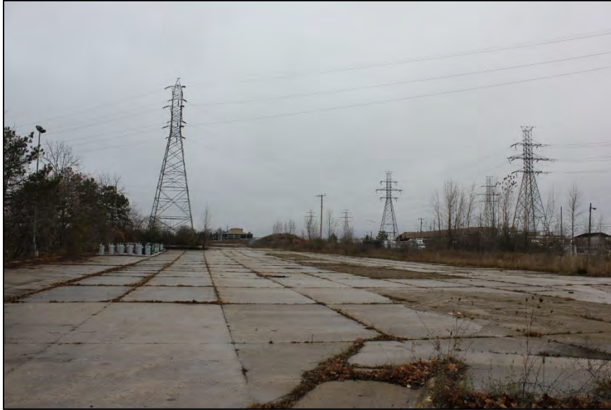
Photo 1: View over east side of project area, looking north.
