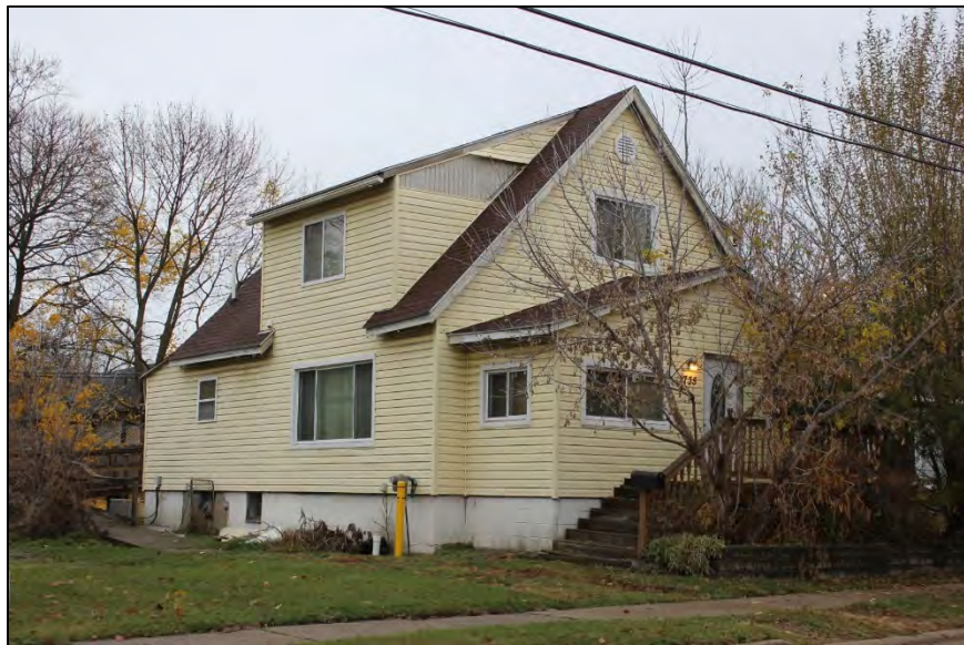
Photo 25: 735 Portland Street, looking northwest. Built 1920.
