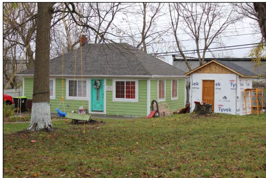
Photo 52: 771 St Clair Street, looking southwest. Built 1920.
