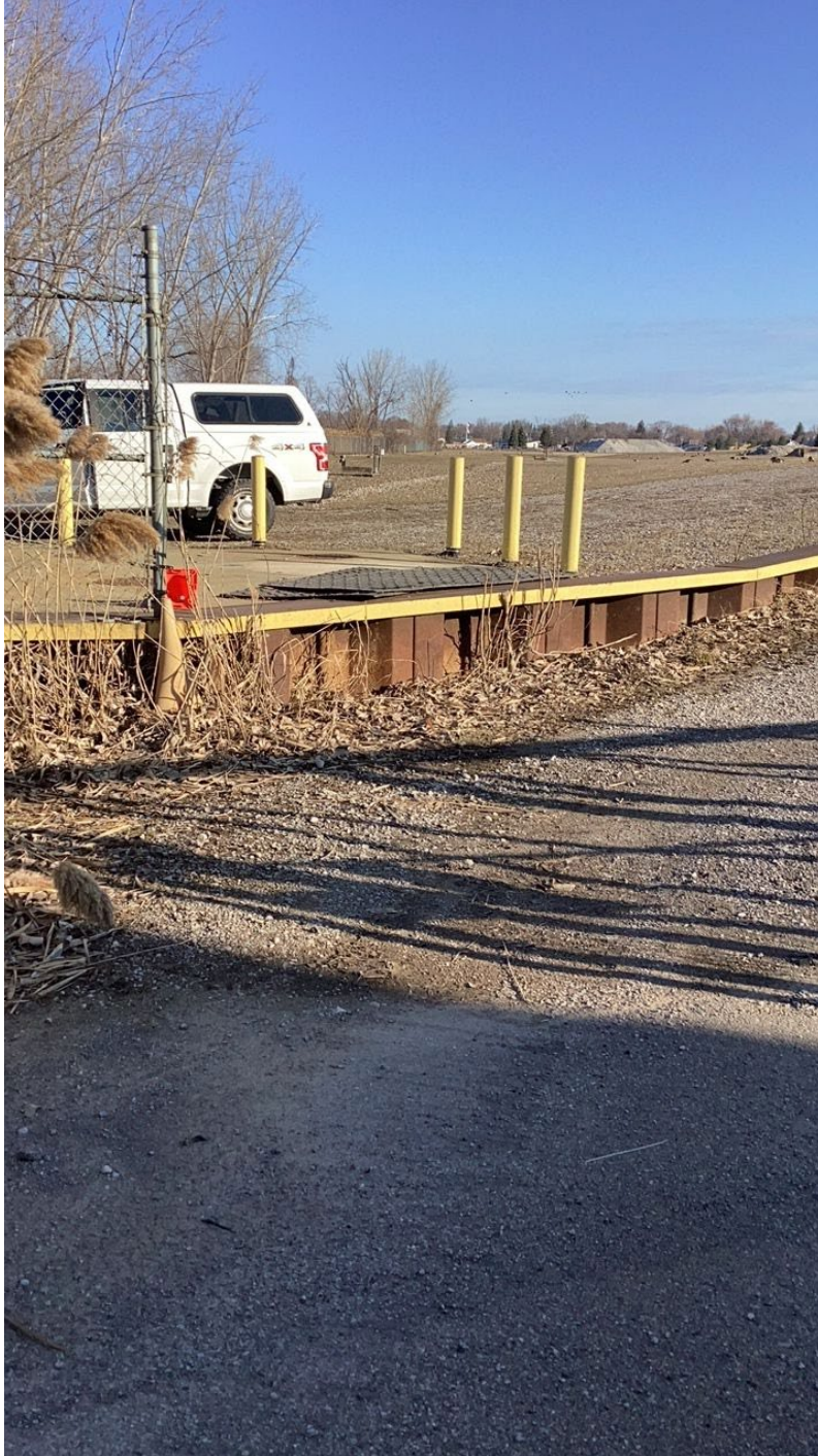
Photo 1 – Sheet Pile Wall At Entrance
