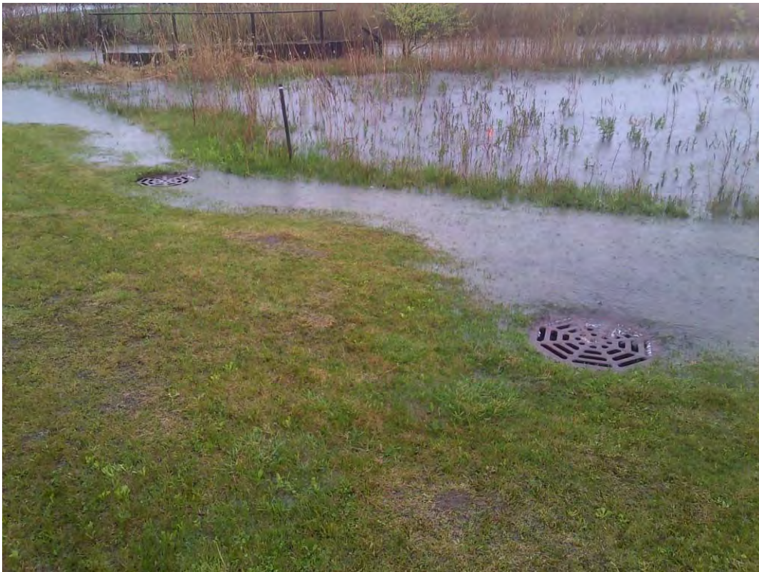
PHOTO 8: NORTH DITCH – OUTFALL 22 DISCHARGE LOCATIONS (5/2014)
