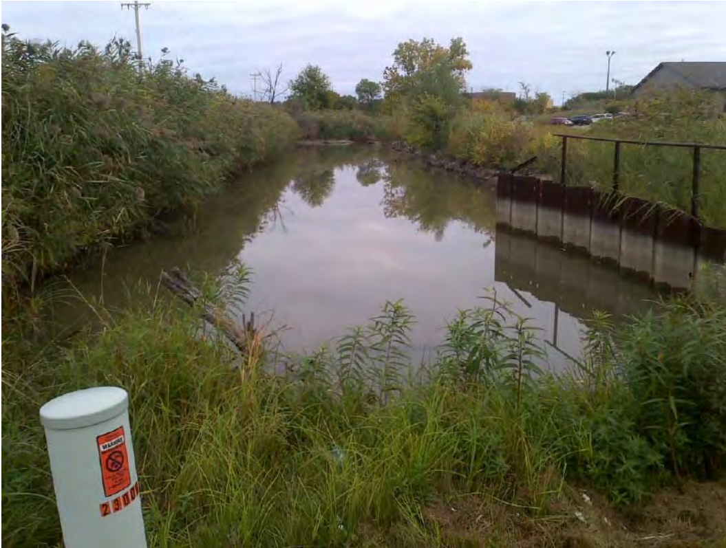
PHOTO 7: NORTH DITCH - LOOKING NORTHEAST FROM DRIVEWAY (9/2013)
