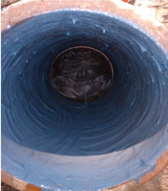
Sandbags installed inside pipe to block flow while bonding agent cures.
