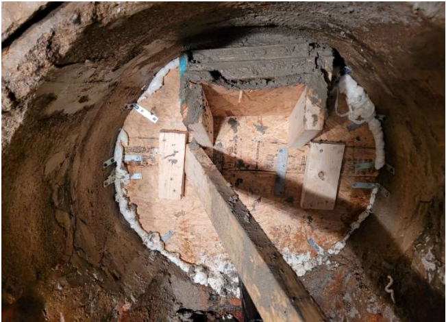
Example of sealed front form exterior with supports.
