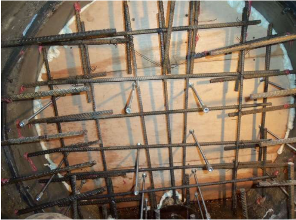
Example of sealed back form and rebar supports installed.
