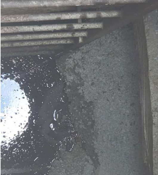
Manhole with bentonite prior to pour
