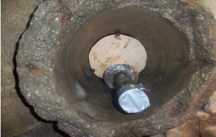
Example of plug on 24" line with flow through pipe still in place
