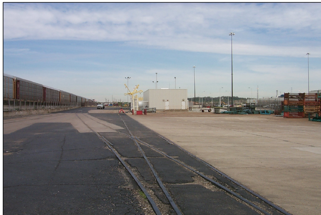
VIEW FACING NORTH, FROM DRIVEWAY WEST OF MORaine ENGINE PLANT. MORaine ENGINE TANK FARM PUMP HOUSE IN THE BACKGROUND.
