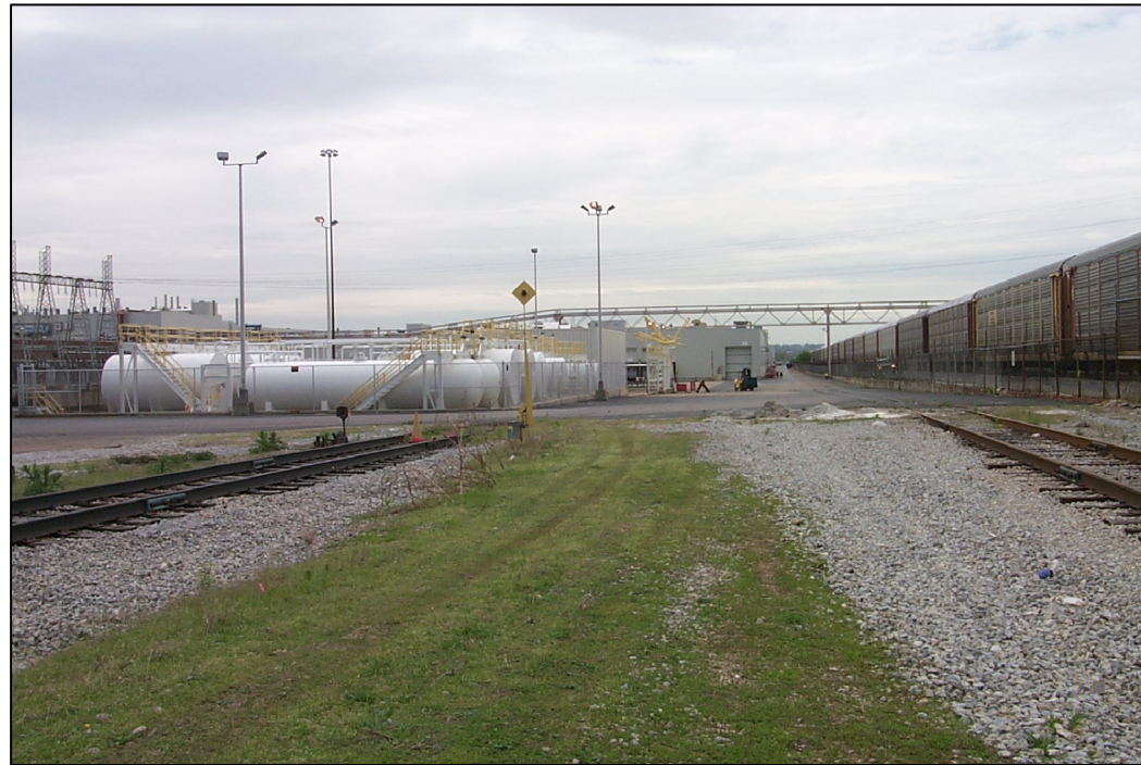
VIEW FACING SOUTH, WITH MORaine ENGINE TANK FARM IN THE MIDDLE AND MORaine ENGINE PLANT IN THE BACKGROUND.
