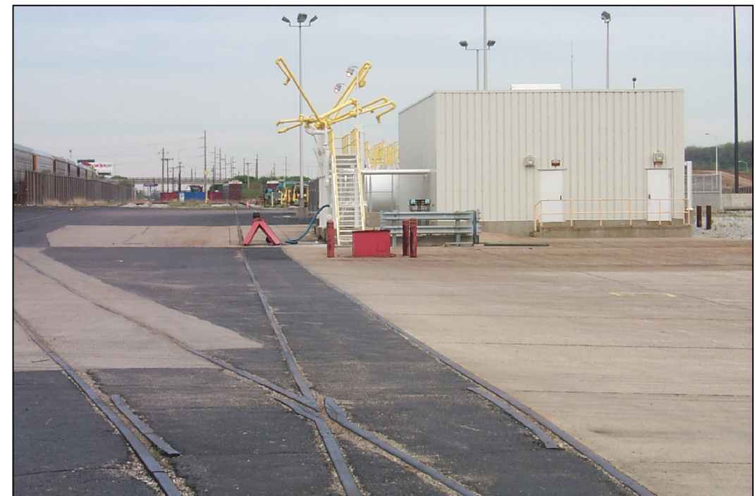
VIEW FACING NORTH, OF THE MORaine ENGINE TANK FARM PUMP HOUSE.
