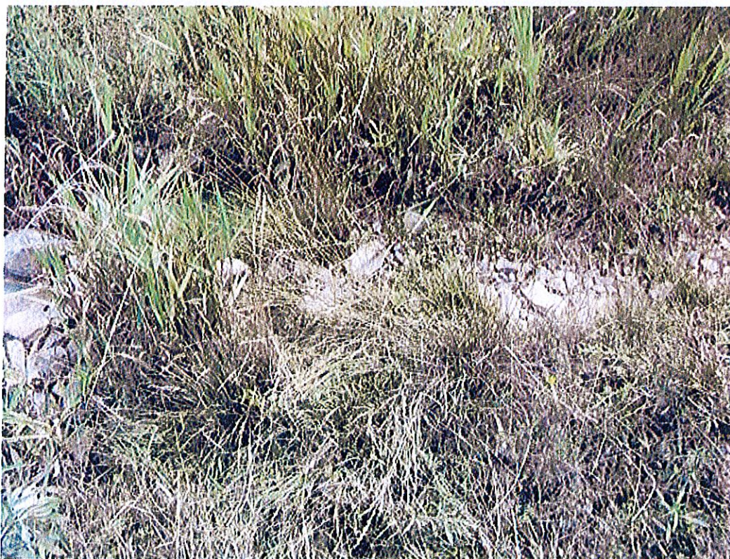
Photograph 8: Erosion in CB-1 overflow spillway along access road.
