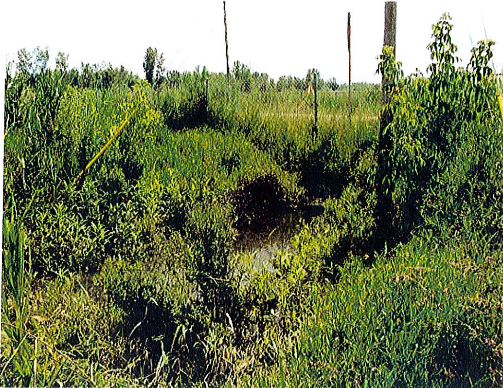
Photograph 5: Stagnant water in CB-1 indicates clogging.
