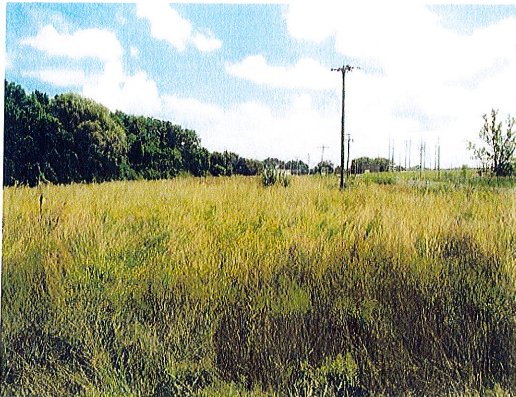
Paragraph 19: View looking east near CB-3 overflow spillway.
