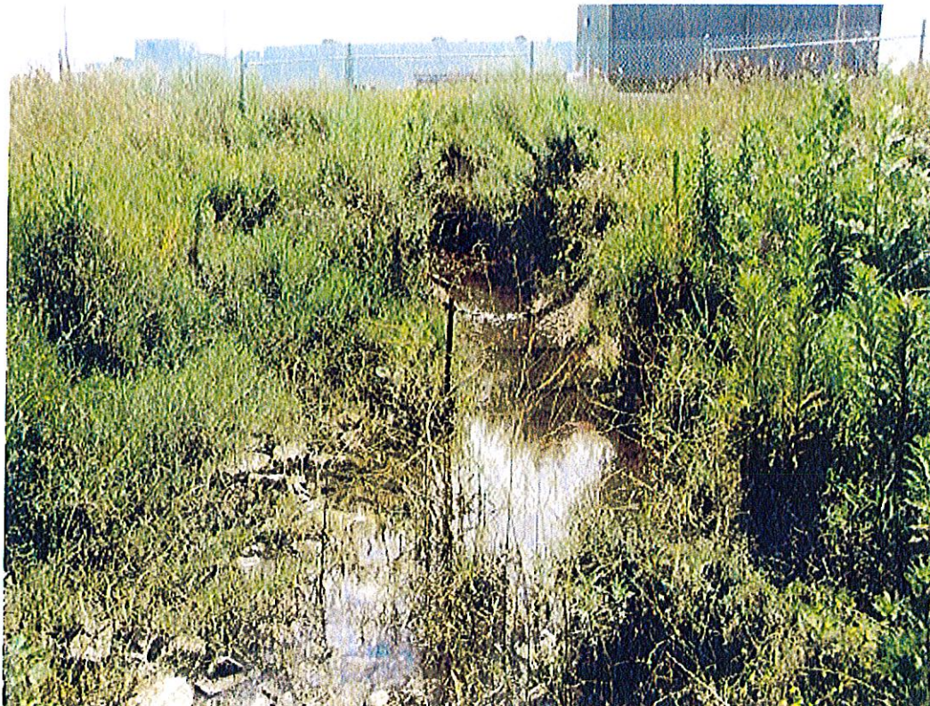
Photograph 24: Overflow spillway CB-4.
