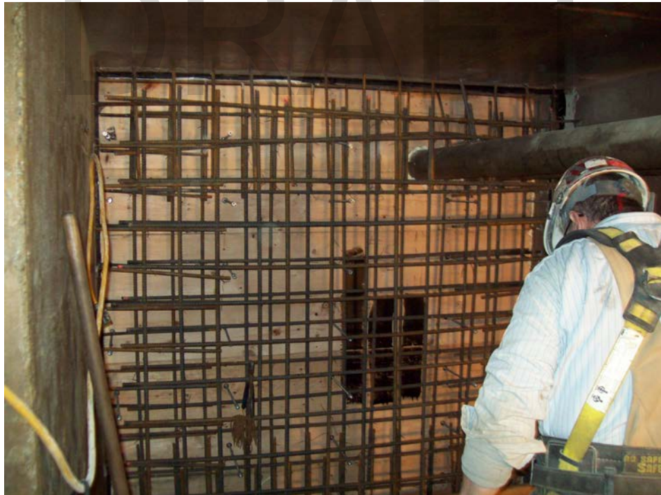
Photo 22: Sacrificial Form Junction Chamber No.1
