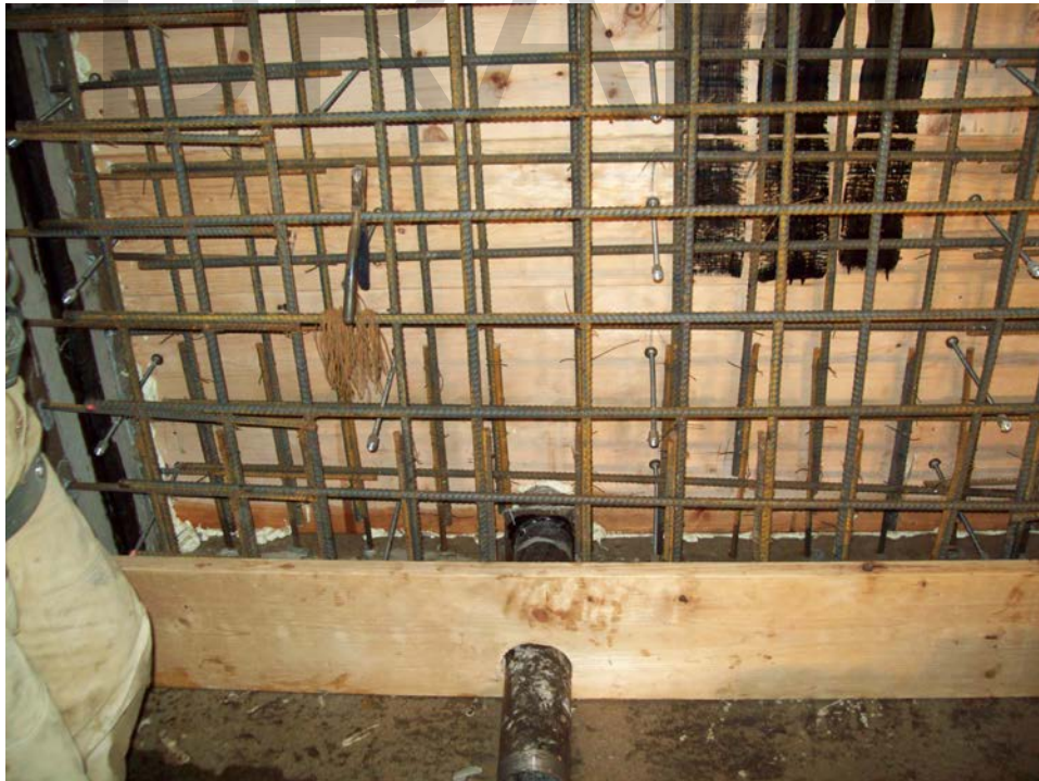
Photo 20: Sacrificial Form Junction Chamber No.1
