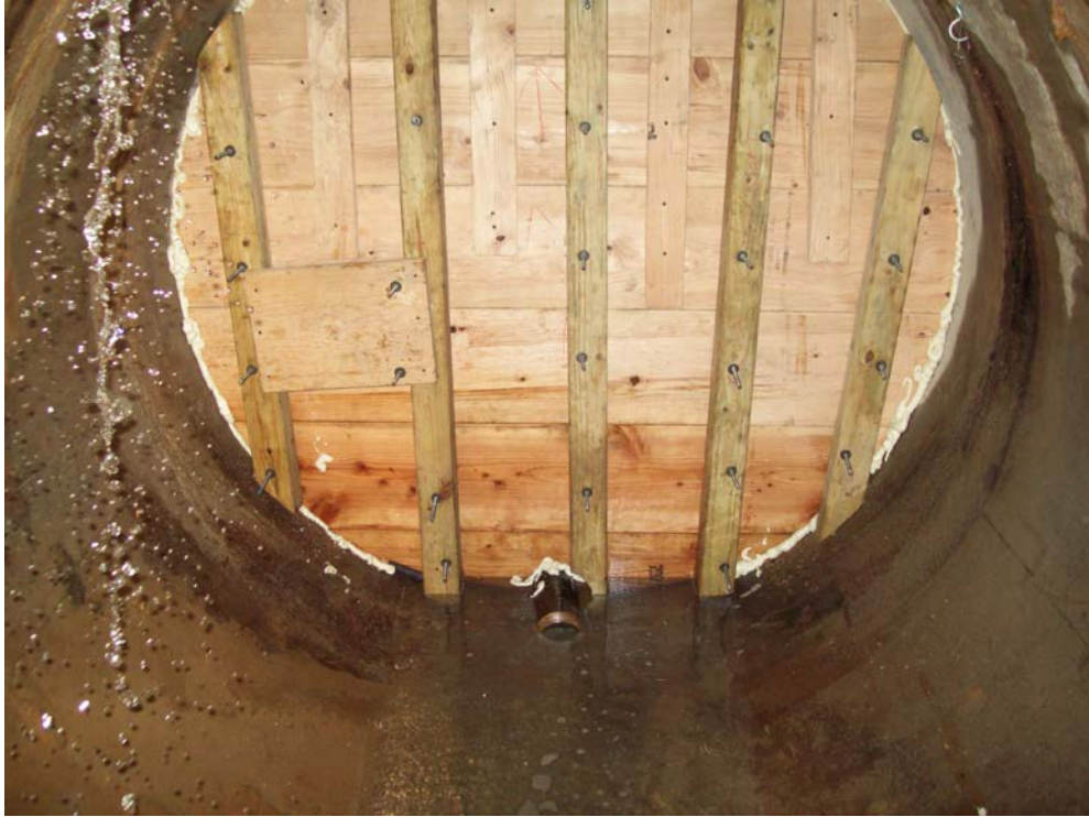
Photo 17: North side of the bulkhead form at ST8A
