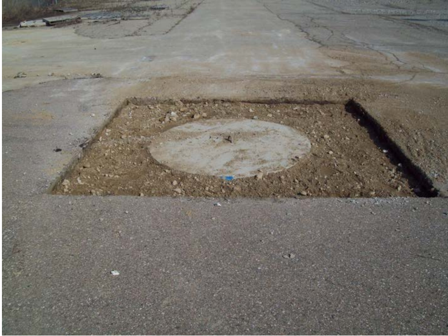
Photo 1: Concrete cookie placed on storm sewer inlet
