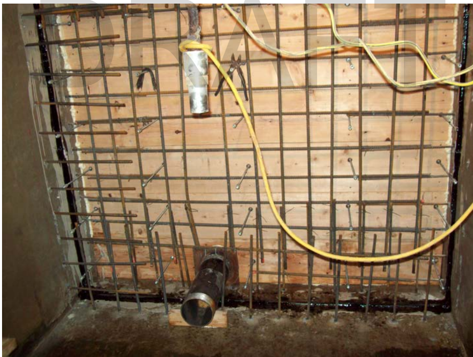
Photo 24: Sacrificial side of form junction chamber No. 2
