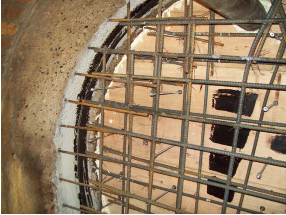
Photo 9: Sacrificial form built in storm sewer No. 4
