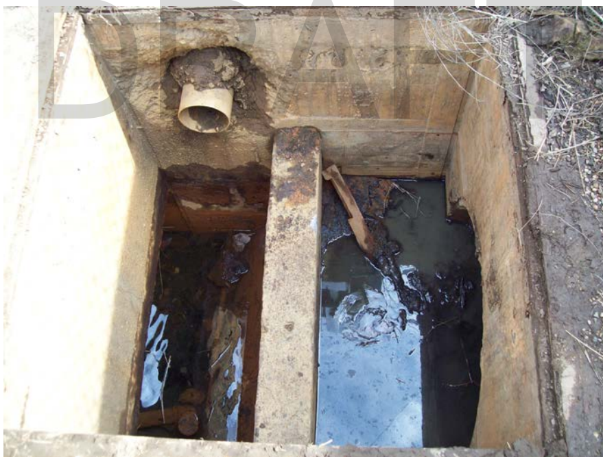
Photo 2: South east side of pump station vault prior to plugs
