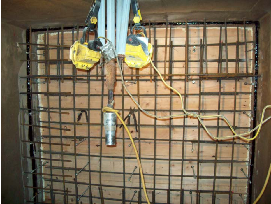
Photo 25: Sacrificial side of form junction chamber No. 2
