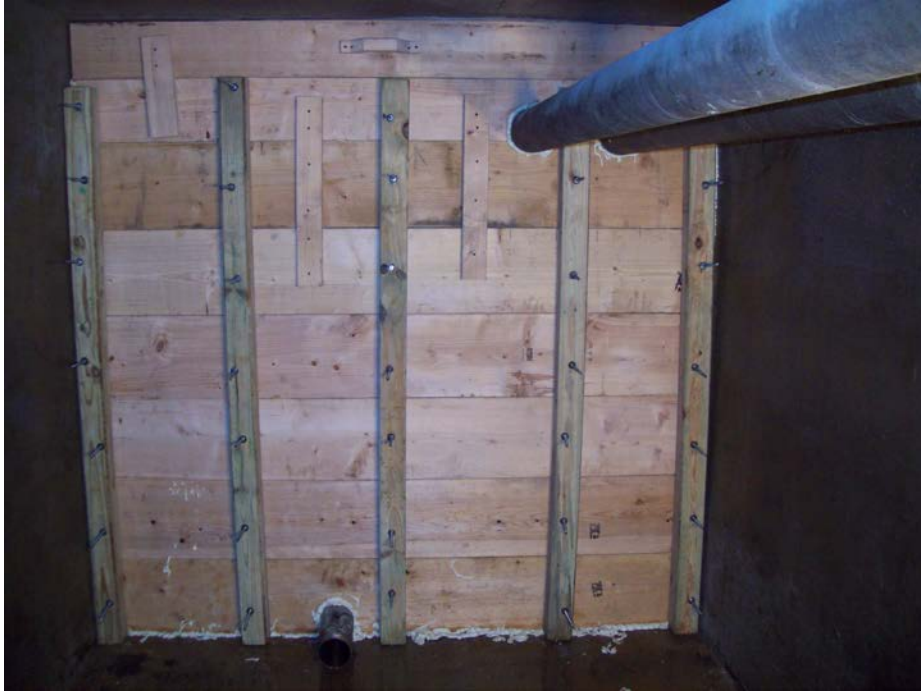
Photo 23: Upstream side of form in Junction Chamber No.1
