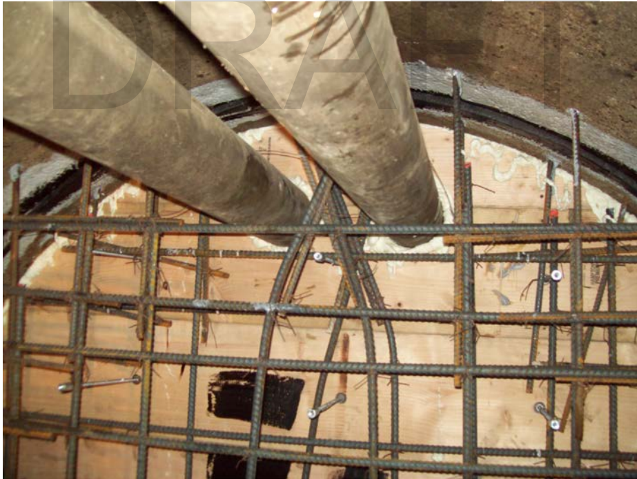
Photo 10: Sacrificial form built in storm sewer No. 4
