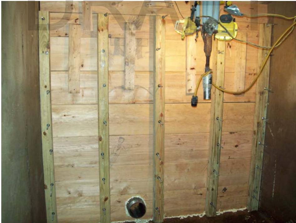
Photo 26: Completed form junction chamber No. 2
