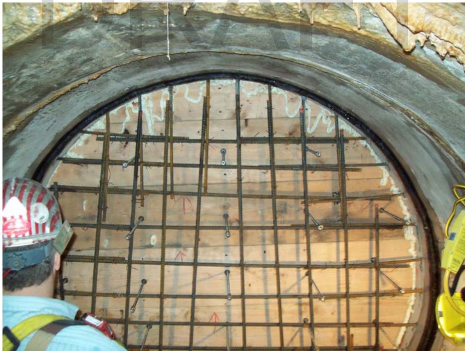
Photo 14: Downstream section of form inside ST8A
