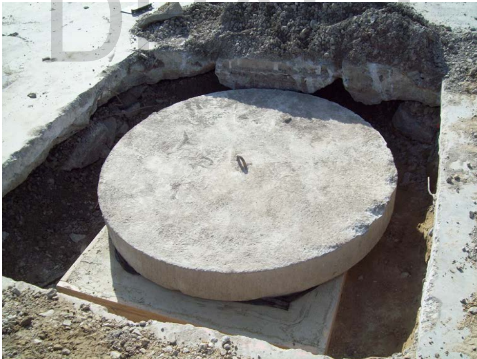
Photo 12: Concrete cookie placed on rectangular shaped storm inlet.
