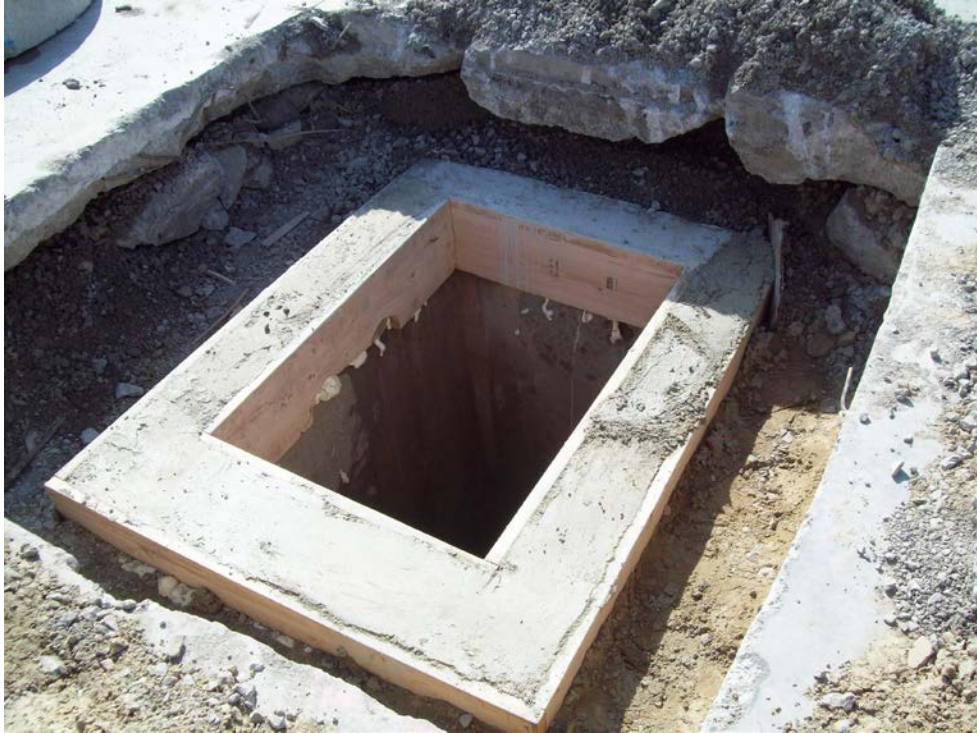
Photo 11: Rectangular shaped storm inlet with concrete base pored.
