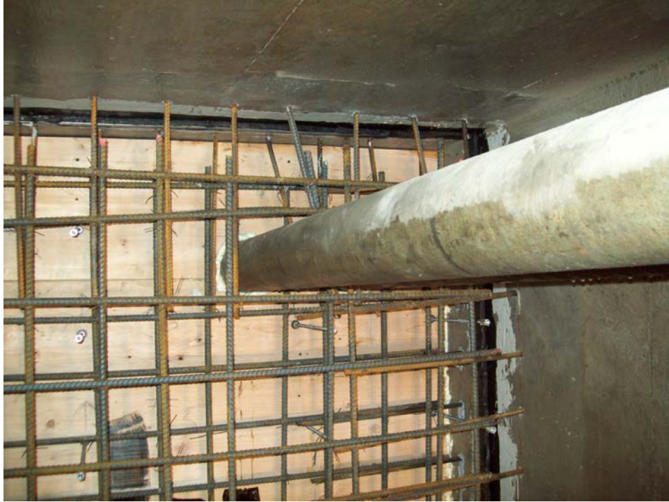
Photo 21: Sacrificial Form Junction Chamber No.1
