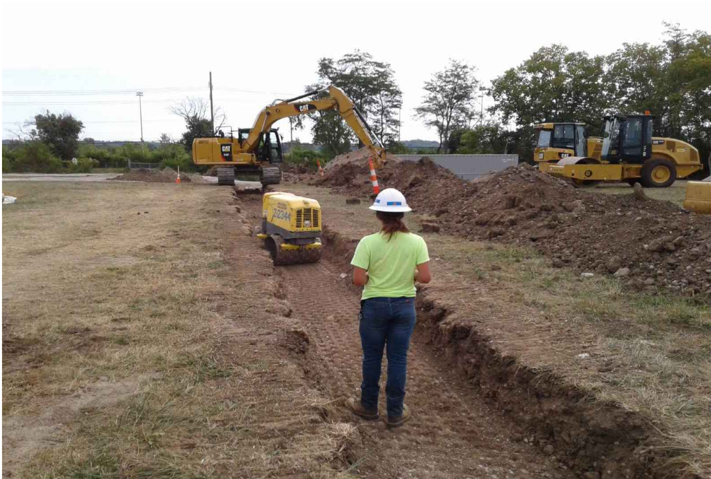
View of compaction site, compaction in progress
