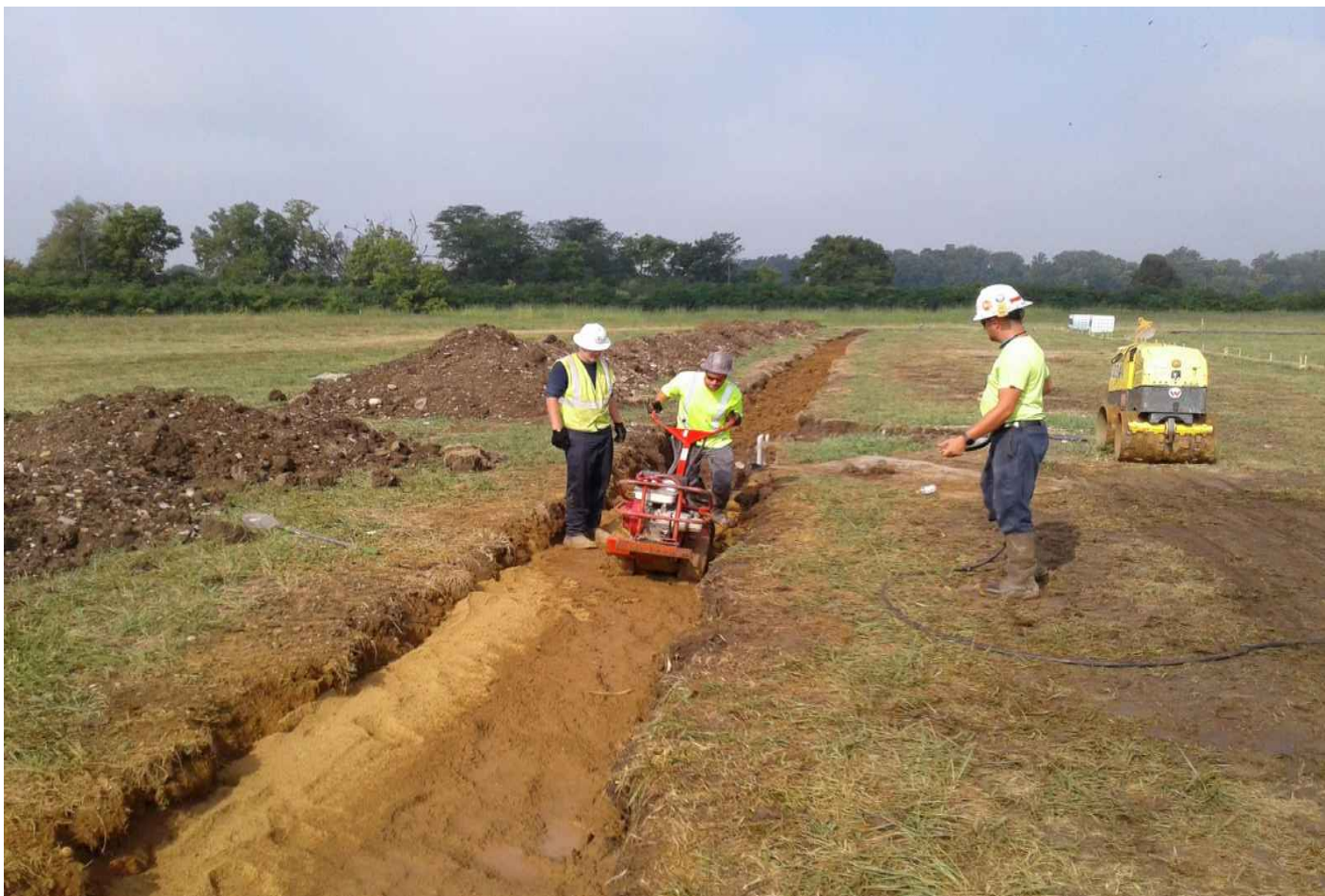
View of compaction site, watering and tilling in progress
