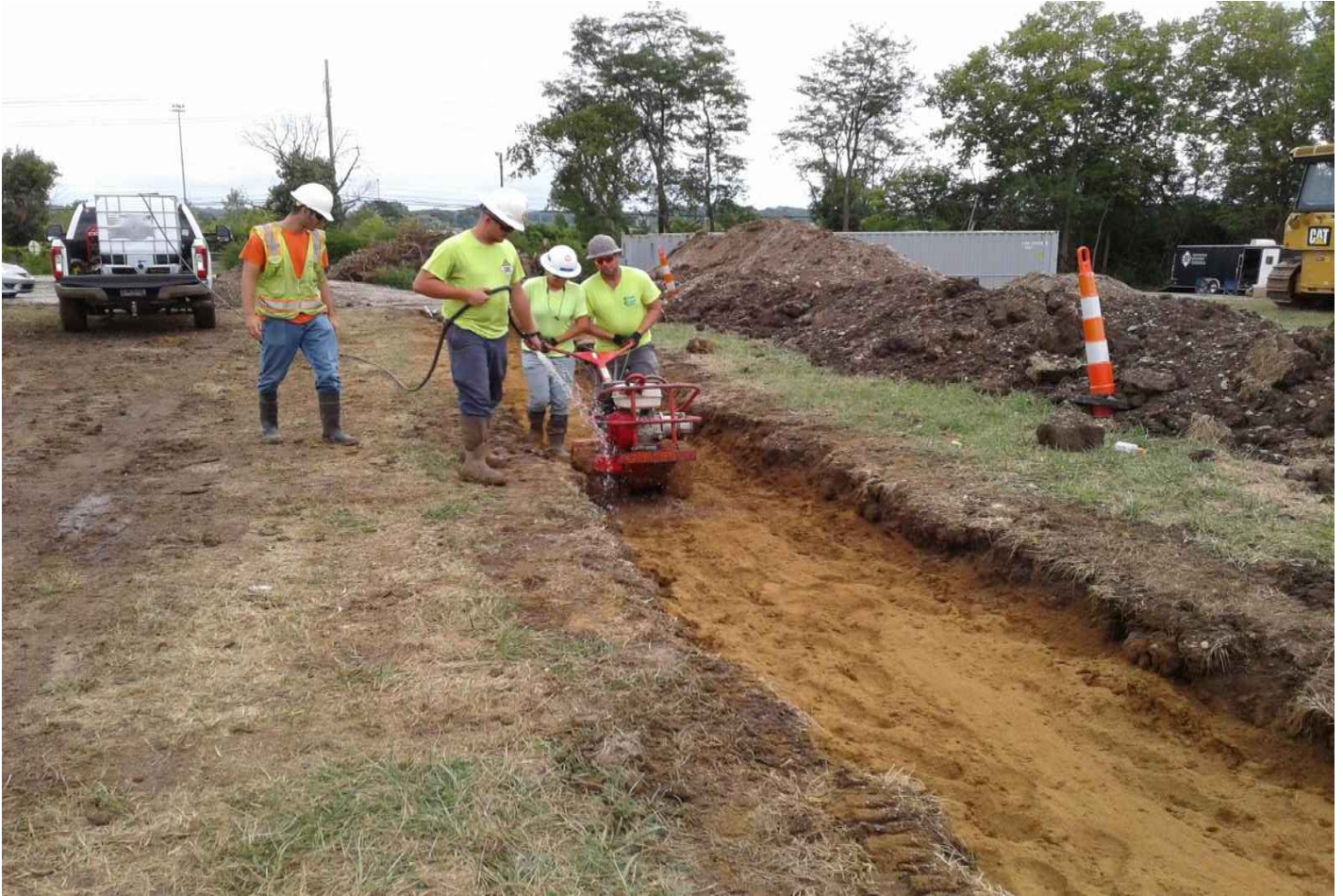
View of compaction site, tilling and watering in progress
