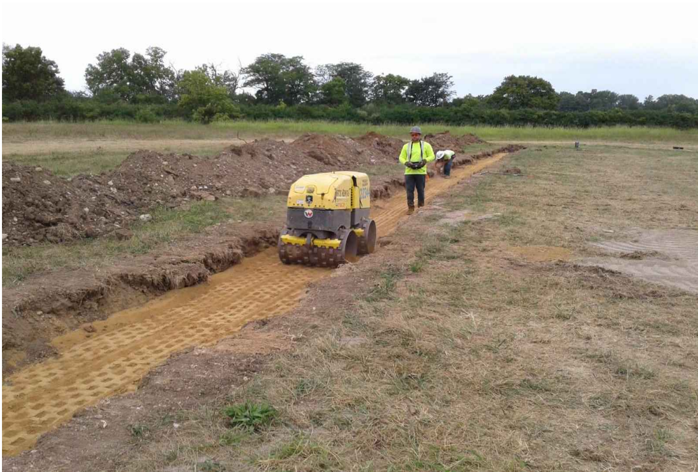
View of compaction site, compaction in progress
