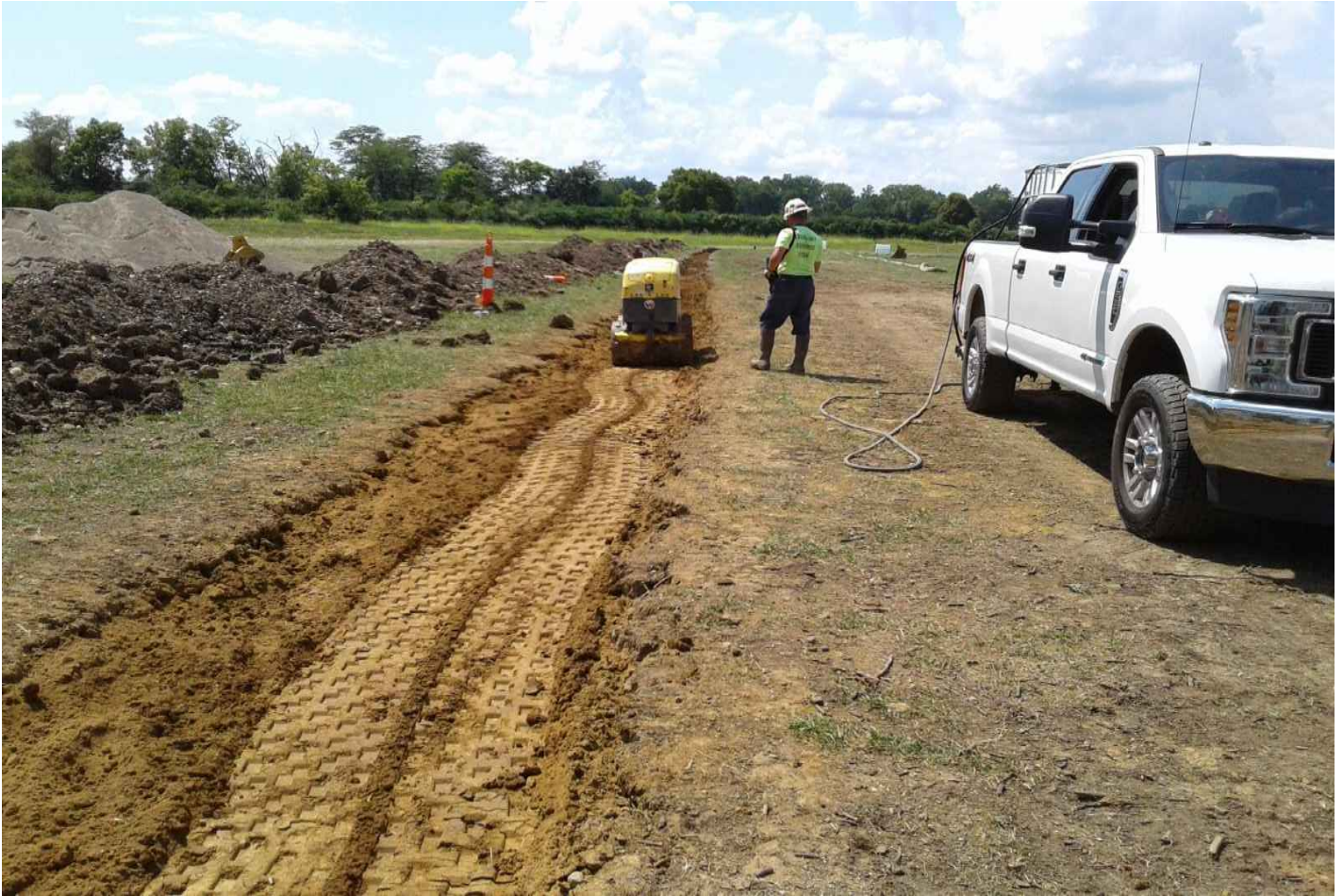
View of compaction site, compaction in progress
