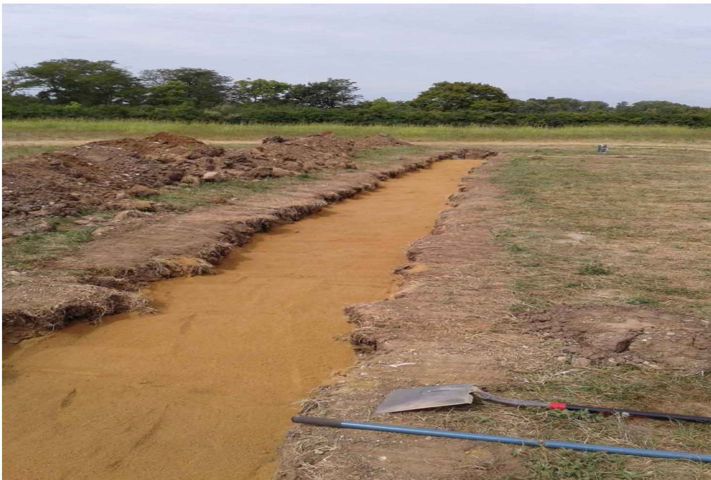
View of clay cap placed within trench, pre compaction
