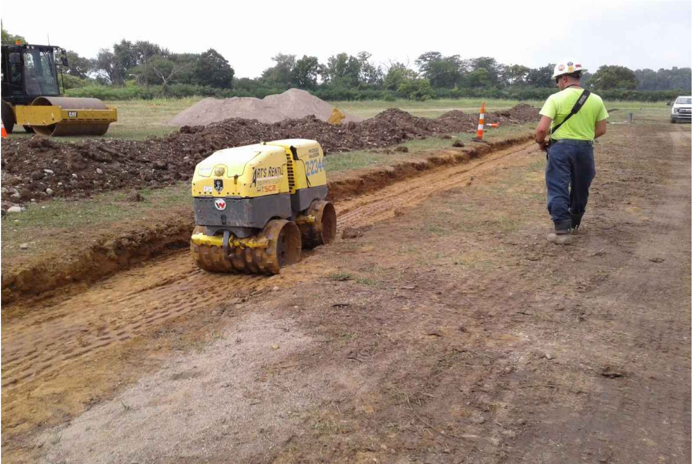
View of compaction site, compaction in progress
