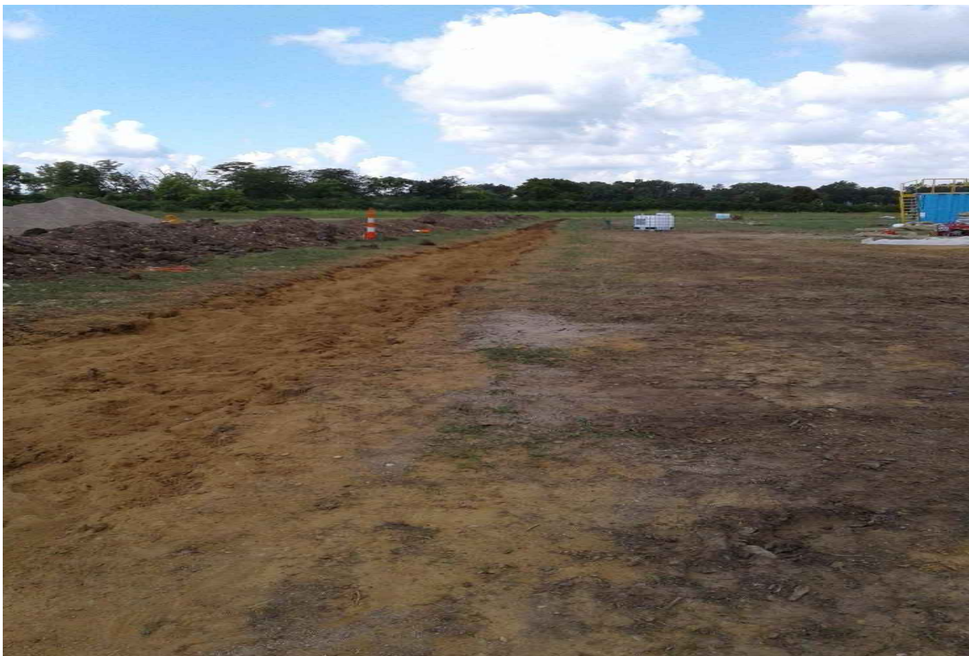
View of compaction site
