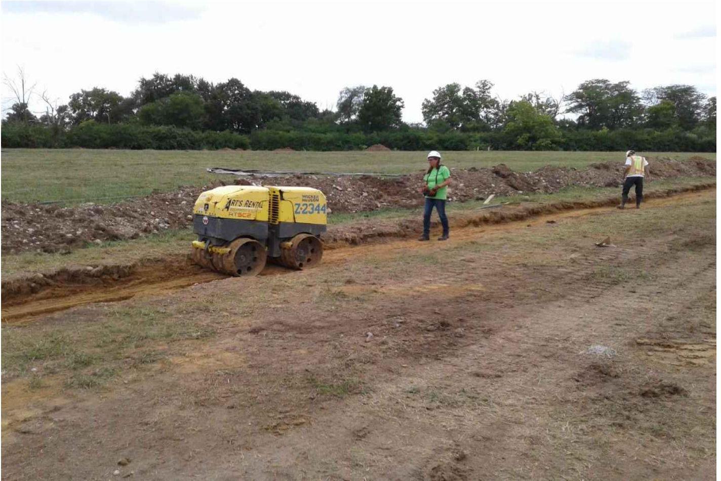
View of compaction site, compaction in progress
