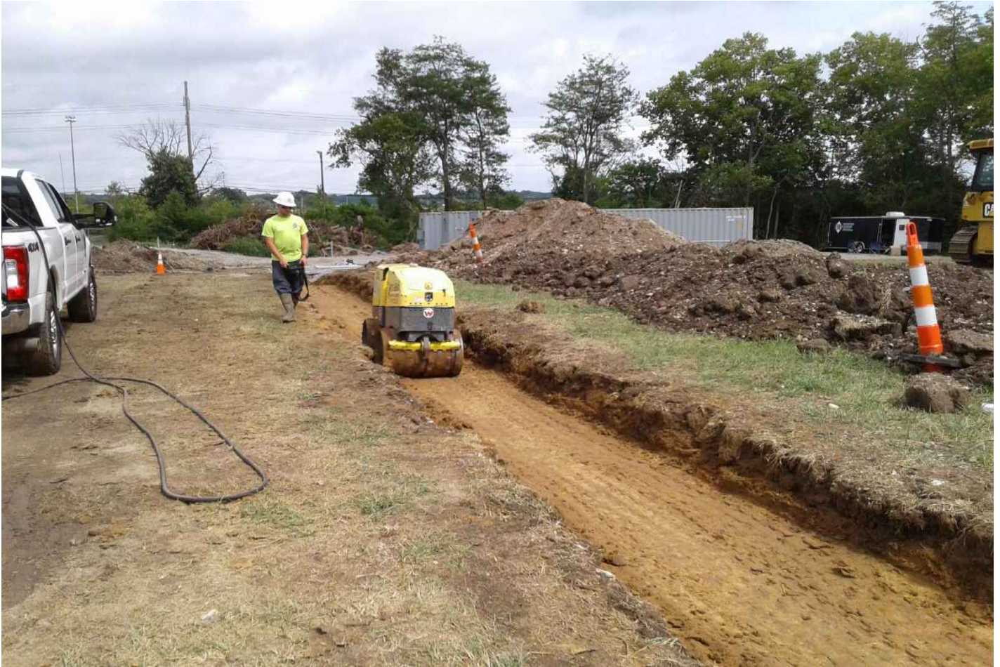
View of compaction site, compaction in progress
