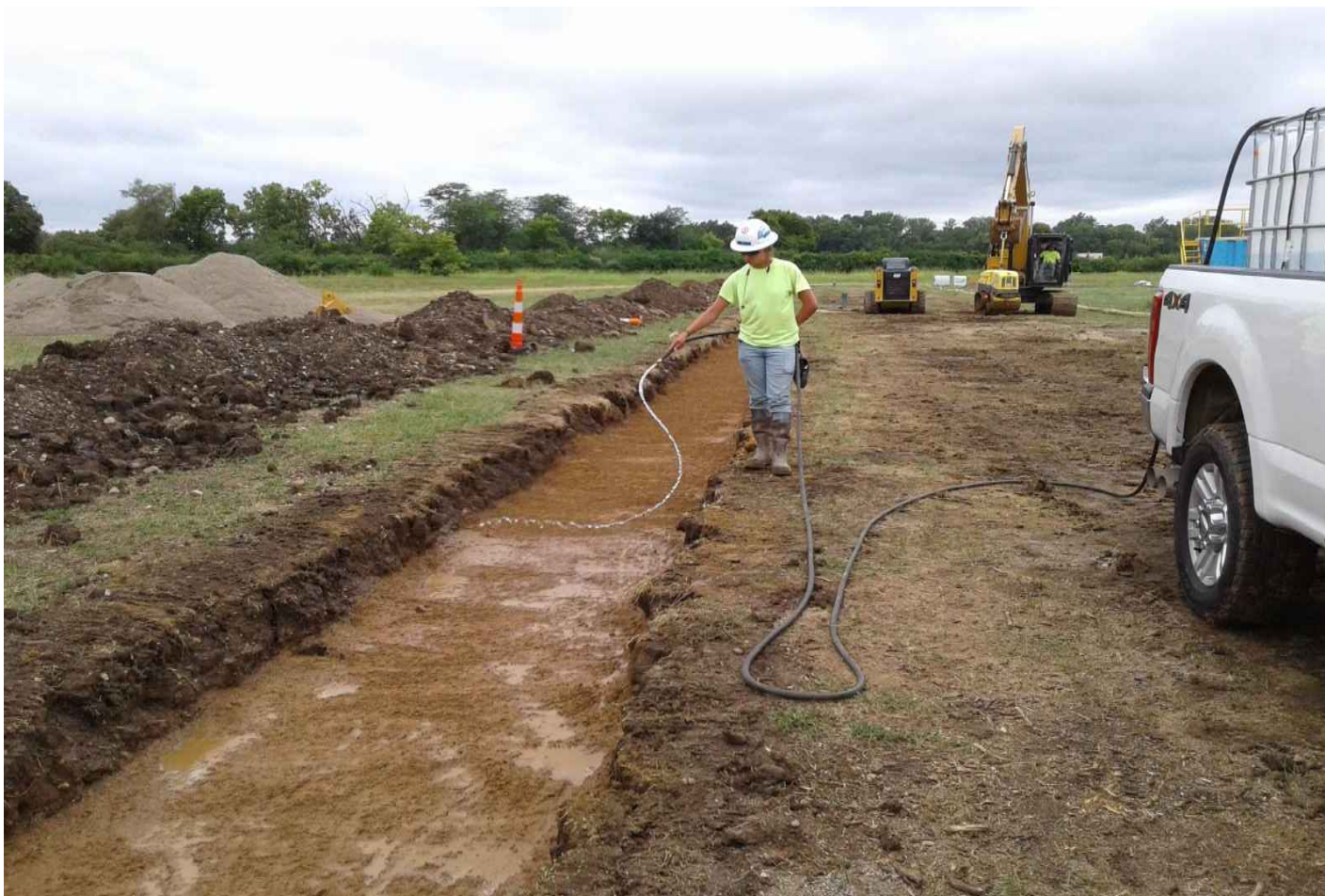
View of compaction site, watering in progress
