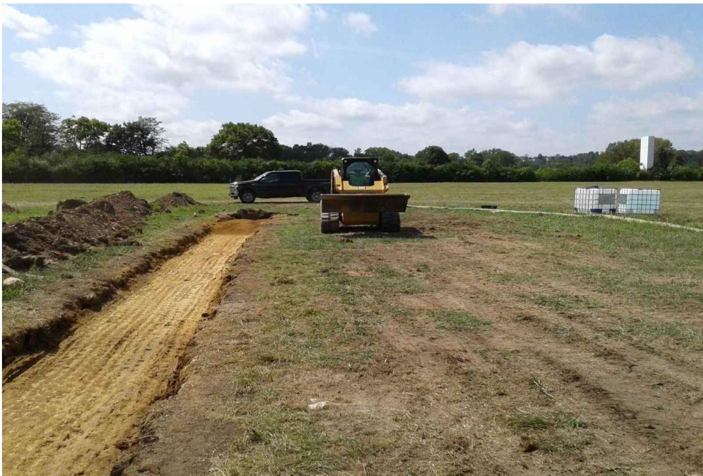
View of compaction site, lift placement in progress
