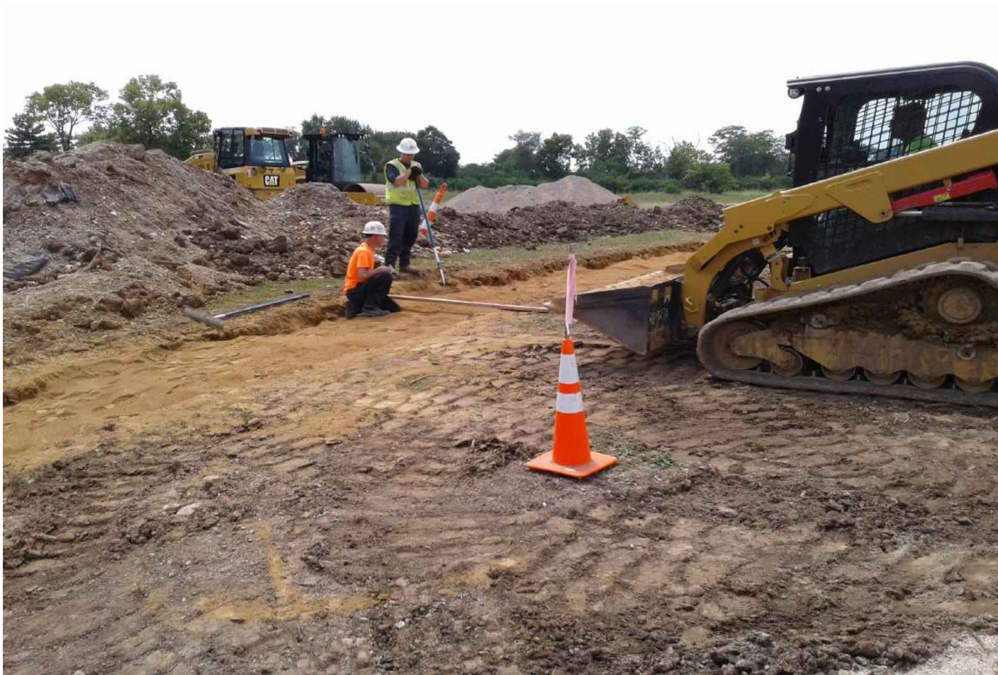
View of compaction site, clay placement in progress
