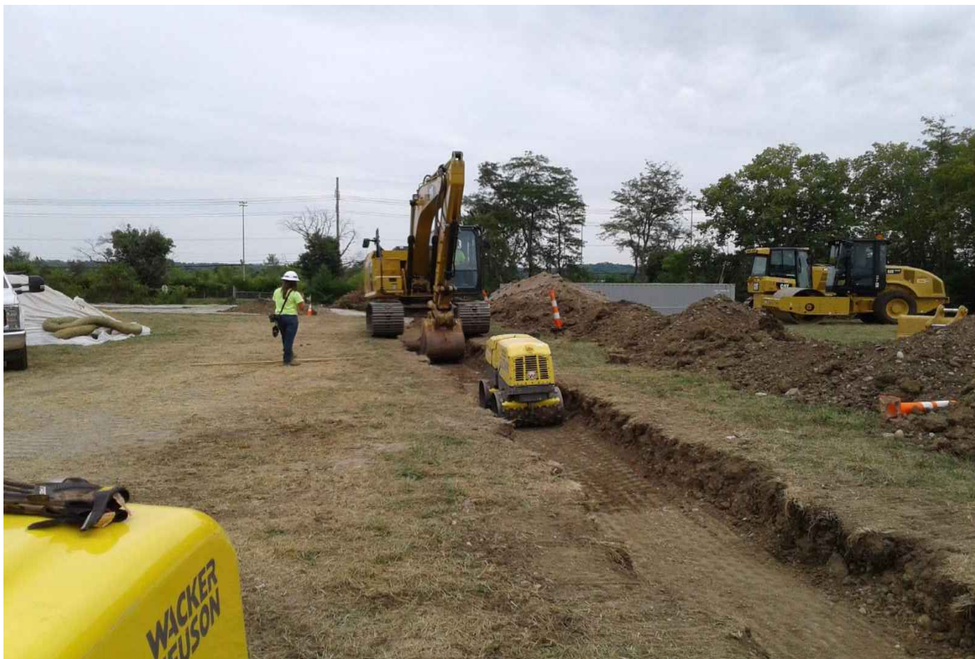
View of compaction site
