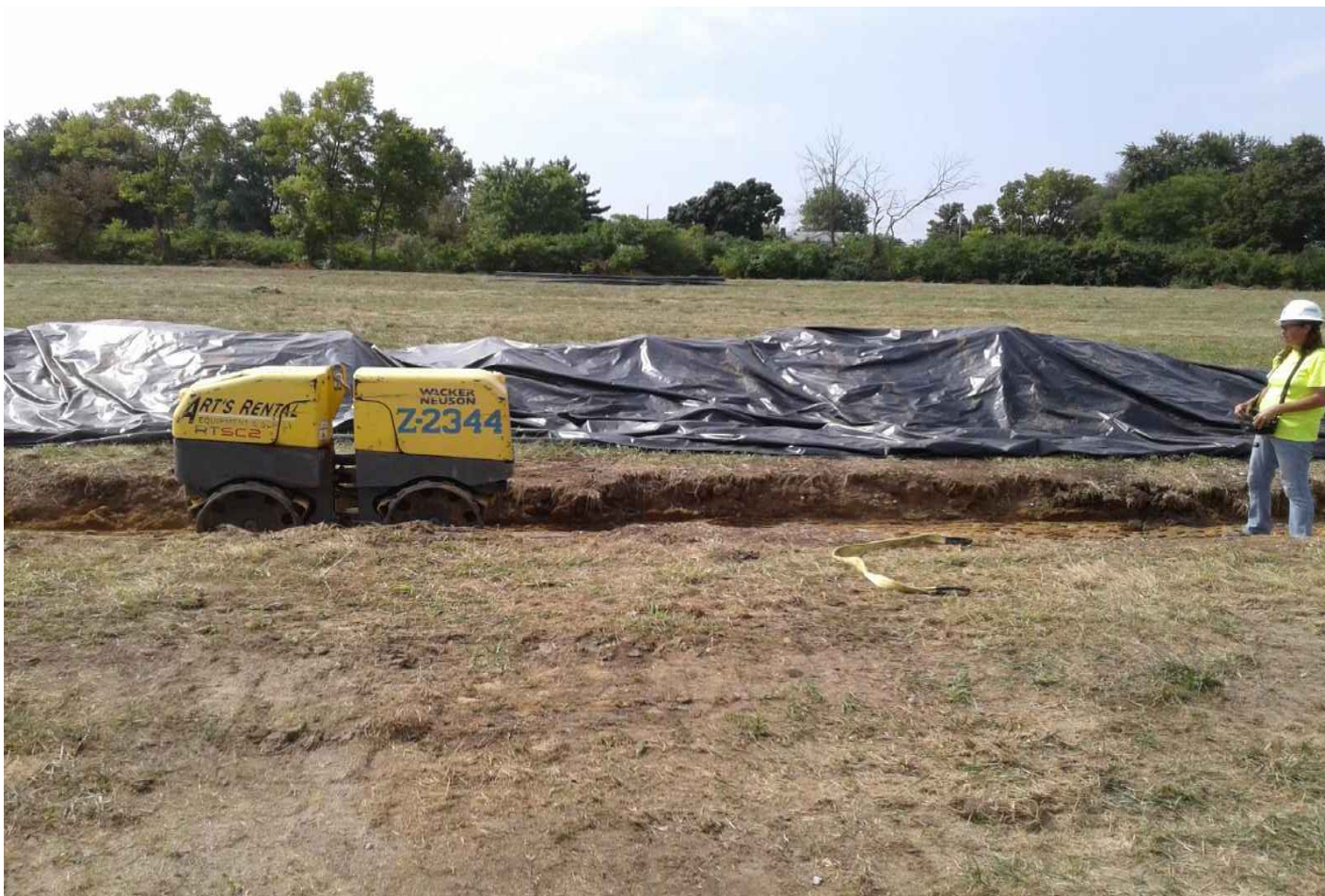
View of compaction site, compaction in progress
