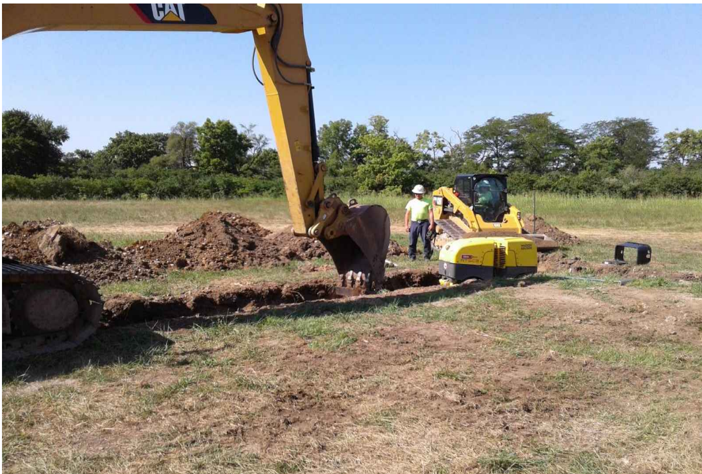
View of compaction site
