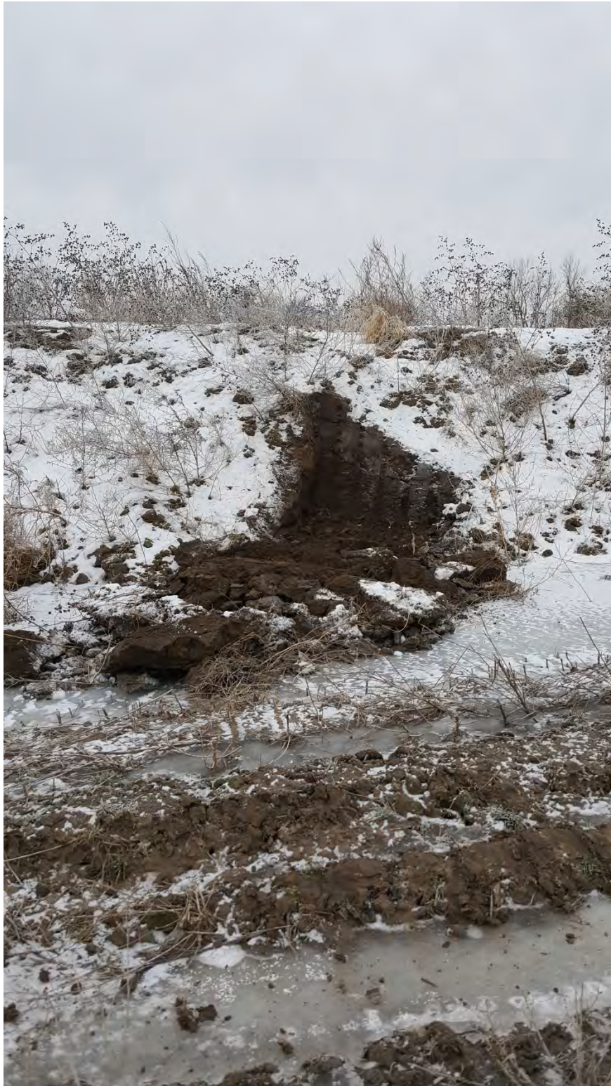
Photo 4 Topsoil Stockpile. Date – 1/16/2016
