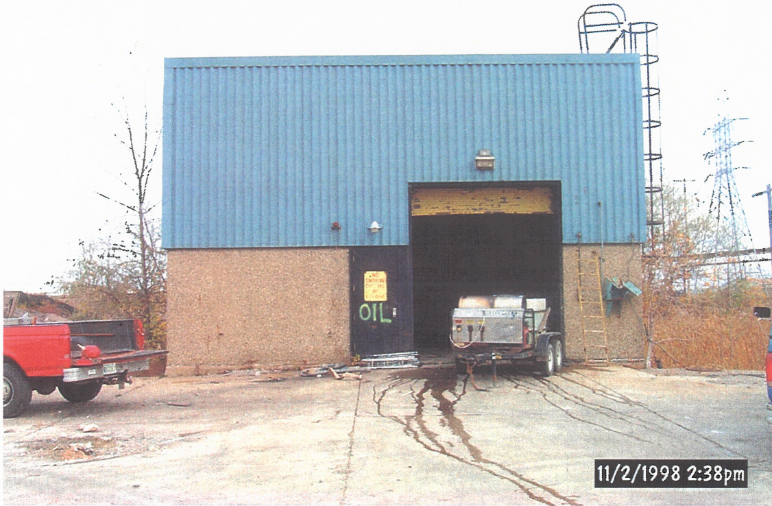
Nodular Iron Oil House, West Entrance (Prior to Cleaning Activities)
