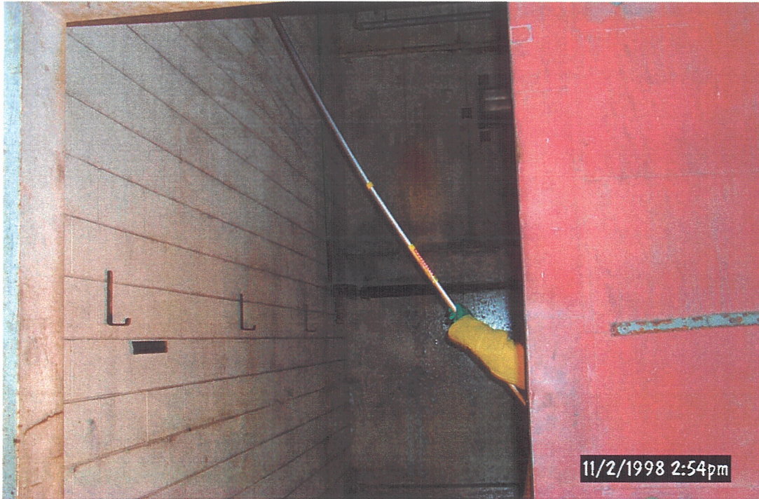
Nodular Iron Oil House, RCRA Storage Unit Wall Scrubbing (Viewing South)
