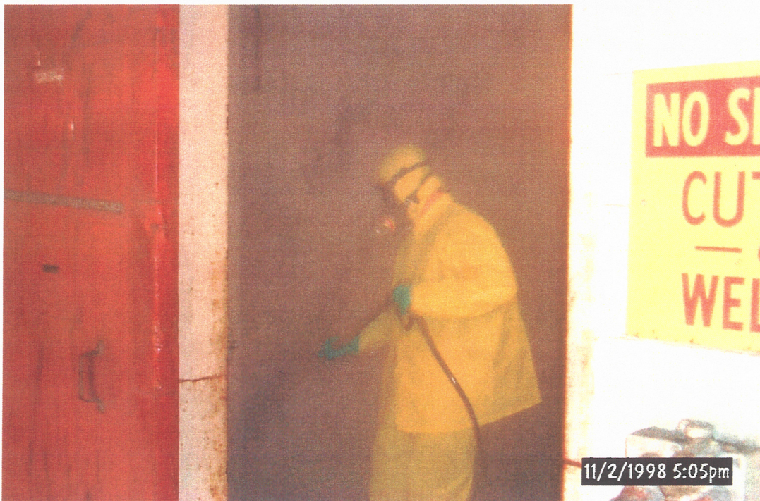
Nodular Iron Oil House, Steam Cleaning RCRA Storage Unit (Viewing Southeast)
