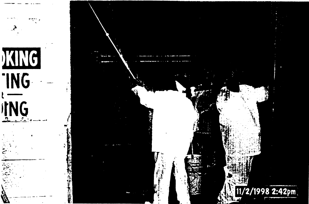
Nodular Iron Oil House, RCRA Storage Unit (Floor and Wall Scrubbing)
