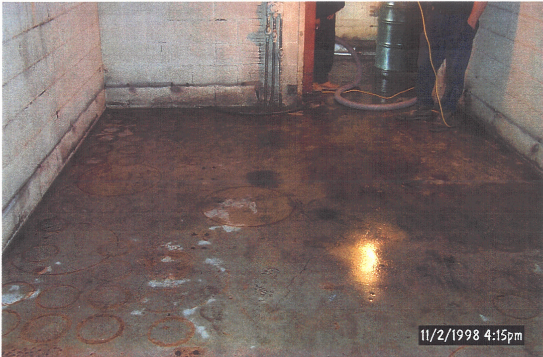
Nodular Iron Oil House, Vacuum Pick-Up of Wash Water After Steam Cleaning Activities (Viewing North)
