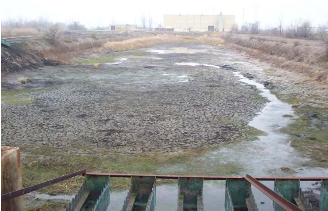
PHOTO 3: PRIMARY SETTLING BASIN 3 - LOOKING SOUTHWEST (12/4/2012)
