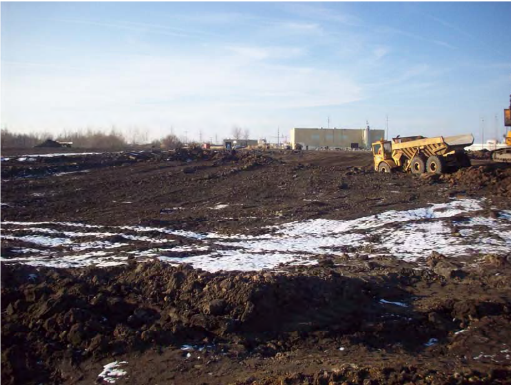
PHOTO 8: PRIMARY SETTLING BASIN 4 - LOOKING SOUTHWEST (01/07/2013)
