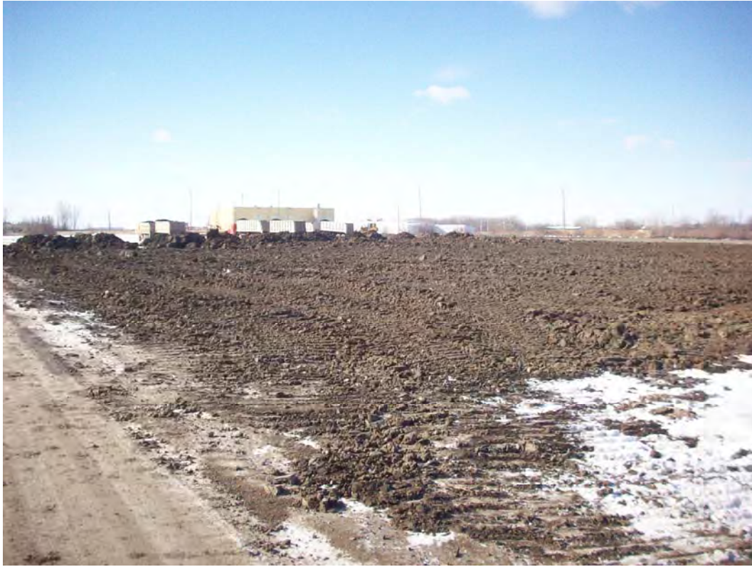
PHOTO 9: PRIMARY SETTLING BASINS - LOOKING SOUTHWEST (02/06/2013)
