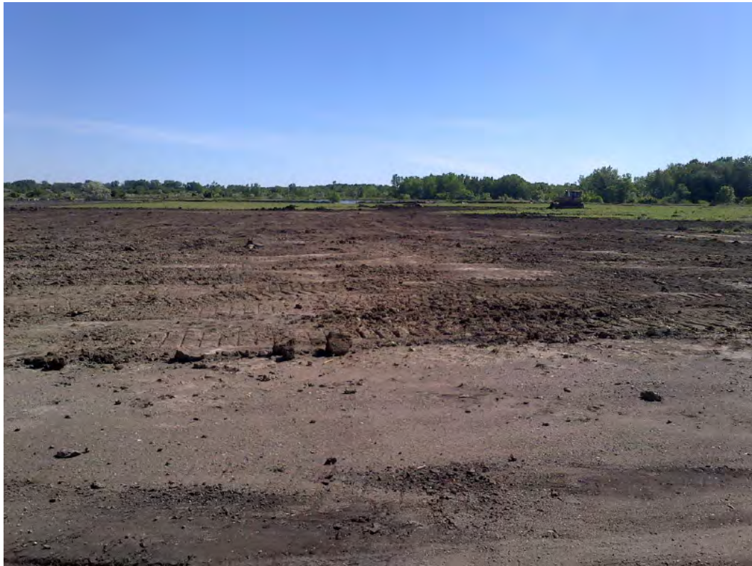
PHOTO 10: PRIMARY SETTLING BASINS – TOPSOIL (06/03/2013)
