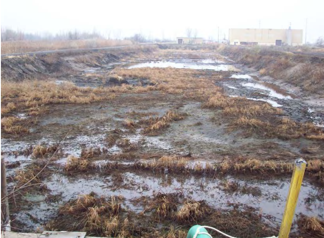
PHOTO 4: PRIMARY SETTLING BASIN 4 - LOOKING SOUTHWEST (12/4/2012)
