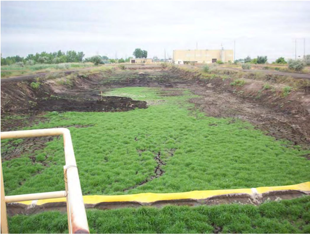
PHOTO 2: PRIMARY SETTLING BASIN 4 - LOOKING SOUTHWEST (07/18/2012)
