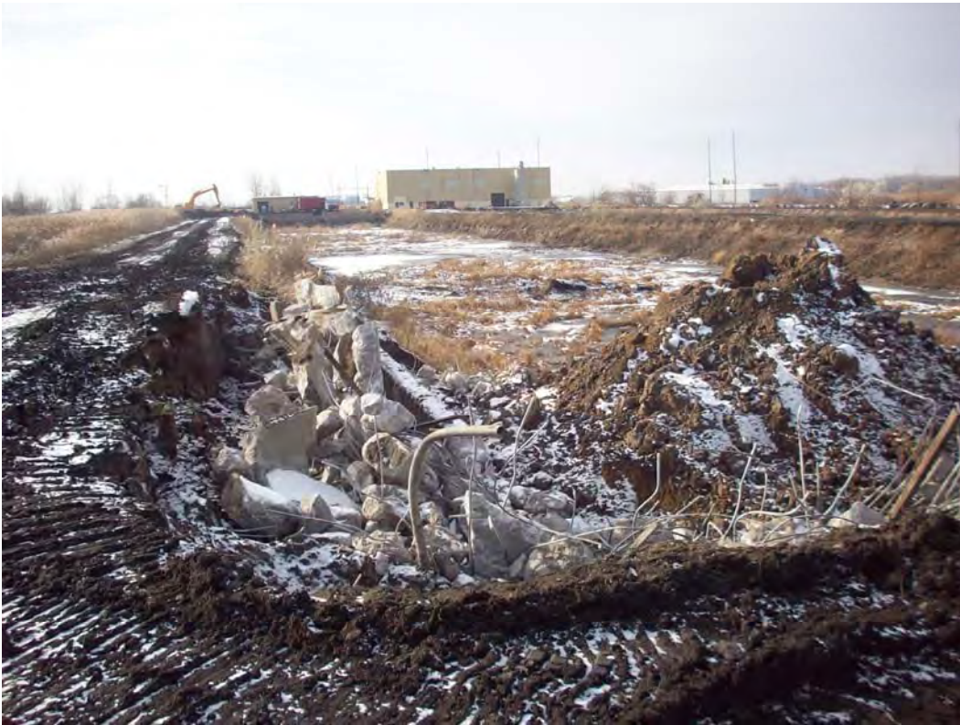
PHOTO 6: PRIMARY SETTLING BASIN 4 - LOOKING SOUTHWEST (12/12/2012)
