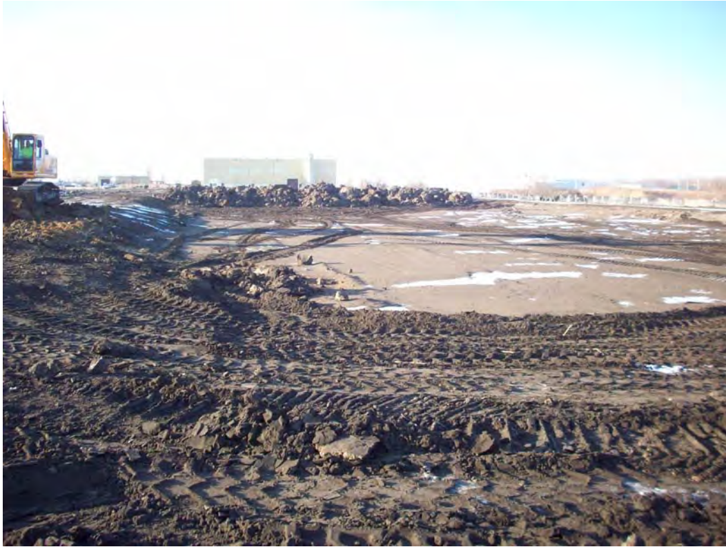
PHOTO 7: PRIMARY SETTLING BASIN 3 - LOOKING SOUTHWEST (01/07/2013)
