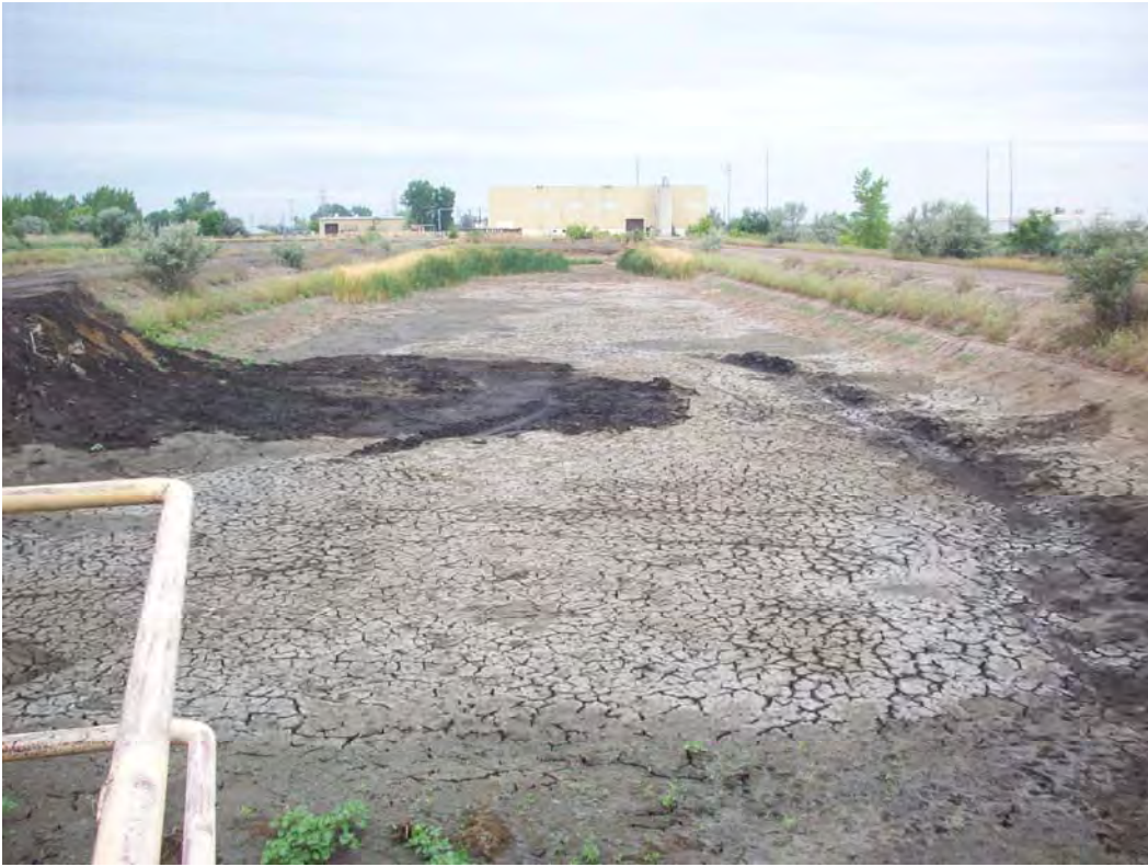
PHOTO 1: PRIMARY SETTLING BASIN 3 - LOOKING SOUTHWEST (7/18/2012)
