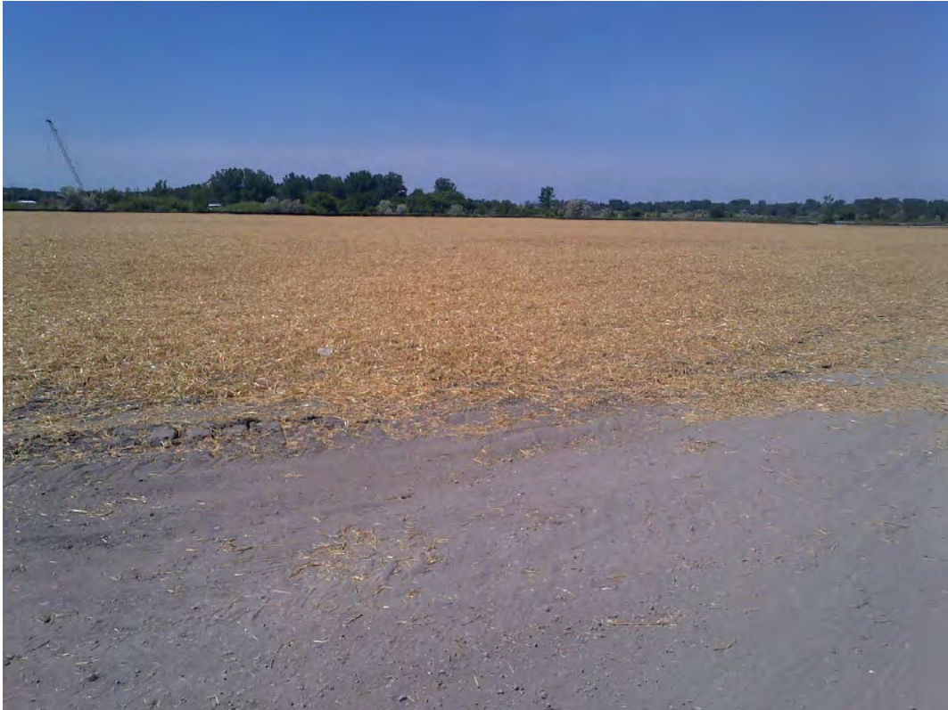
PHOTO 11: PRIMARY SETTLING BASINS - SEEDING (06/20/2013)
