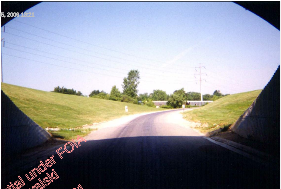
④ LOOKING NORTH AT SWMU #31 (ROAD RUNS UNDERNEATH CENTERPOINT PARKWAY THROUGH SWMU #31)
