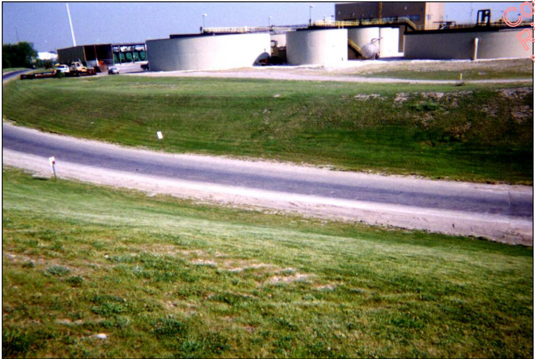
② LOOKING NORTH AT ROAD THROUGH SWMU #31 (WWTP IN BACKGROUND)
