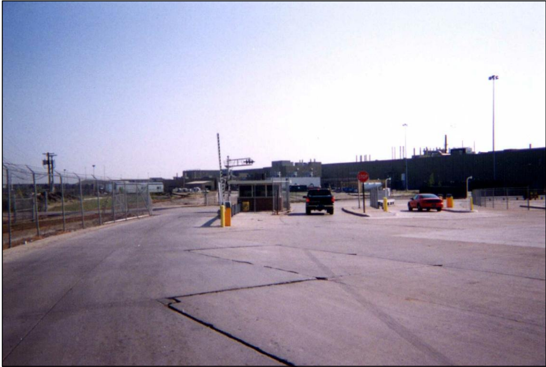
① LOOKING EAST AT GUARD HOUSE RESTRICTING ACCESS THROUGH SWMU #31
