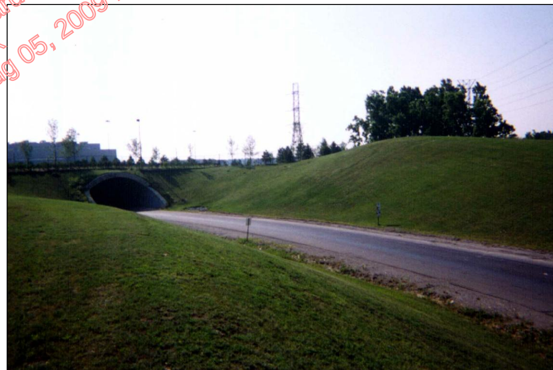
③ STANDING NEAR WWTP LOOKING SOUTHEAST TOWARD SWMU #31 AND TUNNEL UNDER CENTERPOINT PARKWAY (GUARD HOUSE BEYOND TUNNEL NOT SHOWN)
