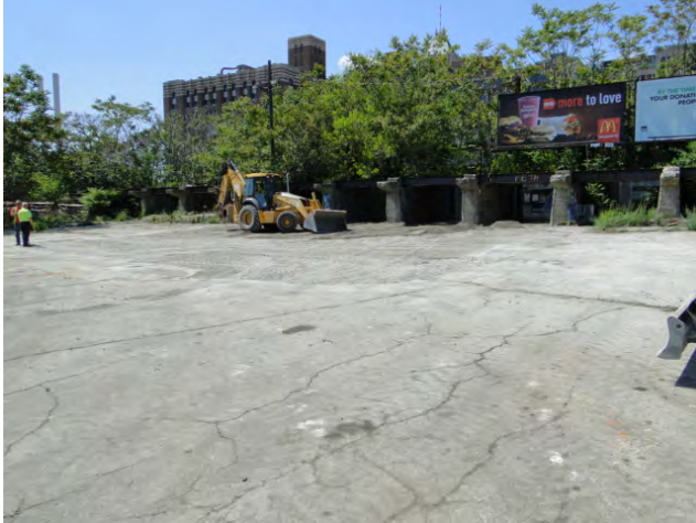
Photo #13: Backfilling in the larger area of excavation approximately 80% complete. Facing northwest.
