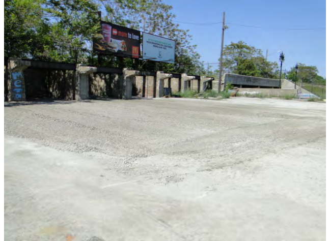
Photo #14: Larger area of excavation backfilled with 21AA aggregate to finish grade. Facing north.
