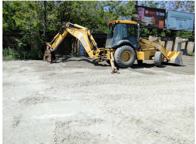
Photo #12: Compacting 21AA aggregate in the larger area of excavation. Facing north.
