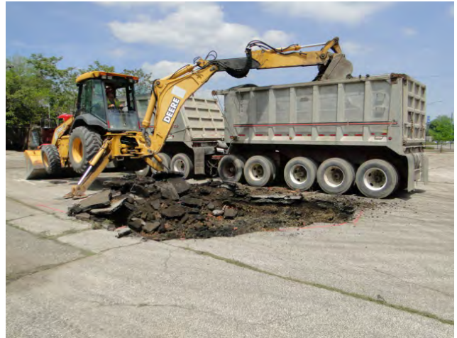
Photo #16: Smaller area of excavation. Removing asphalt and excavating 2 ft. soil cut. Loading into truck for disposal. Facing north.
