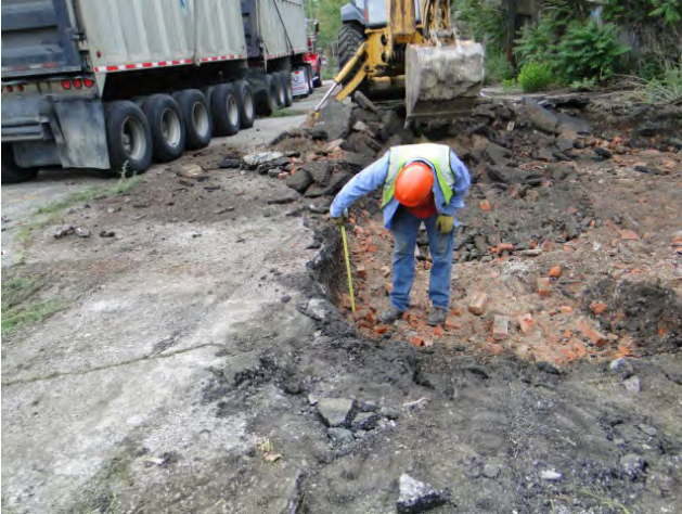
Photo #5: Contractor checking 2 ft. soil cut as work progresses in the larger excavation area. Facing west.
