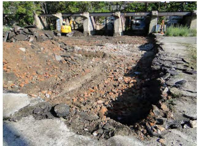
Photo #8: Larger area of excavation. DB-5 boring in foreground, facing northwest towards SB2013-106E. 2 ft. soil cut complete along northeast limits. Survey equipment used for depth verification in background.
