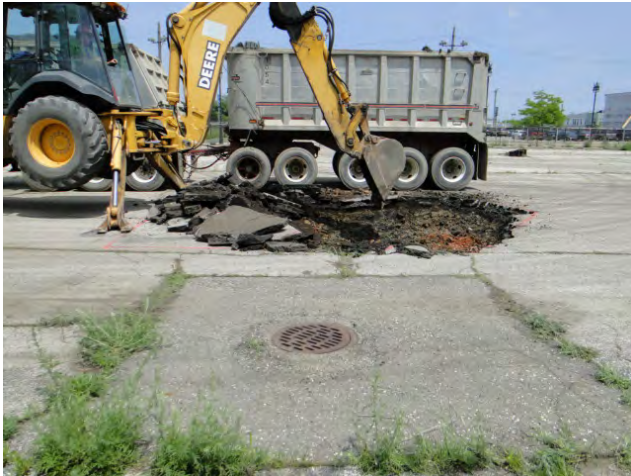
Photo #15: Smaller area of excavation (near DB-3). Removing asphalt and excavating to 2 ft. depth bgs. Loading material into truck for disposal. Facing northeast.
