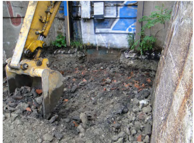
Photo #4: Larger excavation area. Begin 2 ft. soil cut under railroad support structure. Northwest of boring 2013-106E. Facing northwest.
