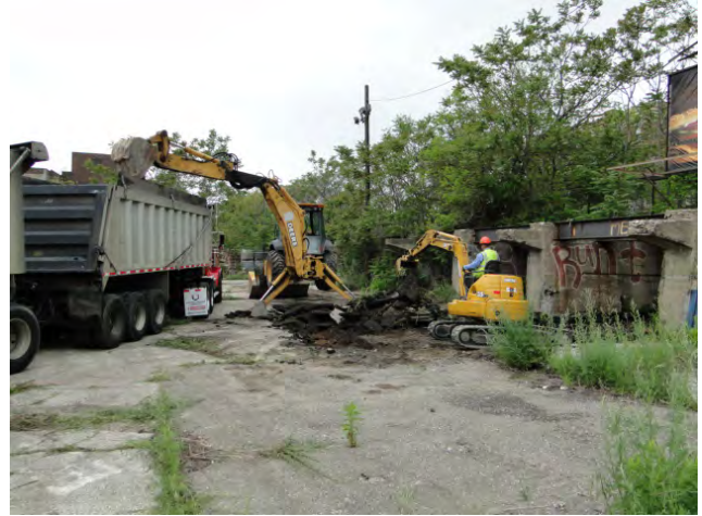
Photo #2: Larger excavation area. Removing asphalt from the 2013-106E boring area, working north and west. Loading into truck for disposal. Facing west.
