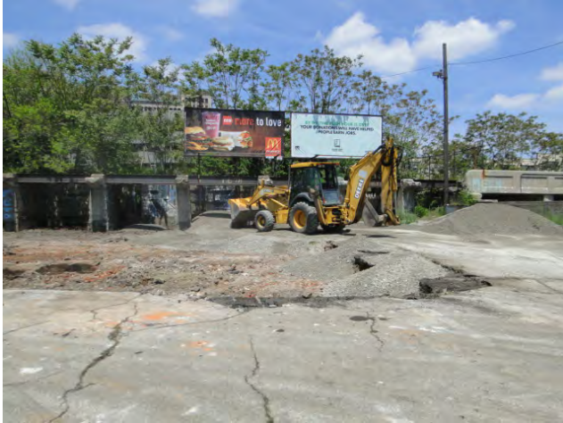
Photo #9: Larger area of excavation. 2 ft. soil cut complete. Beginning backfill with 21AA aggregate. Facing north.
