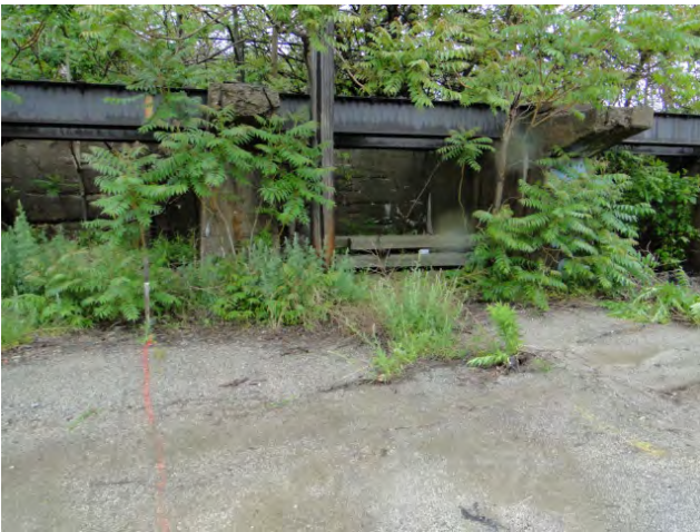
Photo #7: Larger area of excavation. SB2013-107 survey stake in background. Pre-excavation outline (orange) in foreground. Facing north.
