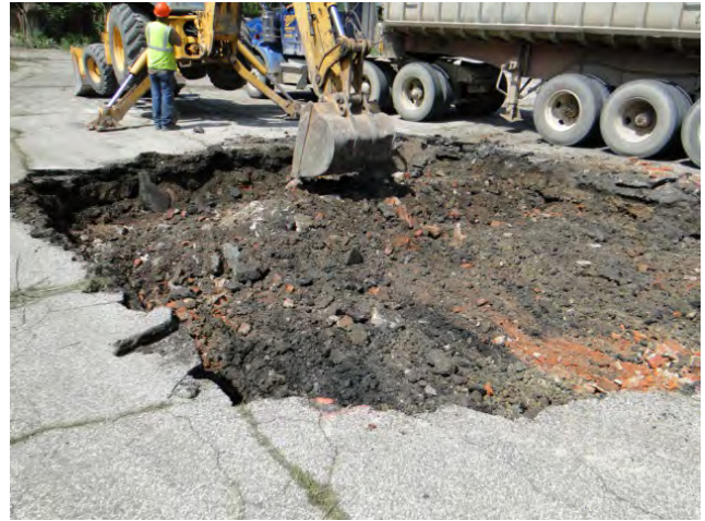
Photo #18: 2 ft. soil cut approximately 90% complete in the smaller area of excavation. Facing northwest.
