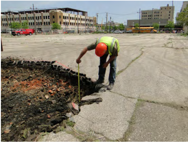
Photo #17: Contractor checking 2 ft. soil cut as work progresses in the smaller area of excavation. Facing southeast.
