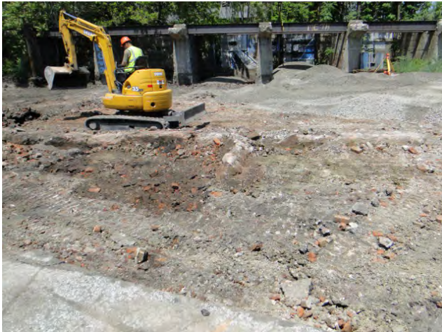
Photo #11: Larger area of excavation. Grading excavation area prior to backfilling. Facing northwest.
