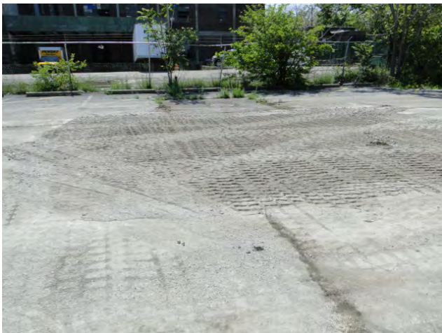
Photo #19: The smaller area of excavation backfilled with 21AA aggregate to finish grade. Facing east.
