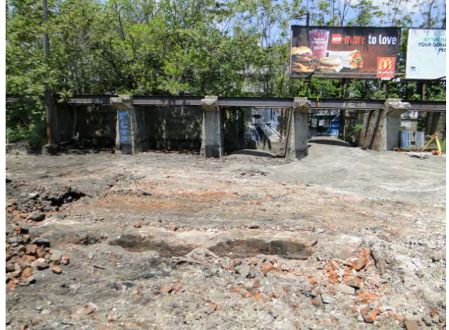
Photo #10: Larger area of excavation. Concrete footer exposed during soil removal. Footer left in place and is below finish grade. Facing northwest.
