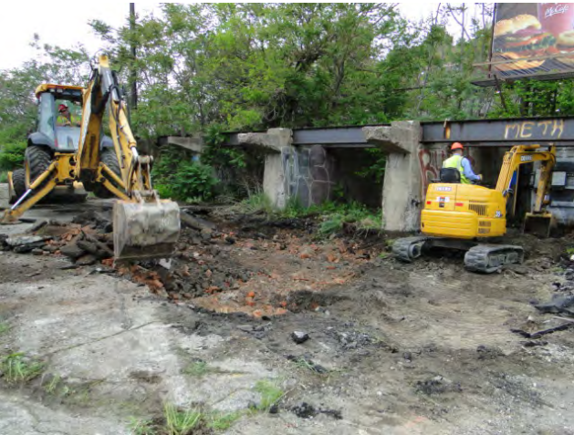
Photo #3: Larger excavation area. Removing asphalt from the 2013-106E boring area. Facing west.
